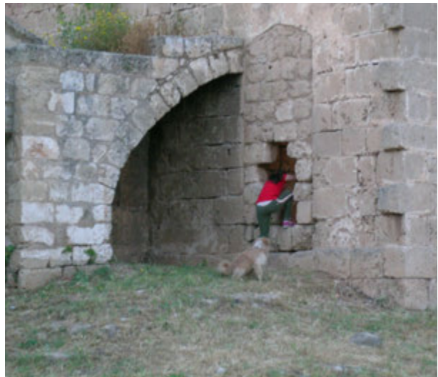
FIGURE 134. A walled opening has been partially reopened, and now offers a way to enter the interior of the church.
