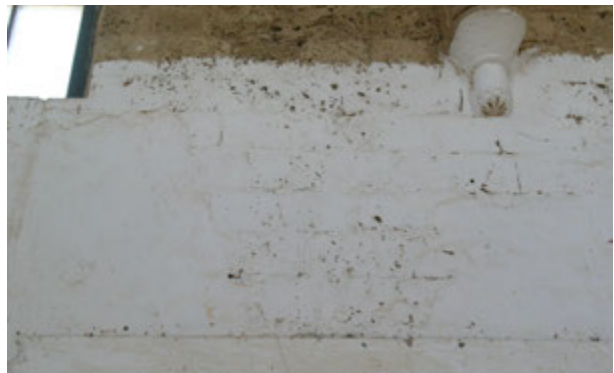
FIGURE 156. Differences in surface levels and texture indicate that painting fragments might still exist underneath.
