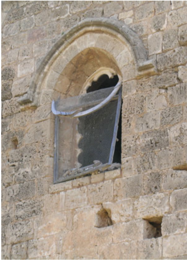
FIGURE 104. Broken wire mesh on the western window of the Armenian Church.
