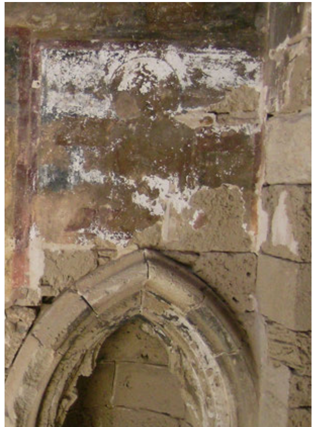
FIGURE 103. The outside painting on the tympanum of the west portal is almost completely lost
