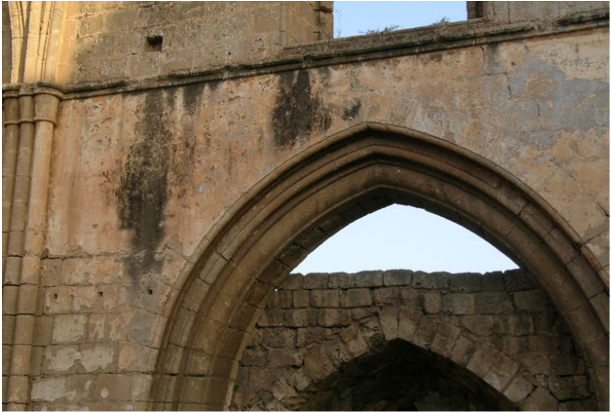
FIGURE 129. Dark stains from the growth of algae can be seen on the south wall of the nave.
