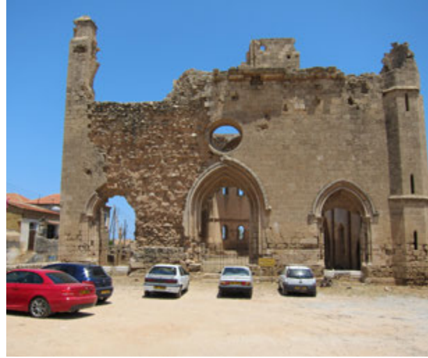
FIGURE 40. The parking lot in front of the Church of St. George of the Greeks could be reimagined as a playground with new landscaping.
