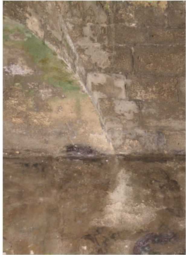
FIGURE 105. Active water infiltration is indicated by a stain of green algae and salt efflorescence on the painting below.
