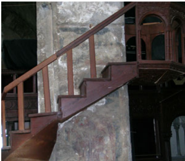
FIGURE 146. A large area of painted plaster was removed from the northern pillar to install the staircase of the pulpit.
