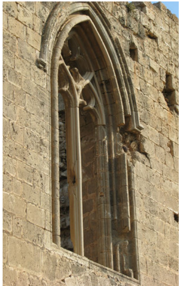
FIGURE 64. The erosion of previous restorations at the Church of St. George of the Greeks.
