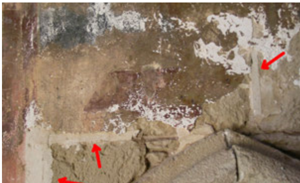
FIGURE 100. Fragments of the stucco finish can also be seen in areas where the painting has been lost.
