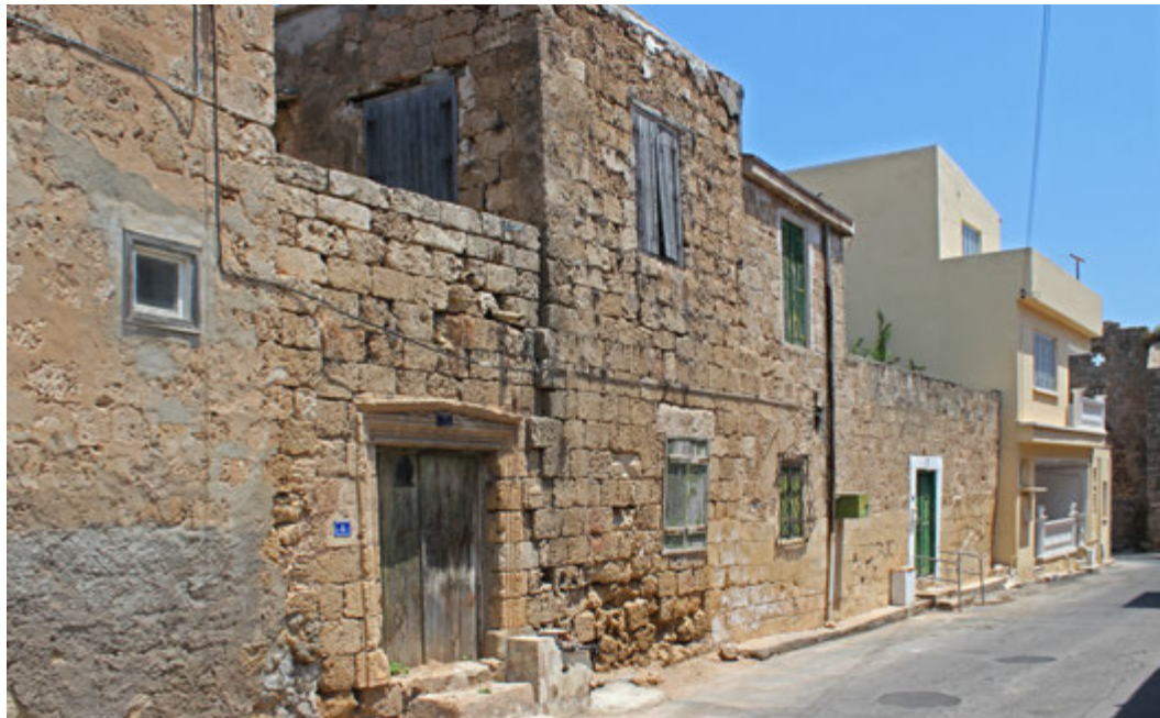
FIGURE 7. Typical streetscape in the Walled City, characterized by low-rise buildings along the street wall, with little or no space between party walls.
