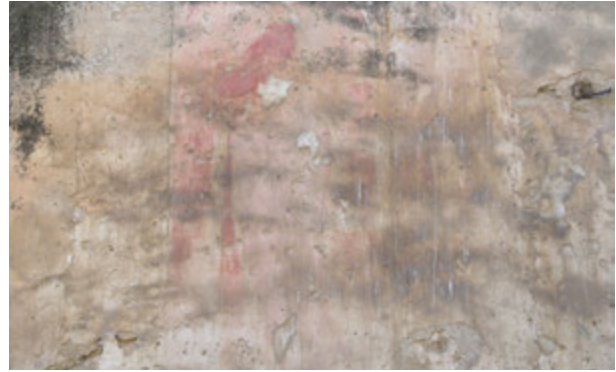
FIGURE 86. This highly deteriorated fragment on the south wall of the church is another later painting (Layer E).
