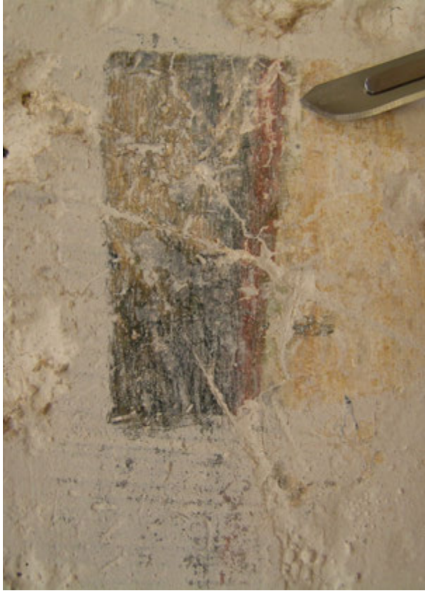
FIGURE 108. The lime layer that has been applied over earlier painted plaster can be easily removed.
