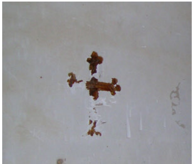
FIGURE 147. Crosses made with a wax-based material have been applied in many locations at the church.
