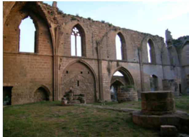
FIGURE 122. The lower sections of the south wall preserve fragments of plaster with traces of painting in all five bays.
