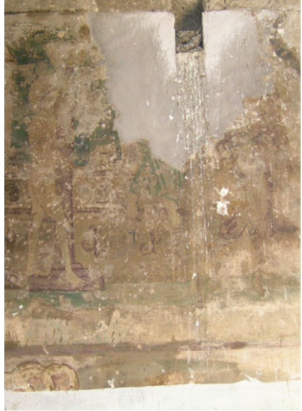
FIGURE 109. Bird nest and guano deposits can be seen inside the Armenian Church.”).
