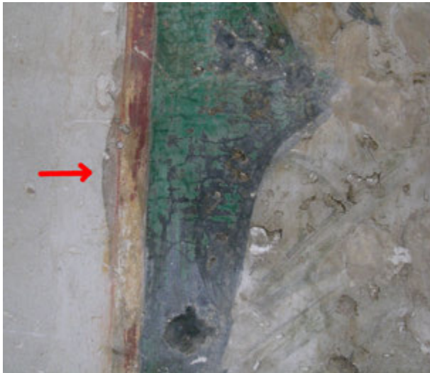
FIGURE 144. The blackening of the wax coating is visible in areas where its application extended onto the white plaster.
