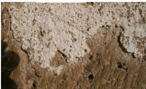
FIGURE 119. The painting plaster in the southern side apse is composed of two thin layers without fibrous material.
