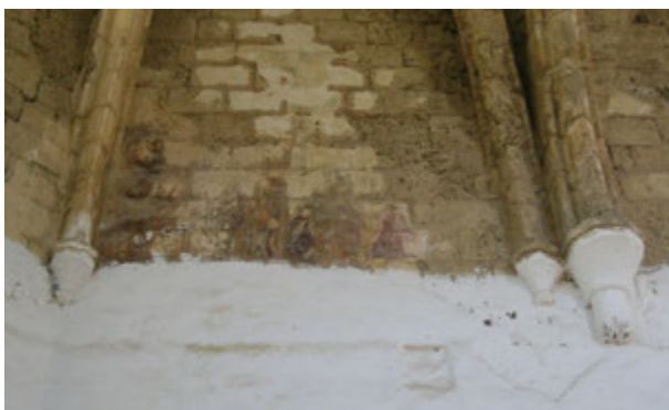
FIGURE 157. Fragments of white plaster with ashlar decoration and remains of a complex composition painted directly on top.
