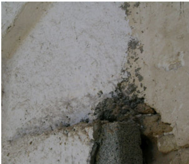
FIGURES 163, 164. These details on the south wall (left) and the north wall (right) show the application of cement slurry onto the walls. As the right image shows, the cement slurry is in contact with the painted surface and lies underneath the cement plaster.
