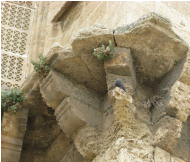
FIGURE 53. Eroded brackets on the apse of St. Nicholas Cathedral (Lala Mustafa Pasha Mosque).
