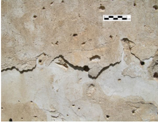
FIGURE 90. The detachment of plaster at the Carmelite Church of St. Mary.
