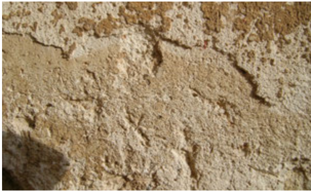
FIGURE 115. The plaster in the central apse is composed of a rough plaster containing straw and a thin layer of fine plaster.
