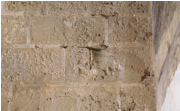
FIGURE 99. The stucco finish of the stone masonry can be seen clearly on the west wall.
