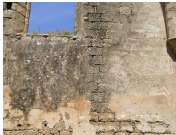
FIGURE 93. Dark patina from the growth of algae on the north wall of the Carmelite Church of St. Mary.
