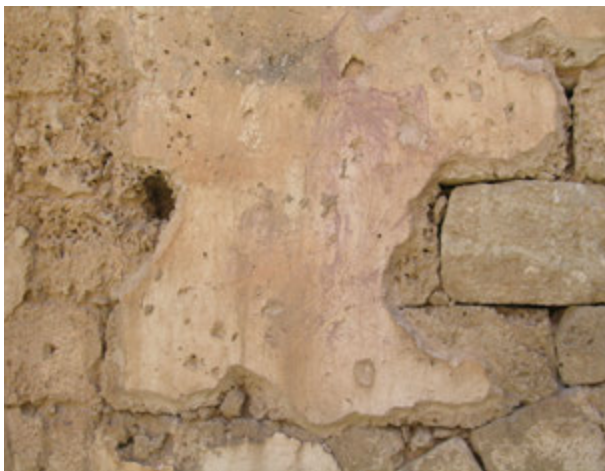
FIGURE 92. Erosion due to rainwater percolating over the south wall of the Carmelite Church of St. Mary.
