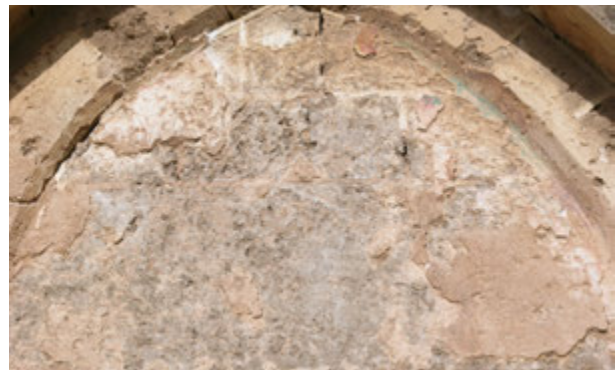
FIGURE 101. Stucco finish and remains of painted plaster on the tympanum of the west portal of the Armenian Church.
