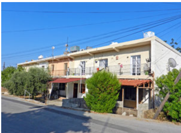
FIGURE 14. Social housing was constructed in the late twentieth century in the northern edge of the Walled City.
