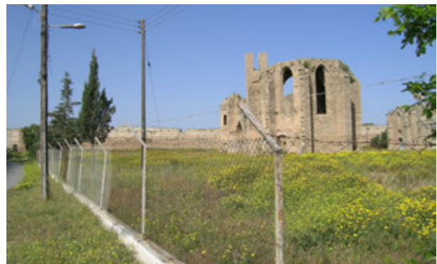
FIGURE 89. View of the Carmelite Church of St. Mary from the East, with the fence that surrounds the site.
