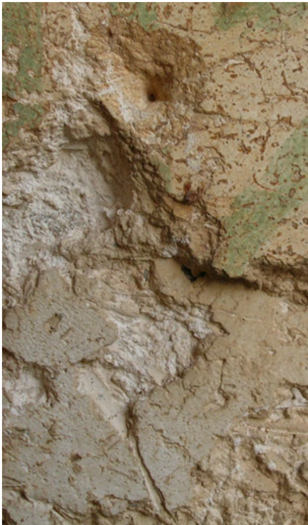
FIGURE 121. The painting plaster in the northern side apse contains straw and fine fibers.
