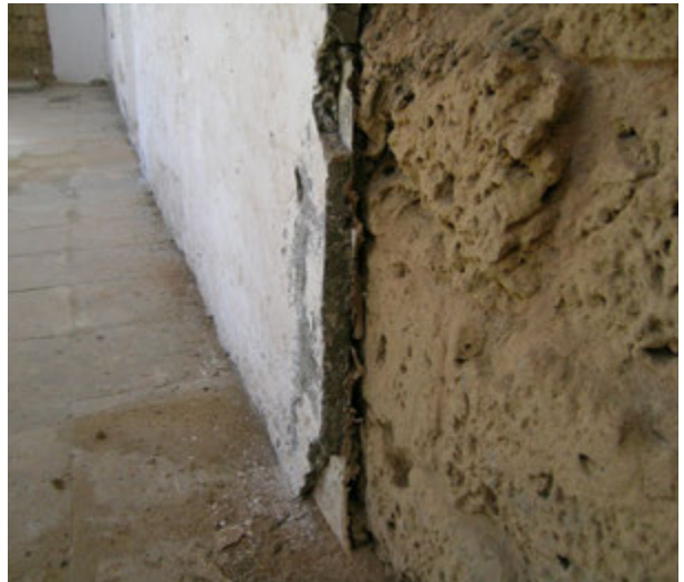
FIGURE 162. Fiberboard between the original wall surface and the cement plaster near the bottom of the south wall.
