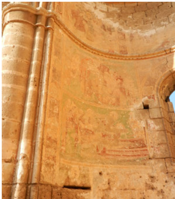
FIGURE 60. Well-preserved fragments of painted plaster can be seen in the apse on the south side of the Church of St. George of the Greeks.
