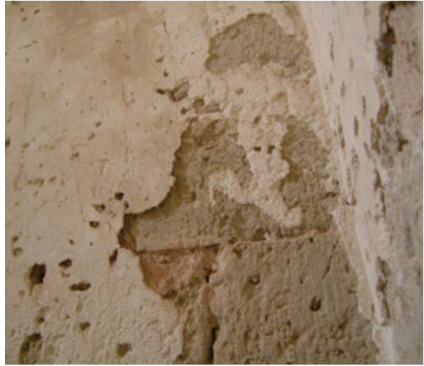
FIGURE 143. Severe detachment of plaster in the northwest corner of the nave.
