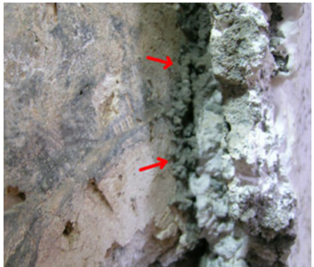
FIGURES 163, 164. These details on the south wall (left) and the north wall (right) show the application of cement slurry onto the walls. As the right image shows, the cement slurry is in contact with the painted surface and lies underneath the cement plaster.
