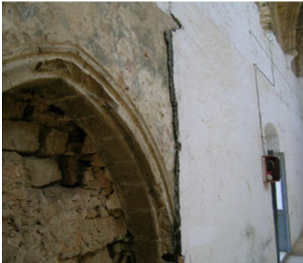
FIGURE 161. Cement plaster covers most of the lower register of the painting scheme, as seen here along the north wall.
