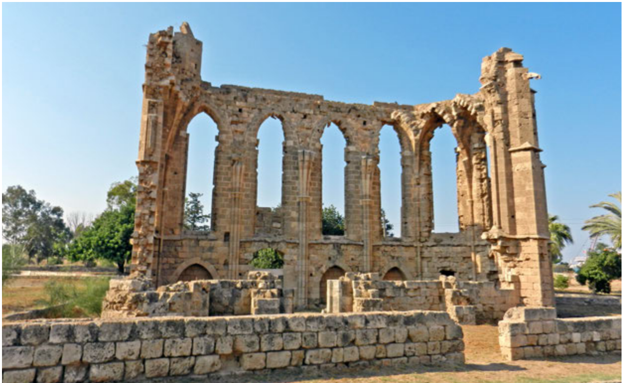
FIGURE 13. The ruins of the Church of St. George of the Latins are located to the north.
