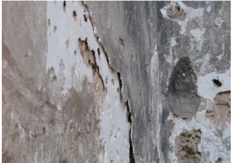
FIGURE 63. Potential plaster loss in the Church of St. Anne.
