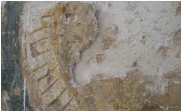
FIGURE 155. A detail of one of the later paintings in the northwest corner, which use the white plaster as a ground.
