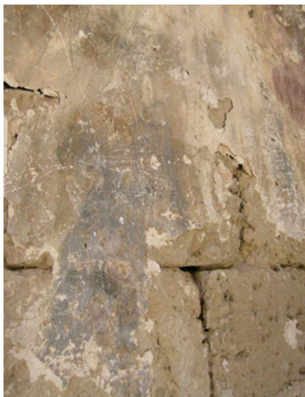
FIGURE 107. Severe detachment of plaster from its support can be seen in the lower part of the north wall.
