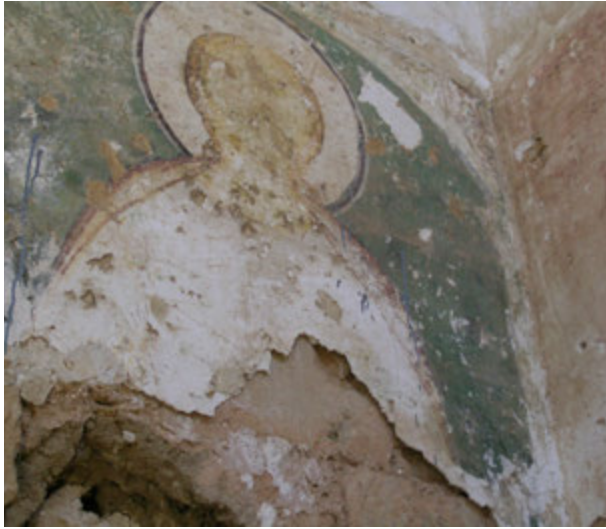
FIGURE 159. Severe bulging of the plaster and separation between the two layers on the south wall.
