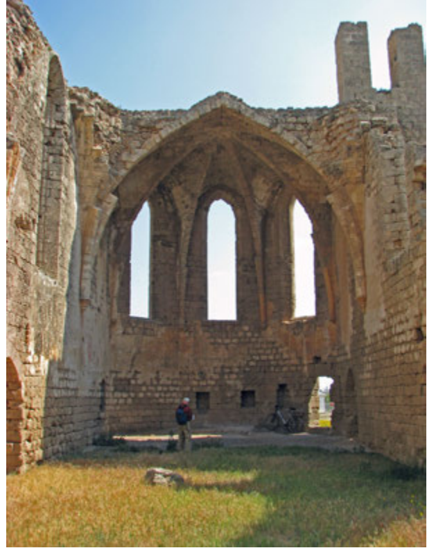
FIGURE 66. This vault above the apse of the Carmelite Church of St. Mary may become compromised if the structure is allowed to deteriorate further.
