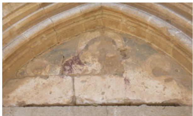
FIGURE 158. A painting of the Virgin and Child can be seen in the tympanum above the main portal on the western façade.
