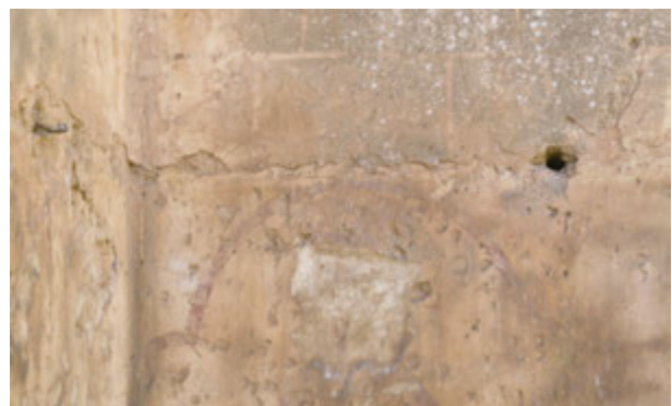
FIGURE 76. An earlier painting scheme is visible underneath the ashlar decoration on the west wall.
