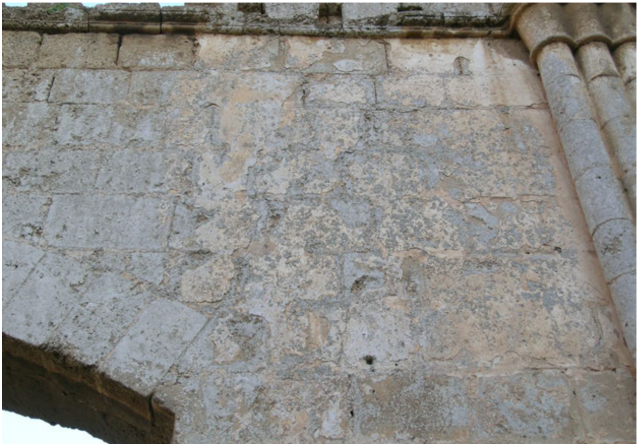
FIGURE 130. A light gray patina of lichens covers most of the south wall of the nave.
