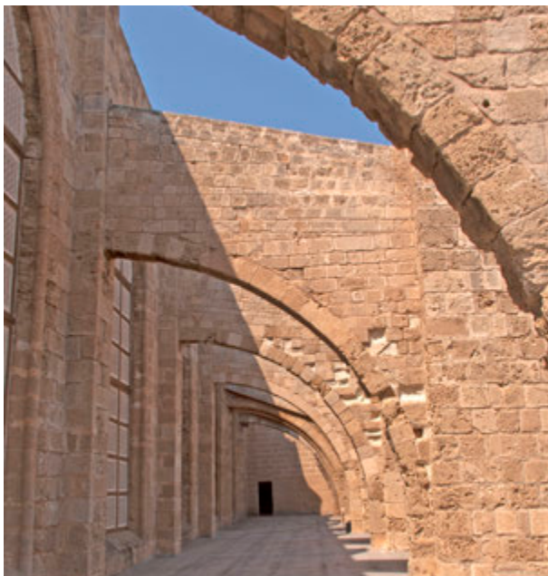
FIGURE 47. The roof and buttresses of the well-preserved St. Nicholas Cathedral (Lala Mustafa Pasha Mosque).
