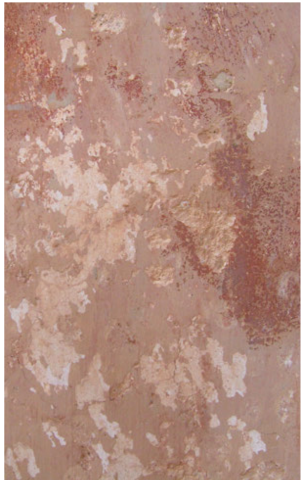
FIGURE 95. The wax coating that was applied over the wall paintings in the 1930s has become opaque.
