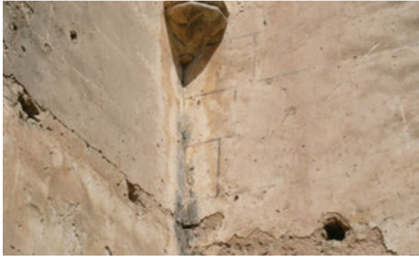
FIGURE 69. Dark gray lines on white plaster in the northwest corner of the church suggest a pattern of mortar joints.
