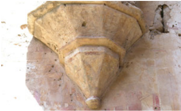
FIGURE 71. Console with painted decoration on the north wall of the Carmelite Church of St. Mary.
