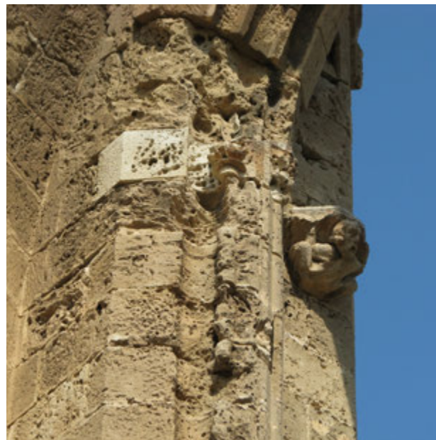
FIGURE 44. Wind and water erosion.
