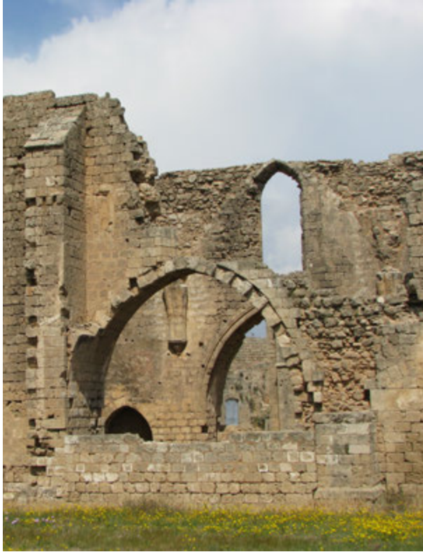
FIGURE 65. This arch on the south façade of the Carmelite Church of St. Mary is asymmetrically loaded and at risk of collapse.
