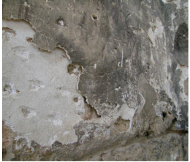
FIGURE 160. On the west wall, the painting plaster is lifting off from the plaster underneath.
