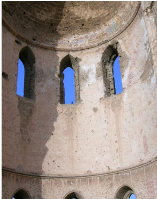
FIGURE 111. The central apse of the Church of St. George of the Greeks is almost completely covered with whitish plaster.
