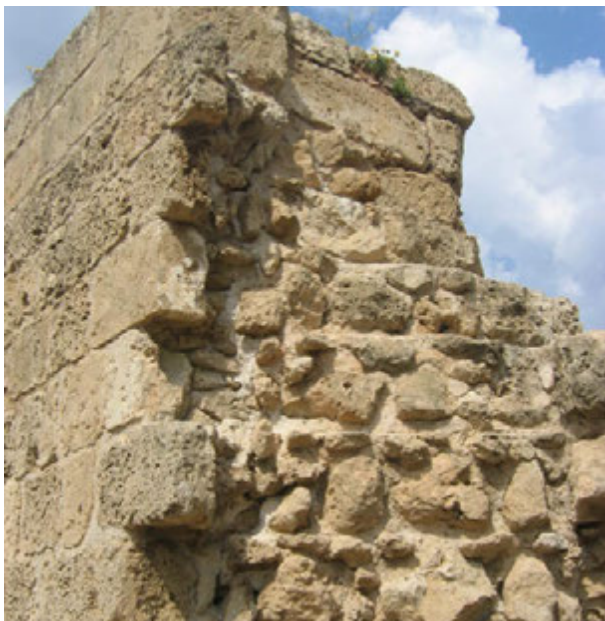
FIGURE 43. Ashlar dimension stone, filled with a core of mortared rubble.
