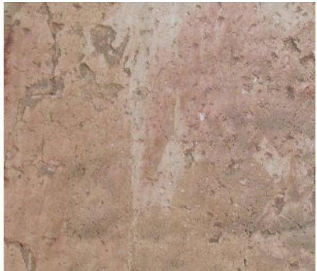
FIGURE 126. Heavily eroded painting fragment on the north wall, near the northwest corner of the church.
