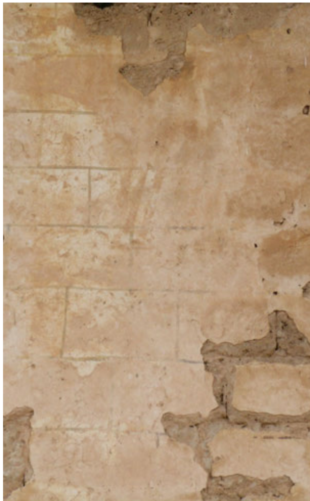
FIGURE 94. Brownish dust deposit covers the ashlar decoration of the plaster in the apse of the Church.
