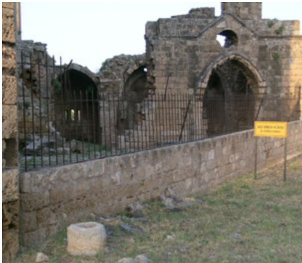
FIGURE 133. The fence protecting the site toward the southwest.
