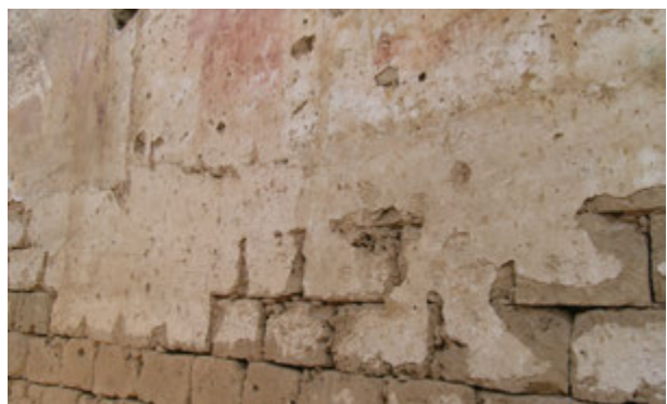
FIGURE 84. An unpainted plaster layer covers the lower part of the wall, and earlier painted layers.
