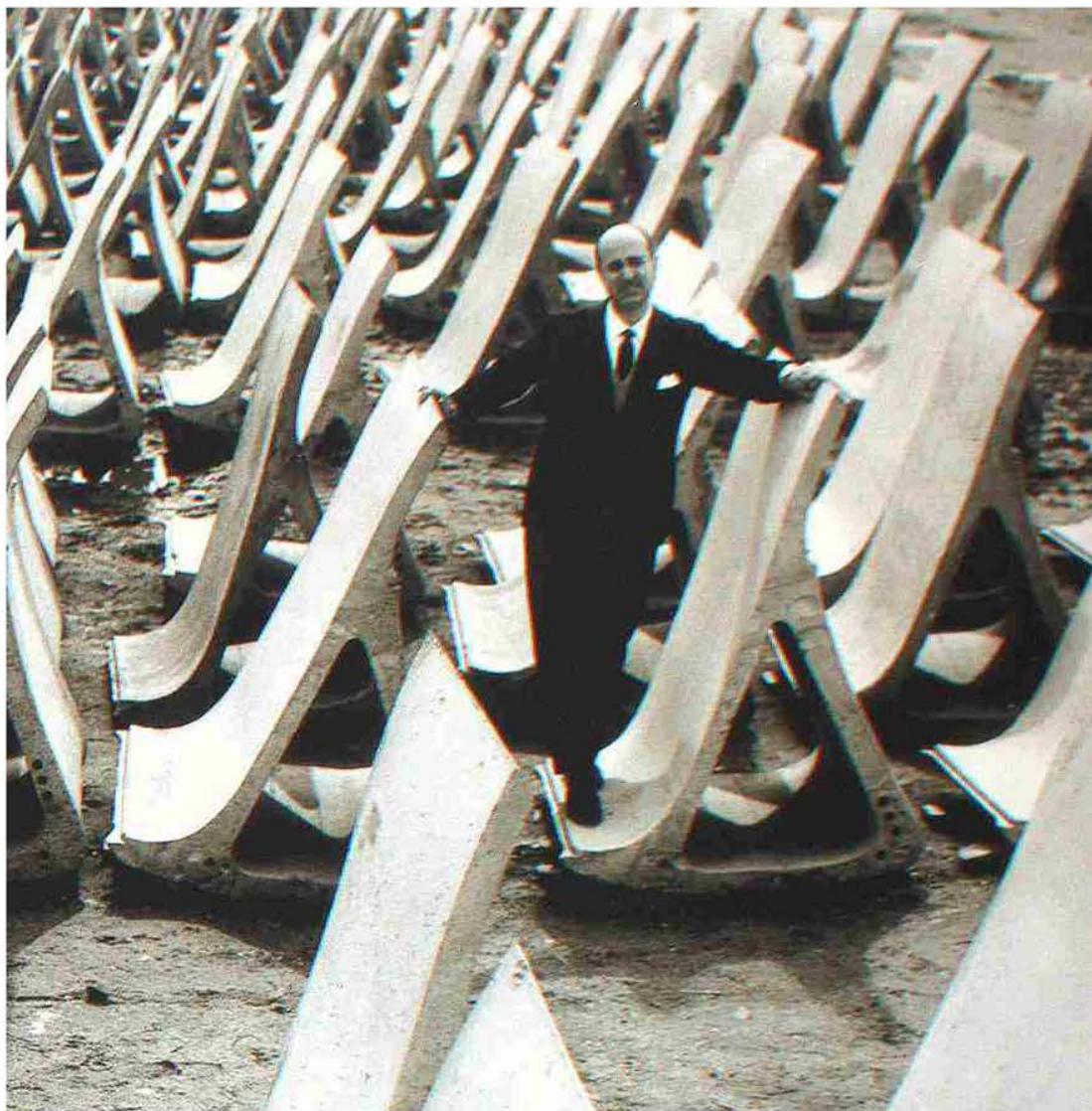
MIGUEL FISAC SURROUNDED BY PRE-FABRICATED VOUSOIRS, 1962
