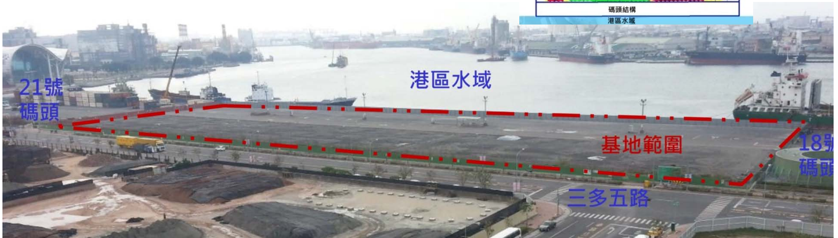
Kaohsiung Port Terminal Site Remediation
