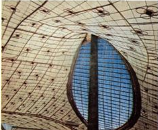
Massive cables stretch taut the skin of West Germany's big top
