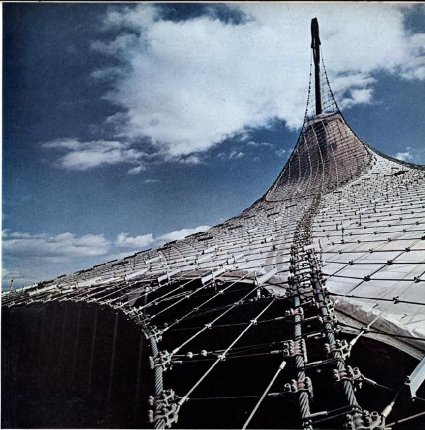
Massive cables stretch taut the skin of West Germany's big top
