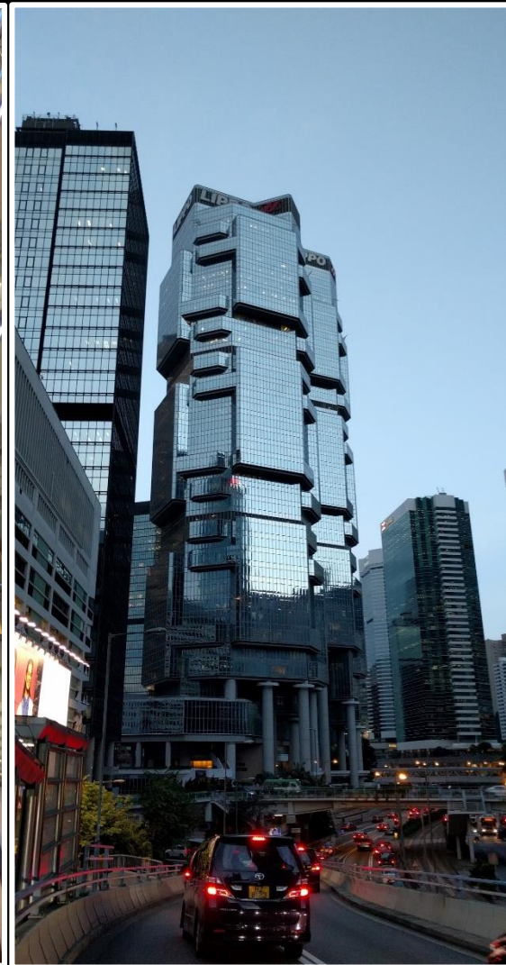
Lippo Centre Paul Rudolph
