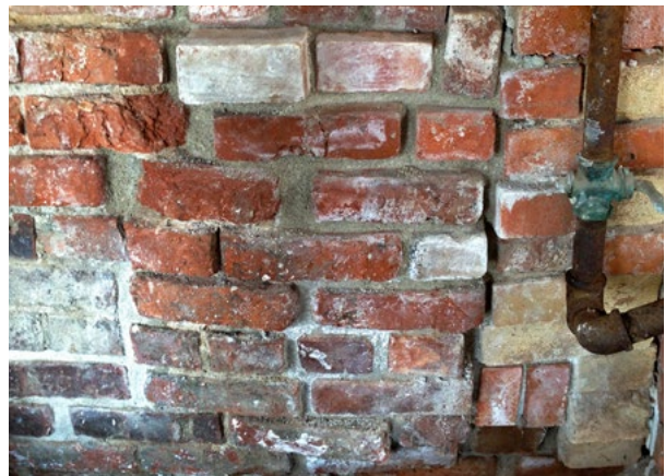
A large void on the northwestern face of Kiln No. 7 was grouted, pinned, and partially rebuilt by Kevin Wohlgenuth and Lindsay Bates.
