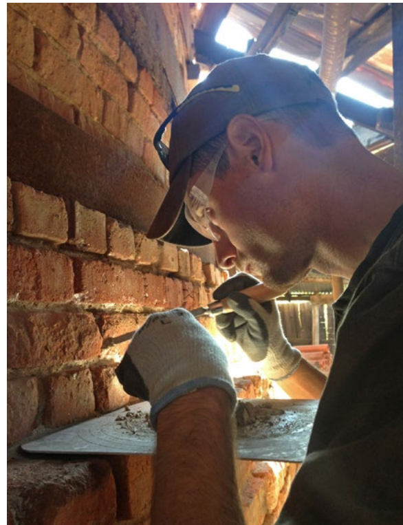
In the Zone: Student Matt Morgan focuses on repointing mortar joints along the southwestern face of Kiln No. 7. Photo: N. Iyer
