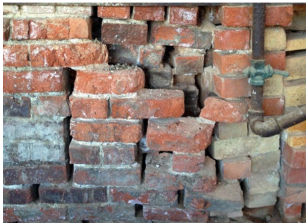
A large void on the northwestern face of Kiln No. 7 was grouted, pinned, and partially rebuilt by Kevin Wohlgenuth and Lindsay Bates.
