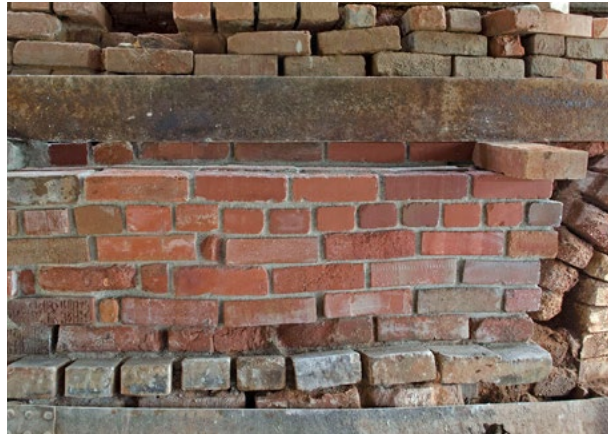
The partially collapsed, second tier of masonry on Kiln No. 7's southeastern face was rebuilt by Sarah Cole and Johanna Sztokman, who took care to maintain the brickwork's original bonding pattern.
