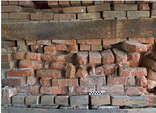
The partially collapsed, second tier of masonry on Kiln No. 7's southeastern face was rebuilt by Sarah Cole and Johanna Sztokman, who took care to maintain the brickwork's original bonding pattern.
