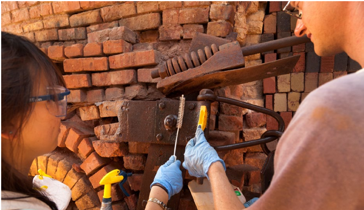
Staying on Task: Shuyi Yin and Benjamin Doubledde wash metal components on Kiln No. 7 with a desalinating agent. The continuation of conservation work at Western Clay will depend on the development of a vision for the future utilization of the site. Photo: J. Elliott
