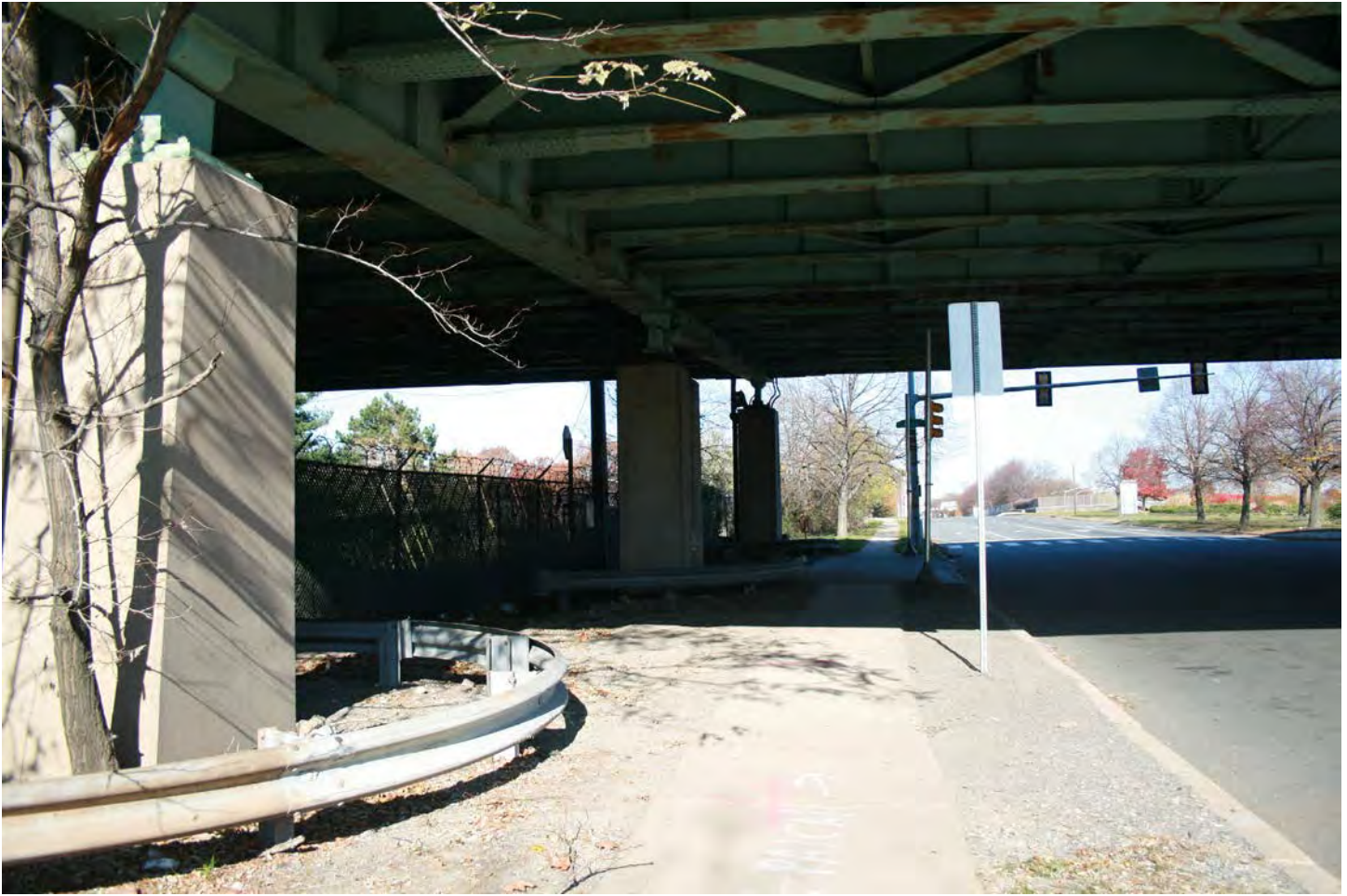
Fig. 8.I.7. The sidewalk leading from the Navy Yard to FDR Park passes underneath Interstate 95
