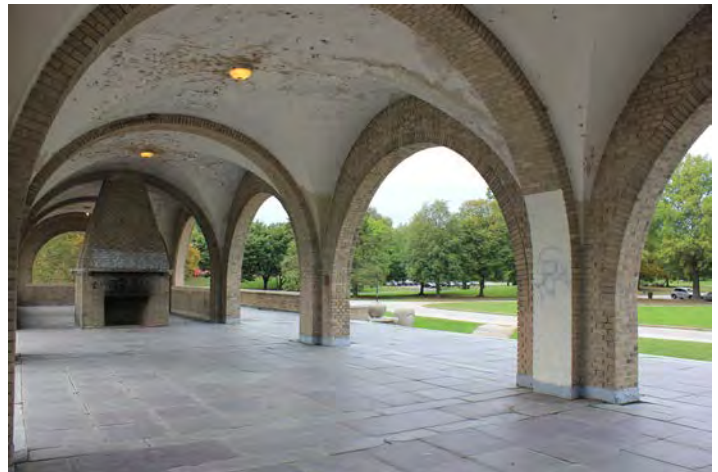
Figure 2.2.2. The interior of the pavilion is embellished with a groin vaulted ceiling, structural brick arches, and a grand floor to ceiling brick fireplace to the east. (E. Lissy)
