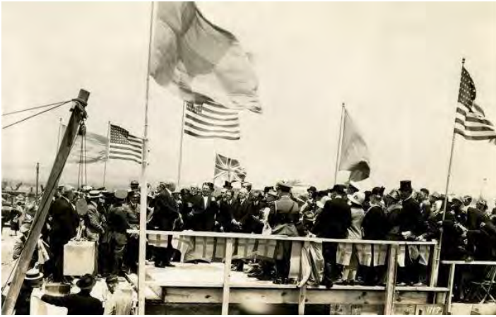
Figure 8.3-7. The Swedish Colonial Society lay the cornerstone for the John Morton Memorial Building as part of a heritage ceremony. DOR.
