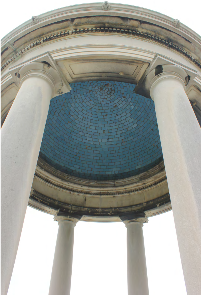
Figure 2.2.6. The dome of the gazebo is covered in blue ceramic tiles, most likely associated with Guastavino tiles, and carved stone trim. (A. Kress)
