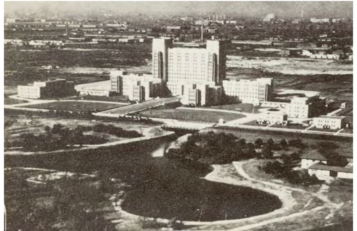
Fig. 8.I.I7. The Naval Hospital, 49 acres, demolished in 2001
