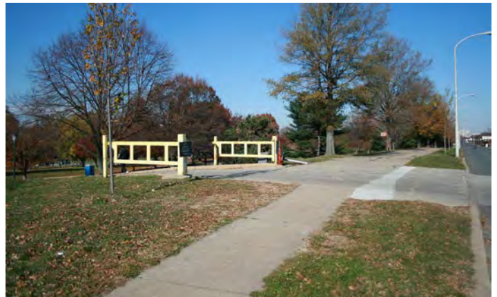
Fig. 8.I.9. The S. Broad St. entrance to FDR Park
