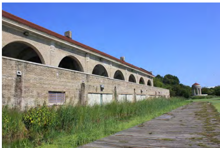
Figure 2.2.4. The classically designed gazebo, located to the east of the boathouse, as seen from the docks. (E. Maust)
