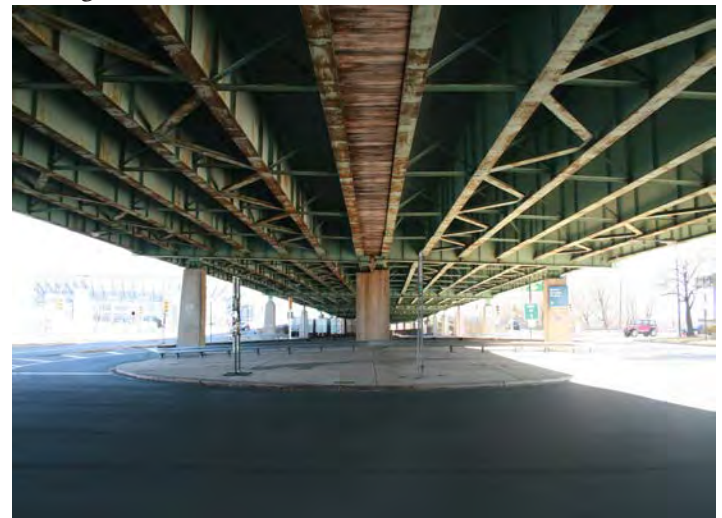
Fig. 8.I.9. Interesting architecture under the highway can be viewed from the Navy Yard to FDR Park sidealk
