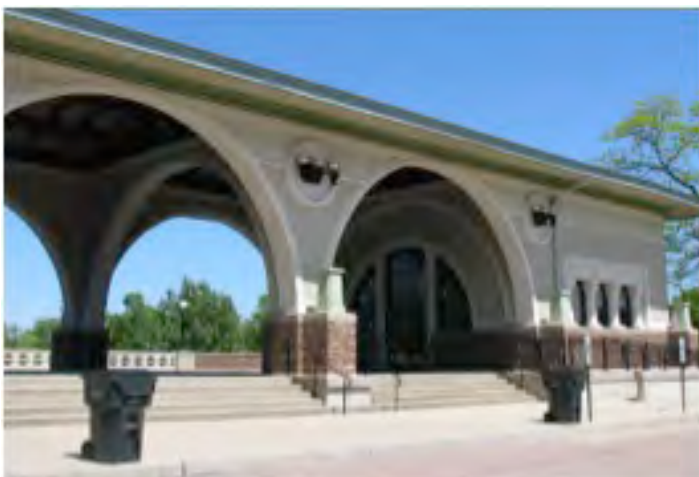
6.3.4 Front Entrance View of Humboldt Boathouse (Courtesy of Bauer Latoza Studio)
