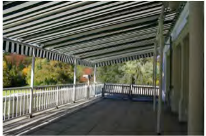
Figure 6.I.2. The second level open pavilion of the boathouse.
