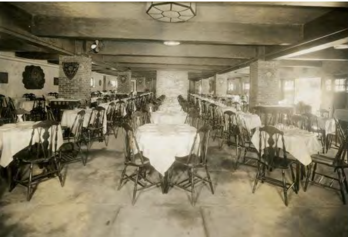
Figure 8.3-17. Interior view of the lower level of the Russian Tea Room. DOR.
