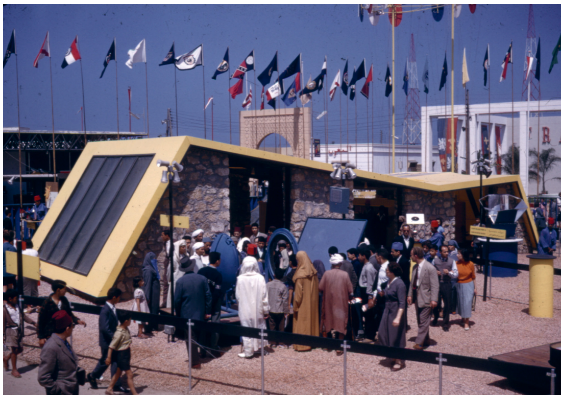
The Casablanca Solar House, by John I. Yellott and Charles Shaw, exhibited at the United States Department of Commerce Trade Fairs in Morocco in 1958, had a sloping roof to maximize solar incidence on an array of phase-change solar heating panels. Source: Department of Archives and Special Collections, Arizona State University, International Solar Energy Society Archive.
