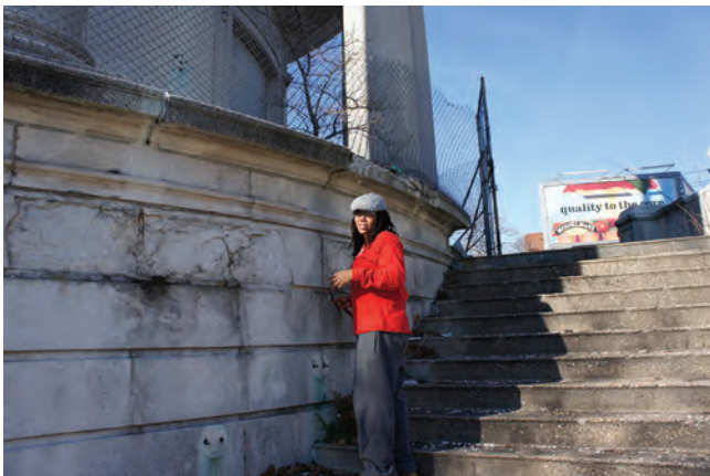
Figure 5. Conditions assessment work, Source: Germantown Town Hall Studio
