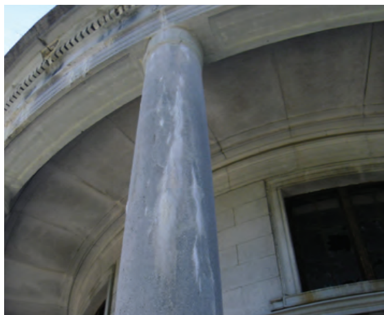
Figure 50. Image of efflorescence, Source: M.Rhodes
