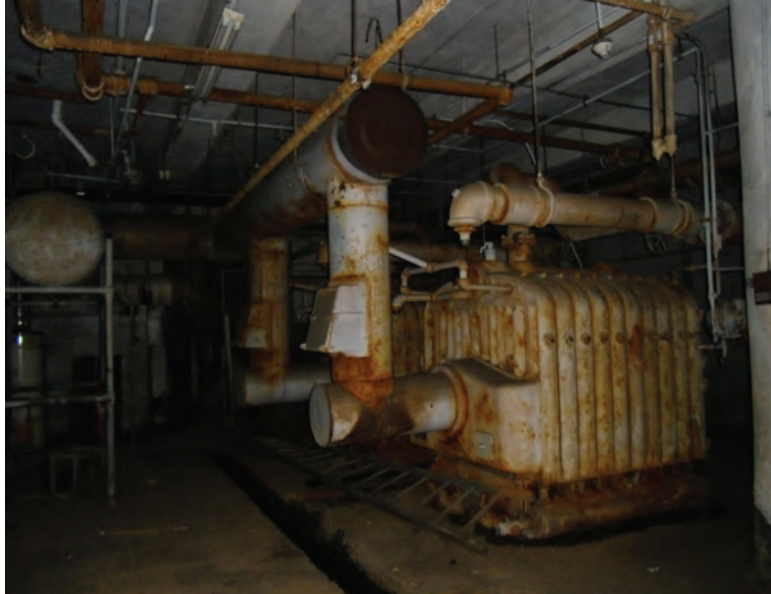
Figure 31. Boiler in basement, Source: Germantown Town Hall Studio 2011
