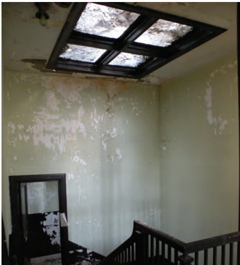
Figure 83. View of 3rd floor landing, Source: M. Wicklund, 2011
