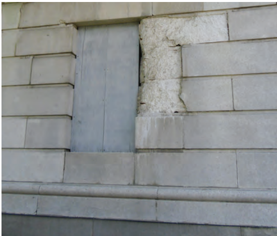
Figure 41. Disaggregation at northeast elevation, Source: L. Allen
