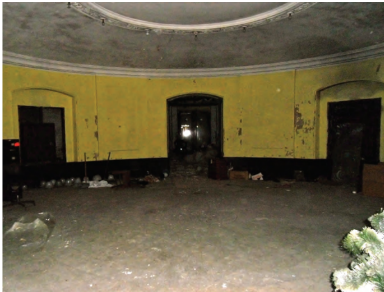
Figure 32. Ground level area below Rotunda, Source: Germantown Town Hall Studio 2011
