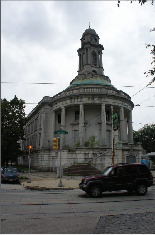
Figure 26. Germantown Avenue elevation, looking southwest from Haines Street, Source: Germantown Town Hall Studio 2011
