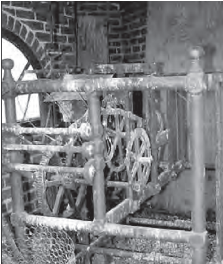
Figure 18. Image of Lukens clock fram and gears in tower prior to 2008 removal, Source: Lukens Clock + Stereoview Return to Independence Park , p.2.
