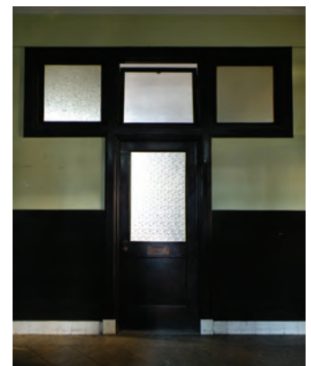
Figure 81. Image of typical door, Source: M. Wicklund, 2001
