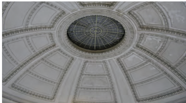
Figure 35. Figure 9: Rotunda and domed ceiling with oculus, Source: Germantown Town Hall Studio 2011
