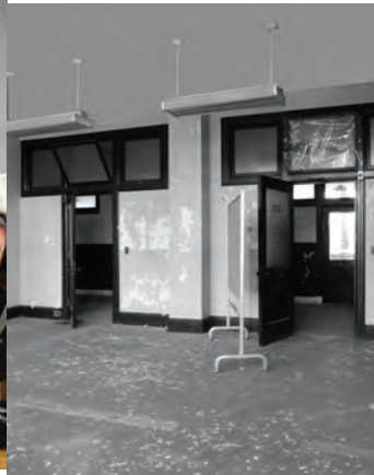
Figure 77. Caption: View of exiting 2nd floor room, Source: L.Allen, 2011
