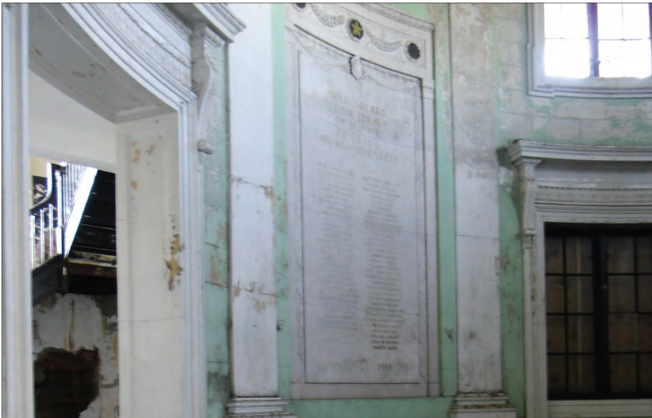
Figure 61. Interior image of GTH Rotunda, Source: L.Allen, 2011
