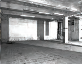
Figure 79. View of exiting basement, Source: M.Wicklund, 2011
