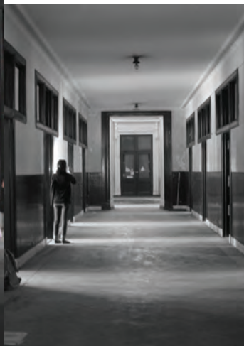
Figure 75. View of exiting 2nd floor hallway, Source: L.Allen
