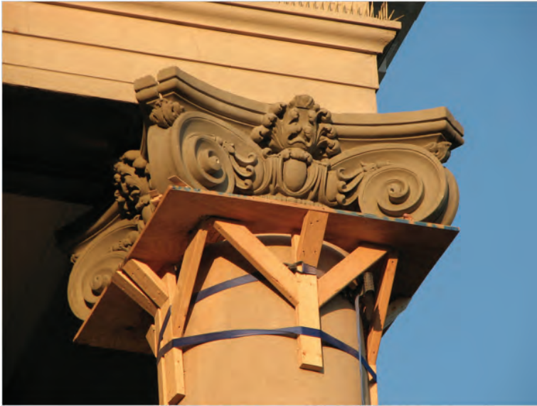
Figure 51. Image of glass fiber column capital, Source: Keystone Waterproofing inc
