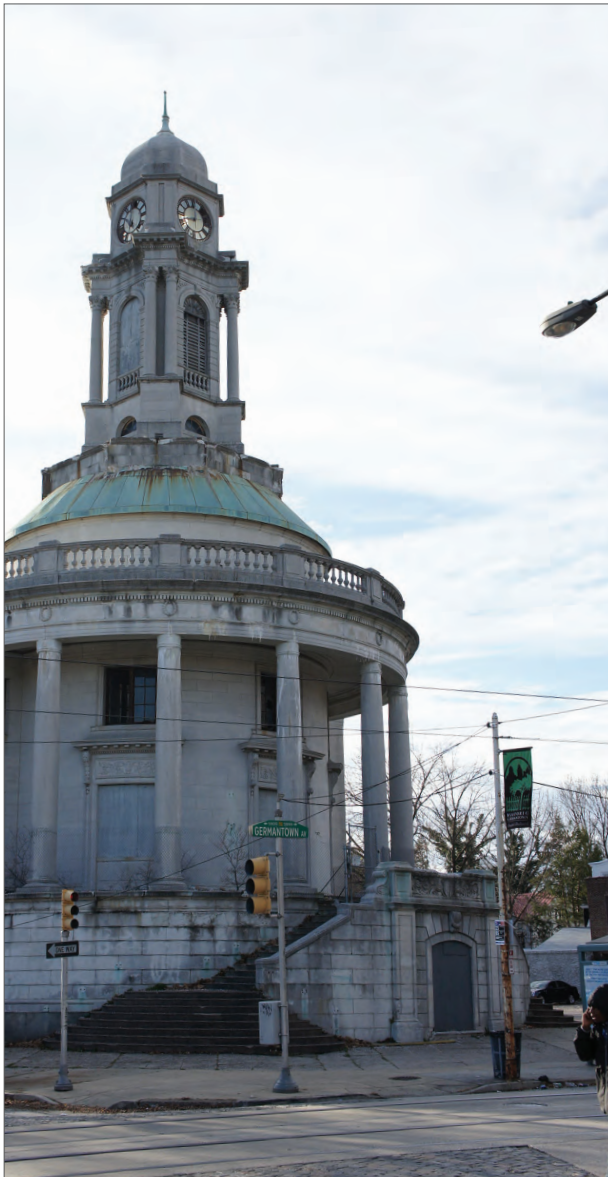
Figure 10. Image of Germantown Town Hall, looking west from Haines Street, Source: M. Rhodes, 2011
