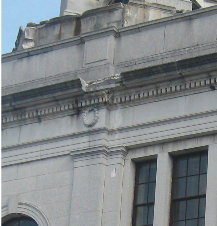
Figure 39. Detail of west elevation, Source: K.McNabb, 2011
