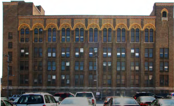
North Elevation facing Brandywine Street
