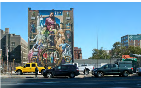
West Elevation facing Broad Street
