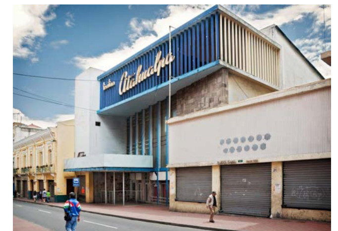
FIGURE 2.07 - Teatro Atahualpa, exterior view
