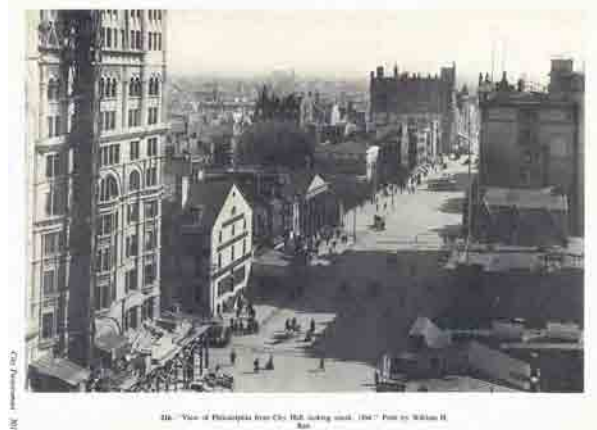
Figures 3-16: The northeast corner of Chestnut and Broad Streets in 1894 with a tall office building going up at the site of the telegraph office, showing the huge change in the landscape resulting from the mass migration of the banks into this area of Philadelphia.
