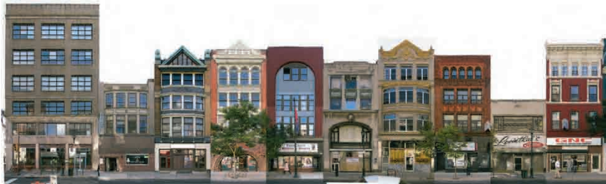
Figure 5-5: South side of the 700 block of Chestnut Street
