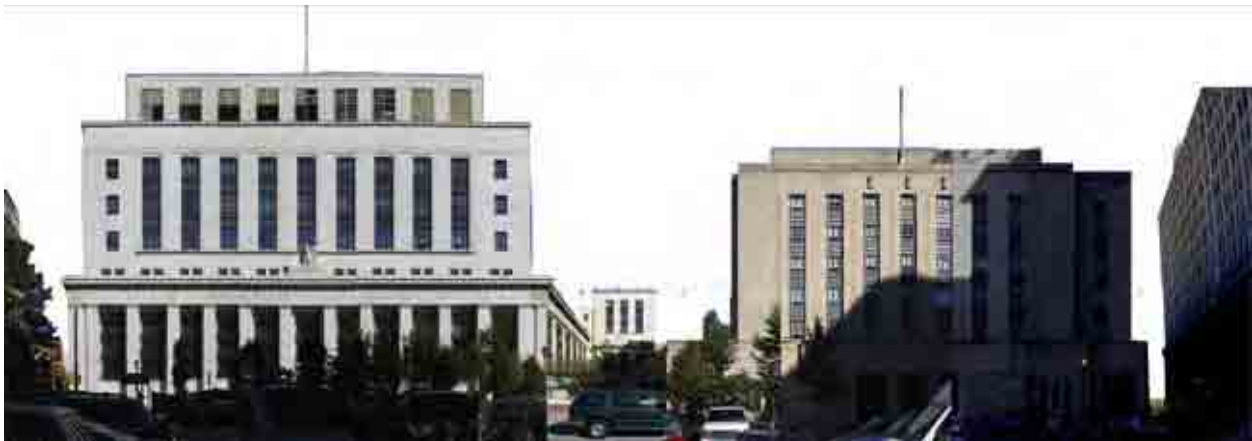
Figure 5-6: North side of the 900 block of Chestnut Street
