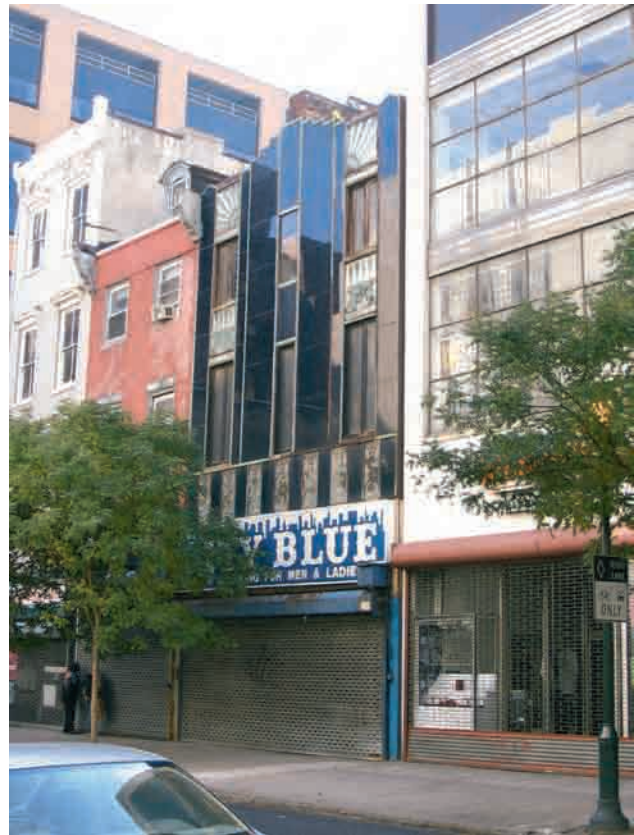
Figure 5-8: South side of the 1100 block of Chestnut Street
