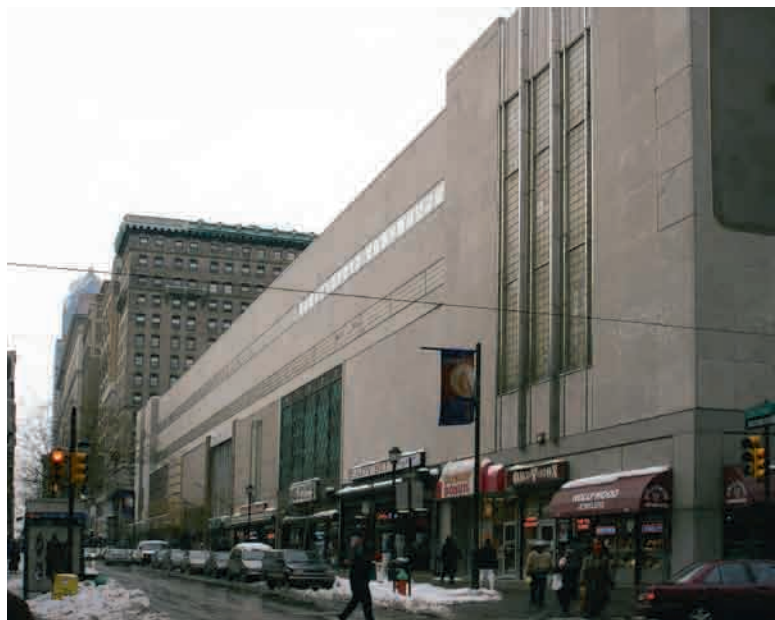
Figure 5-7: North side of the 1100 block of Chestnut Street
