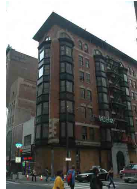
DeLong Building, corner of 13th and Chestnut.
