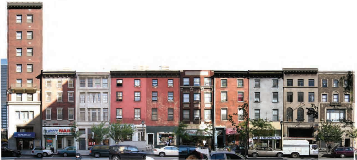
Figure 5-11: North side of the 1900 block of Chestnut Street.
