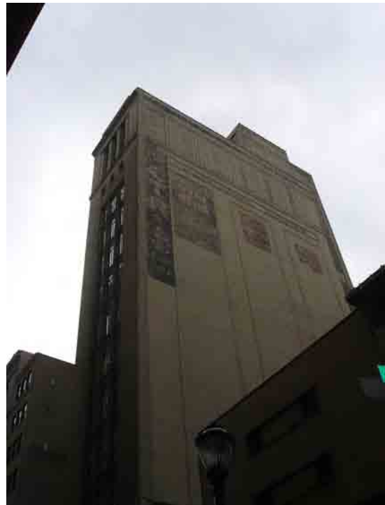
Figure 3-25: The narrow footprint of the Cunningham Building on the 1300 block shows the real estate value of the street in the early twentieth century: each square foot of land was put to maximum use.
