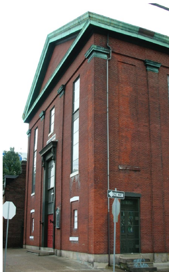
Kensington Methodist Church "Old Brick Church"
