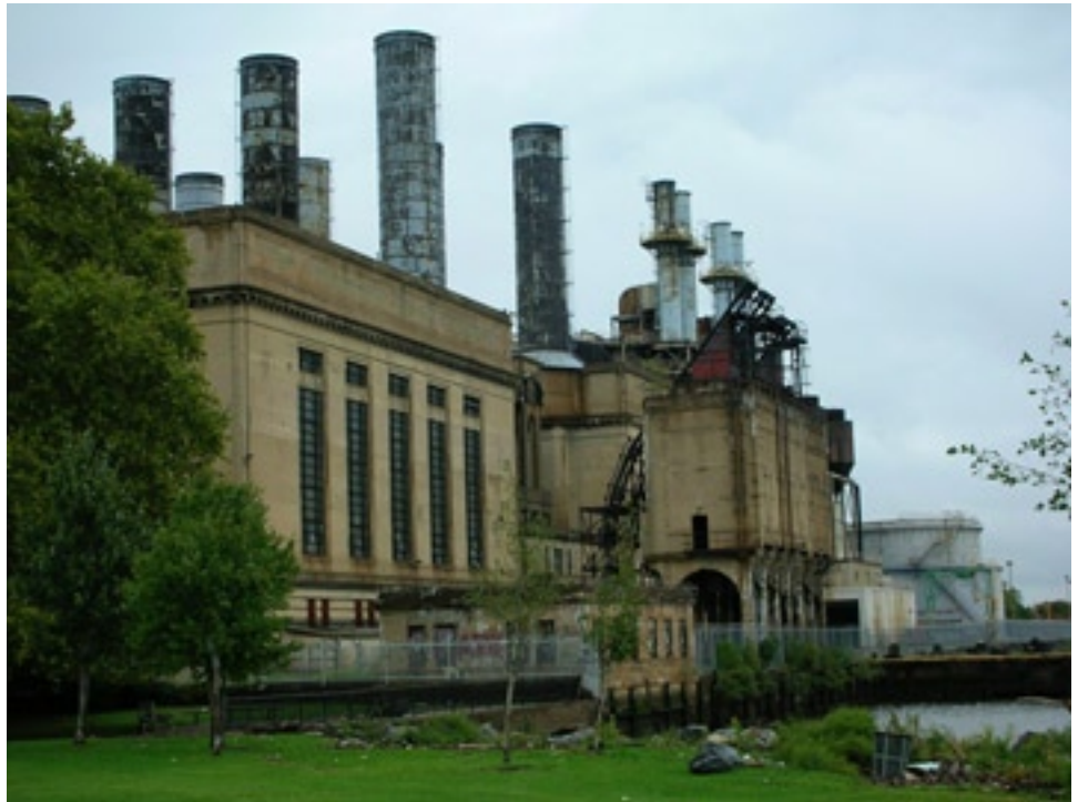
Fig. 12:PECO plant. Source: Ellen Buckley
