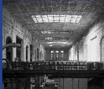
TURBINE HALL: PHOTO COURTESY OF JOE ELLIOT
