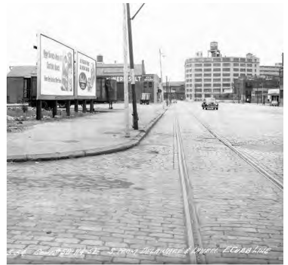
Delaware Ave, bridged factory in distance, 1954
