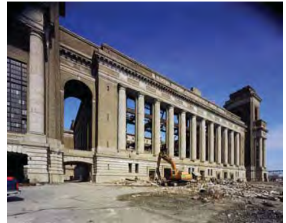
Figure 11: Chester Station during construction. Source: Blackney Hayes Architects.
