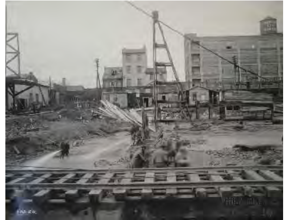
Figure 8: Site work for construction of Delaware Station, Photo taken 24 Oct 1919. Source: PECO Archives.
