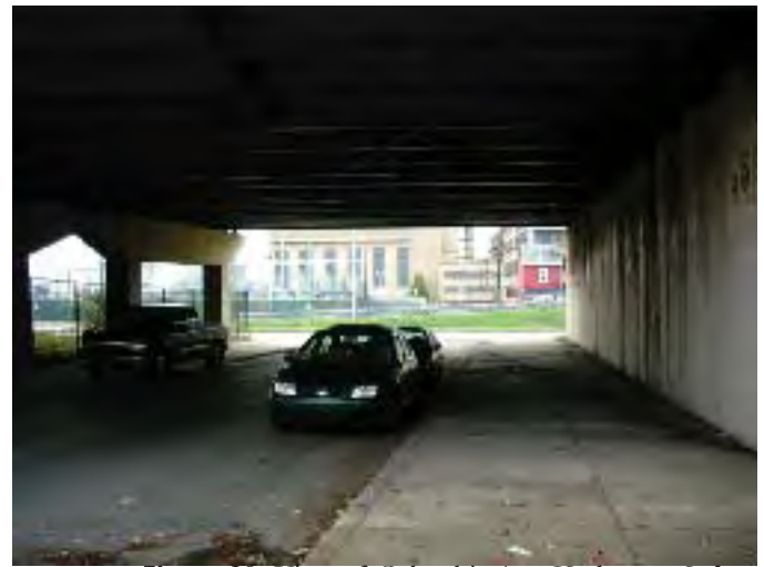
Figure 21: View of Columbia Ave. Underpass Before Improvements.
