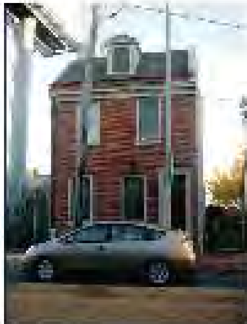
1. VIEW FROM 20' NORTH OF THE HOUSE 10/15/12
