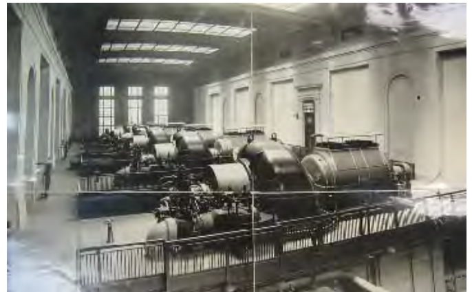
Figure 10: Interior of Turbine Hall, Delaware Station. Source: PECO Archives.
