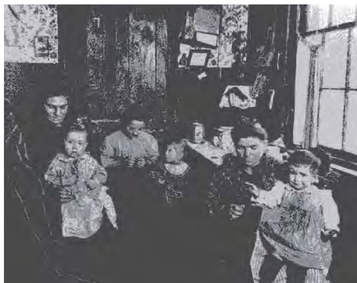
Mothers and children doing piece work in the home Work Sights: Industrial Philadelphia, 1890 – 1950
