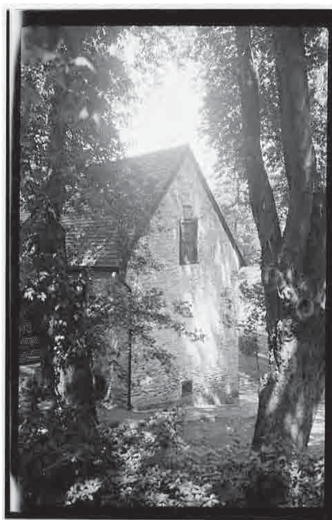
207 Lincoln Drive. (Source: Historic American Buildings Survey)
