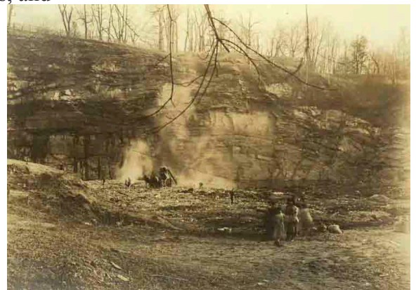
Quarry near Historic RittenhouseTown. Undated. (Source: Shouemaker Collection, Free Library of Philadelphia)
