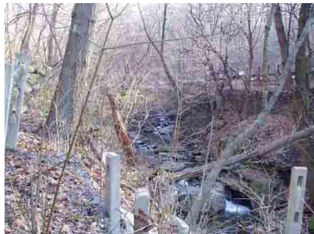
Figure 9. View of the remains of the Amnidown Mills. (Source: Reagan Ruedig)
