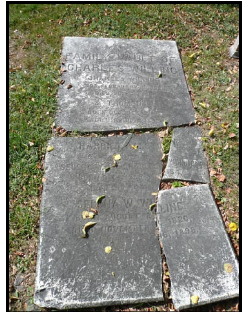
A severely cracked slab. Cracking can lead to partial loss of the marker and total loss of fragments.
