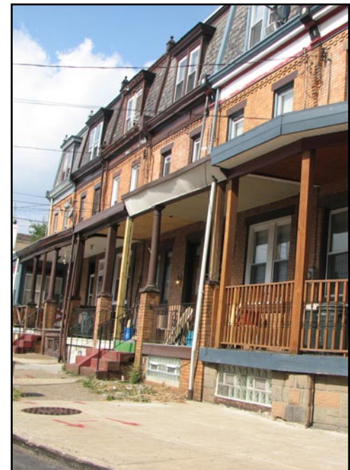
Strawberry Mansion Neighborhood, along Ridge Avenue. Photo: T. Aphale 2007.
