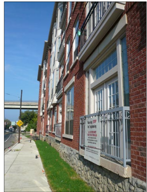
Dobson Mills apartment development. The side facing Ridge Avenue consists of unusable doors and air conditioning units, preventing active use of the sidewalk. Photo: M. Goeke 2007.
