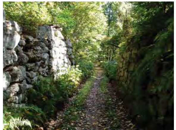
The Five-mile Tree Overpass.
