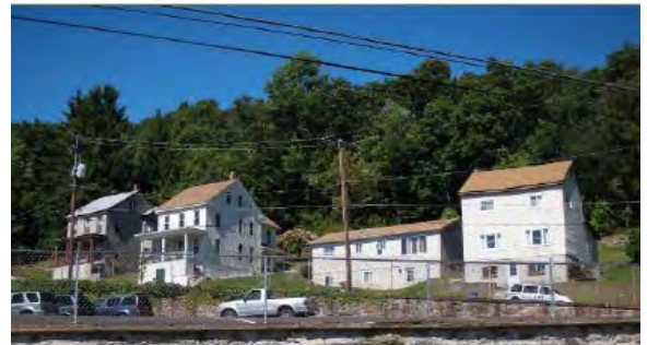
The Studio Team surveyed residences in the Heights, including these single- and multi-family homes along North Avenue at the base of Mount Pisgah.
