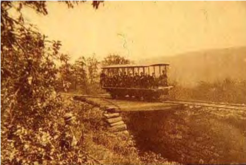
Historic Image of The Five-mile Tree Overpass. Photograph courtesy of the Mauch Chunk Museum. http://www.mauchchunkmuseum.com/PhotoArchives
