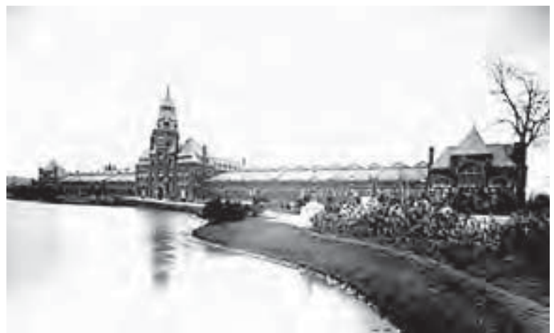
Fig. 2.3.5: View of the South Factory Building along the artificial lake. Source: http://www.chicagohs.org/history/pullman.html .
