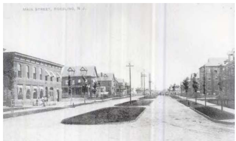
Fig. 2.3.13: Main Street in Roebling, facing the Main Gate, 1910. Source: Images of America: Roebling .
