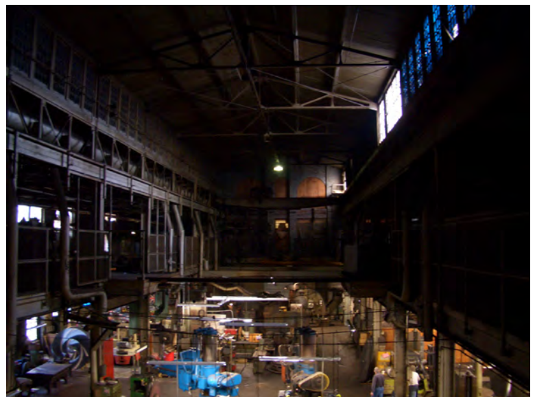
Fig. 5.2.14: Interior of Building 7, showing the steel-framed clerestory roof structure.
