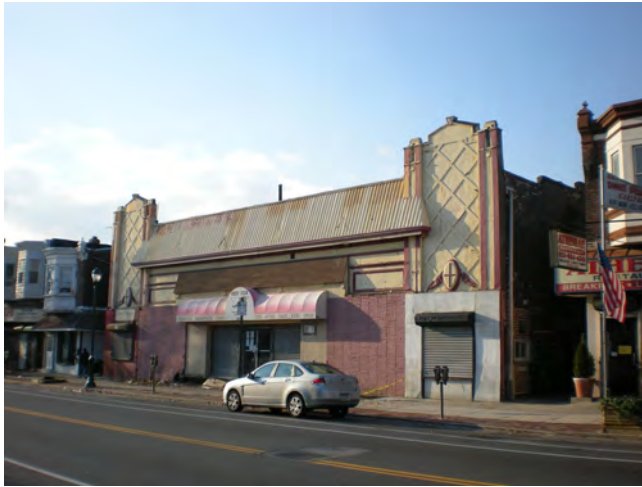
Fig. 5.3.11: Many important historic resources, like the former Liberty Theatre located at 6814 Torresdale Avenue, are currently underutilized but exhibit potential for future renovation and adaptive reuse in commercial corridor redevelopment efforts.
