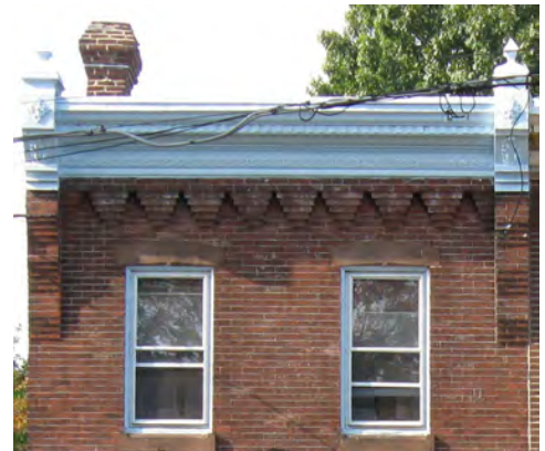
Fig. 5.4.5: 6710 Keystone Street, detail of corbelling and brackets
