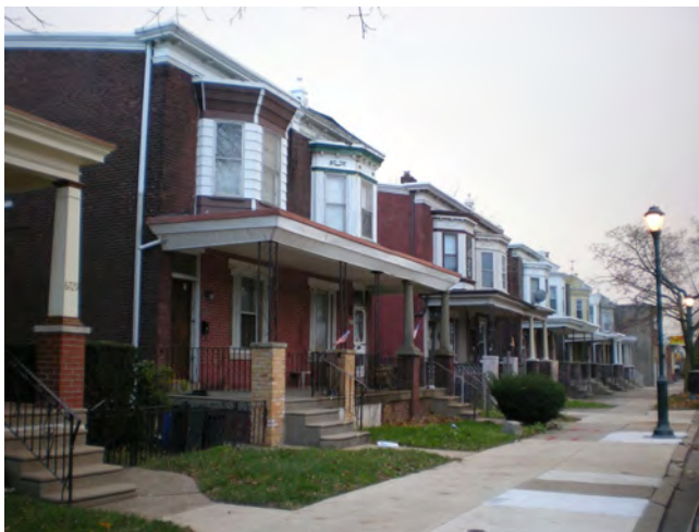
Fig. 5.3.12: The residential structures included within the boundaries of the Torresdale Survey generally exhibit good condition and upkeep. Here, vinyl siding obscures architectural details at the nearest house, while historic details can be seen down the street at the upper story bay windows.
