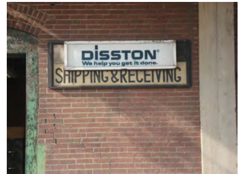
Fig. 5.2.10: Disston Precision currently occupies a complex of buildings on the site.
