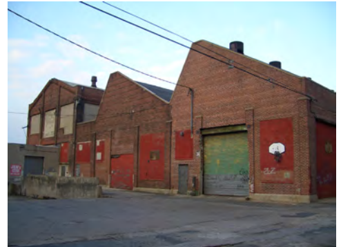
Fig. 5.2.24: Modern alteration to the roofscape of Building 3.
