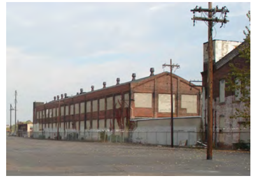
Fig. 5.2.7: Buildings façade along capped brownfield.
