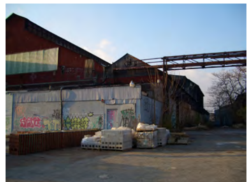
Fig. 5.2.25: Lean-to addition to the north side of Building 1.
