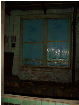
Fig. 5.2.21: Blueboard infill within second story window of Building 7.
