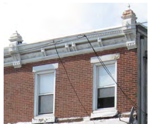
Fig. 5.4.7: 6824 Hegerman Street, detail of cornice and brackets
