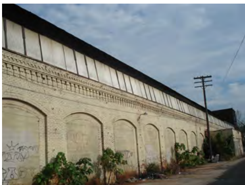
Fig. 5.2.22: CMU aperture infill along south side of Building 1.
