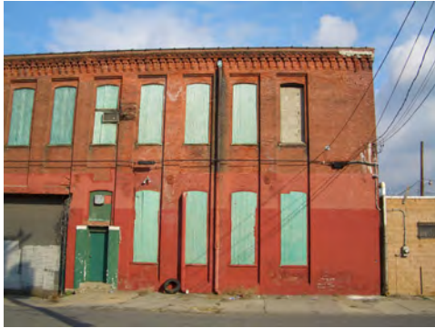
Fig. 5.2.20: Typical corrugated asbestos aperture infill.
