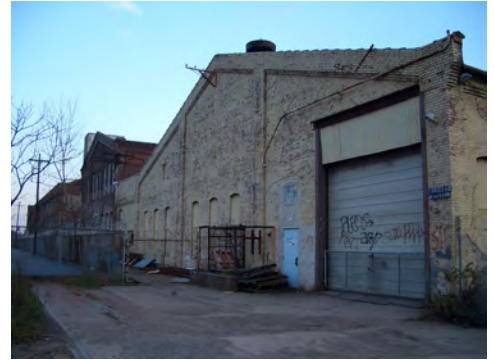
Fig. 5.2.23: Cut opening to allow for a modern garage door along north west facade of Building 4.
