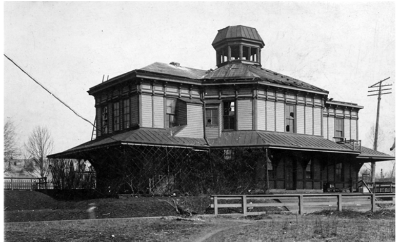
Fig. 4.2.1: Tacony RR Station after Windstorm March 27, 1911. Courtesy Tacony Historical Society Archives
