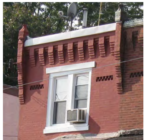
Fig. 5.4.6: 6820 Hegerman Street, detail of corbelling and brackets
