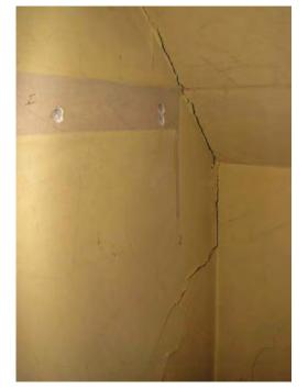
Image 13. Room 309 Cracking
