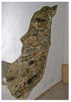
Image 15. Basement Foundation Material Loss
