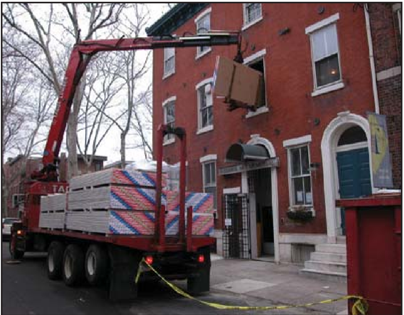
Figure 3.1.2. Loading drywall into 713 Catharine Street, 2005. Credit: www.fleisher.org/about/renovations.php
