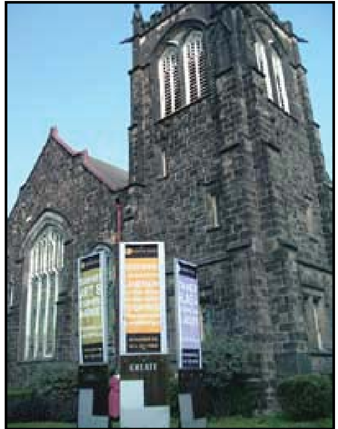
Figure 5.1.1.3.1. Union Project, former Union Baptist Church, Pittsburgh, PA. Credit: www.unionproject.org/ .
