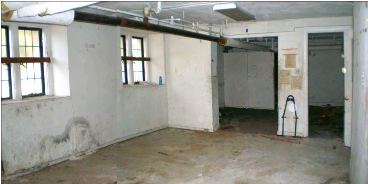
Figure 7 Existing conditions of the ground level of the deanery, 2010.
