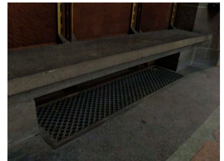
Figure 6 Vent grilles, nave floor, 2010.
