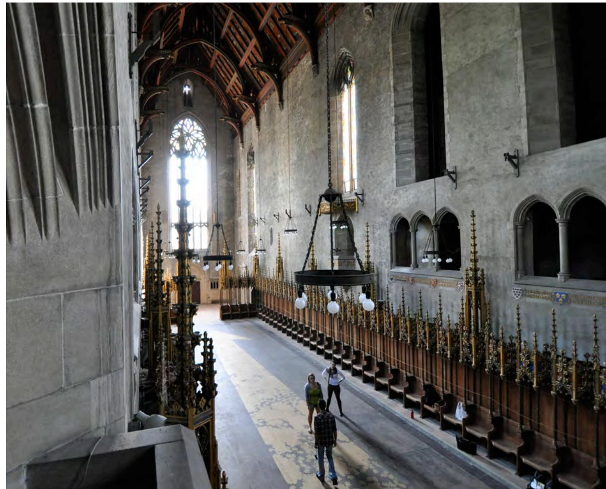
Figure 8 View of sanctuary from above showing the existing plywood floor
