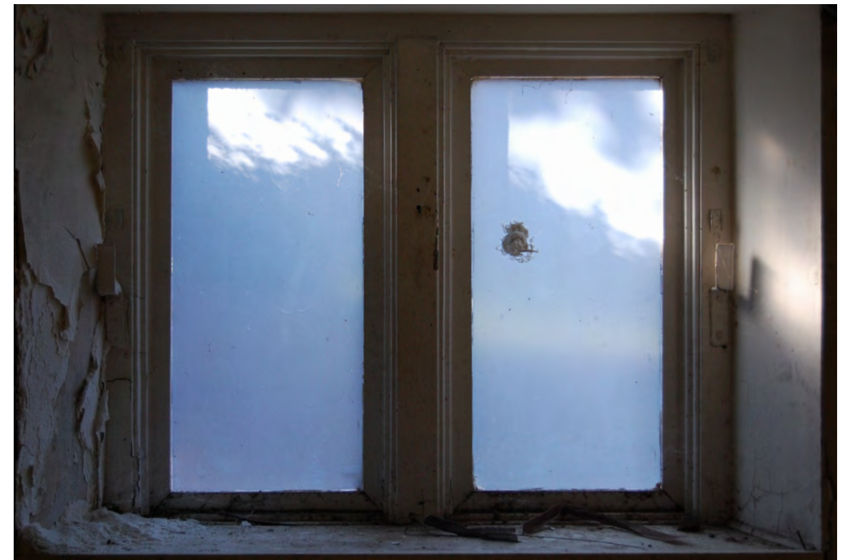
Figure 8 Casement replaced with insulated sash and glass in deanery basement
