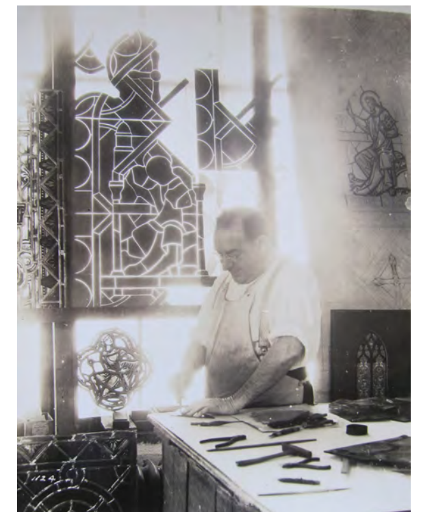
Figure 4 Nicola D'Ascenzo assembling individual pieces of glass.
