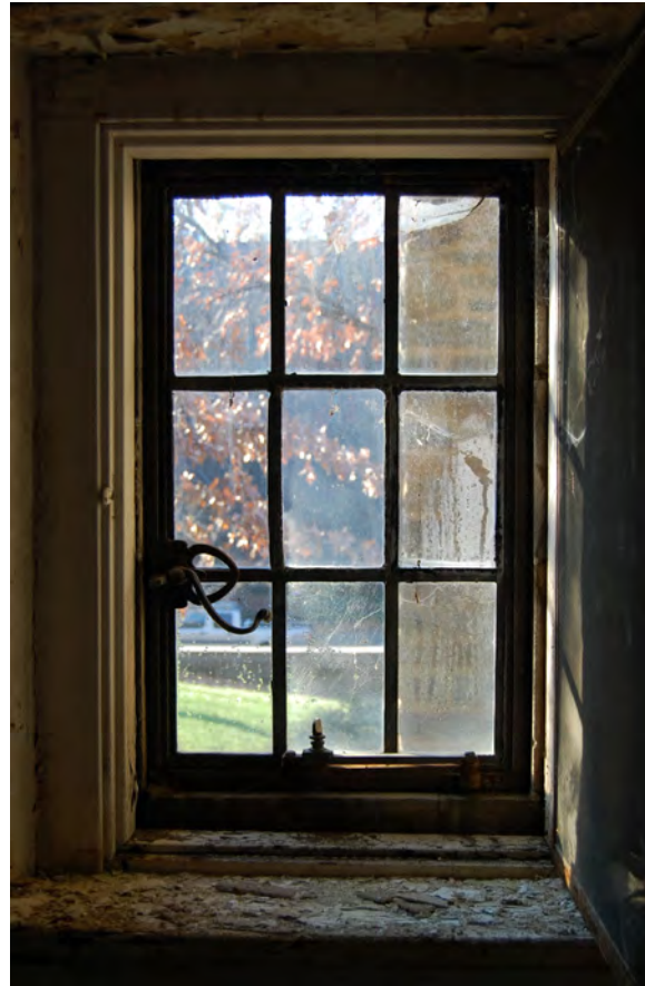
Figure 1 Leaded casement window in deanery
