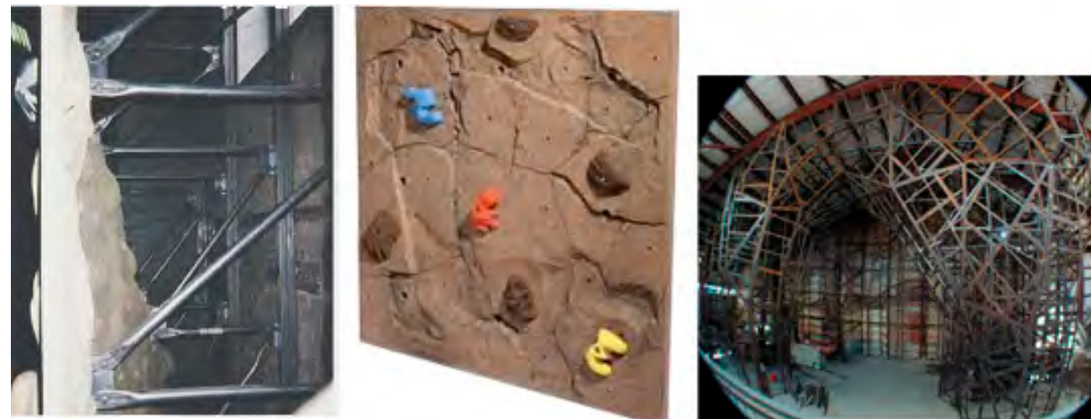
Figure 13 Attachment options for a climbing wall. From left: fiberglass reinforced concrete panels ( www.copecourse.com/climbingwalls.htm ); polyurethane surface panels that are anchored directly to a subwall or framing ( www.copecourse.com/climbingwalls.htm ); steel frame reinforced concrete ( www.athletiquet.com/indoor-rock-climbing.php ).
