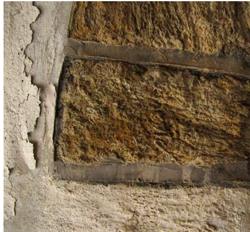
Figure 4 The texture and color of the schist changes as the feldspars decompose.
