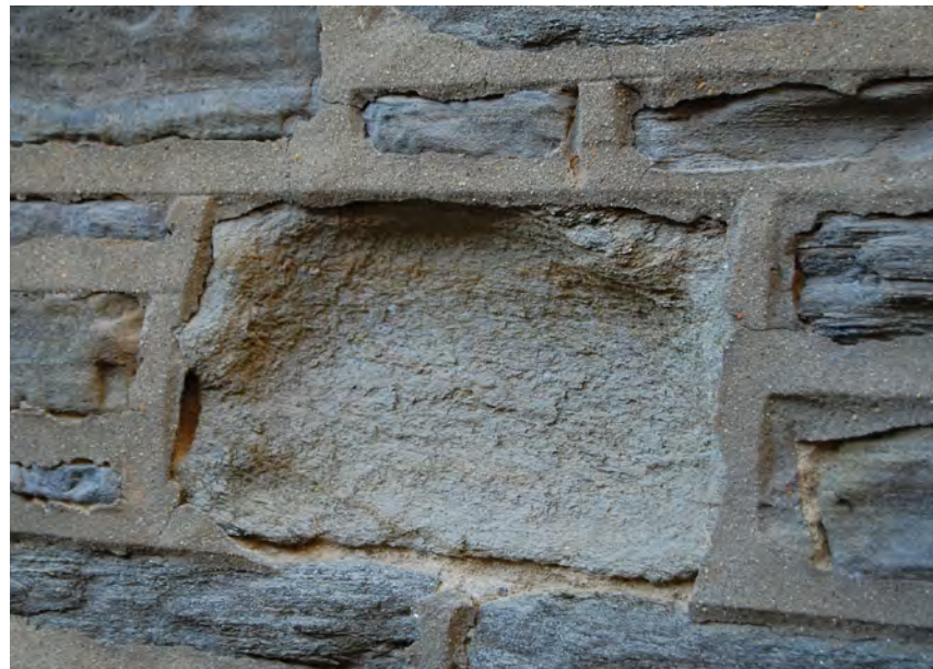
Figure 1 Delaminating schist
