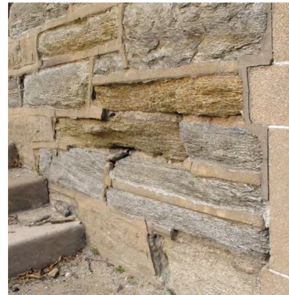
Figure 2 Decomposing schist on the southern elevation at the entrance to the crypt, exhibiting loss of material and brownish coloration.
