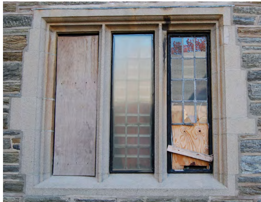
Figure 6 Center window has received additional glazing for protection from vandalism
