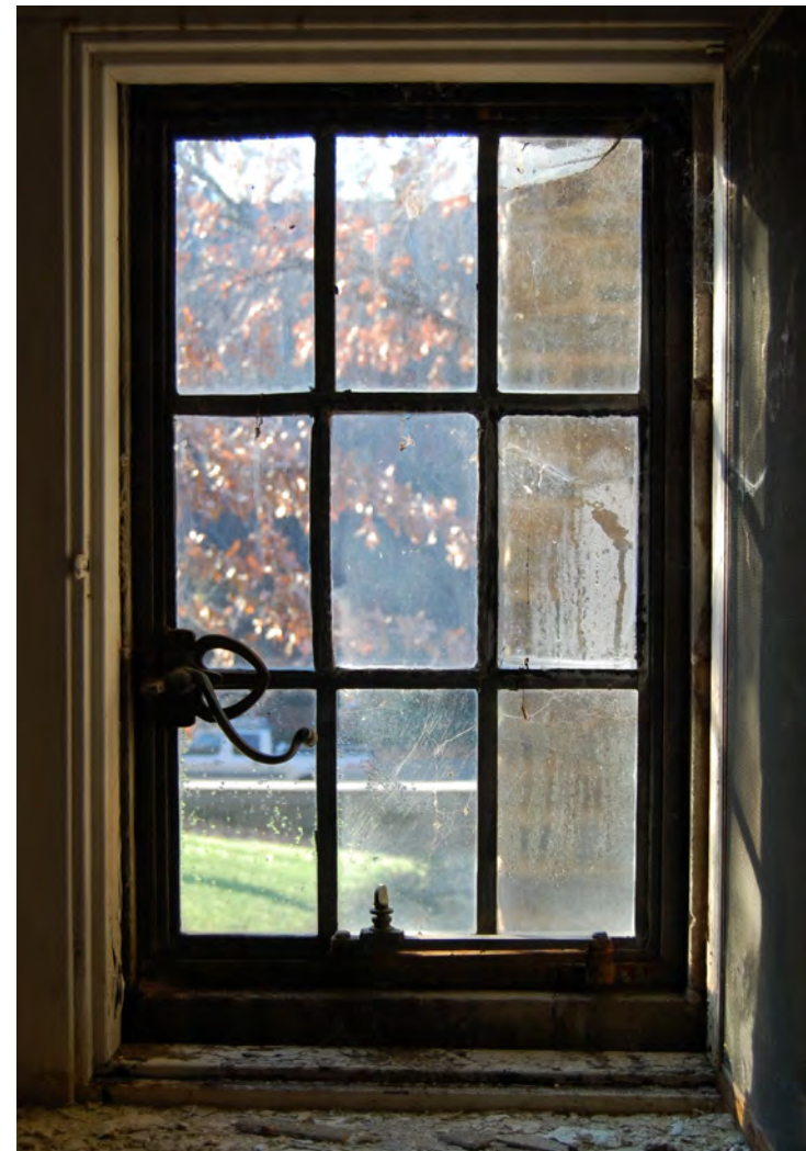
Figure 5 Characteristic iron window latch
