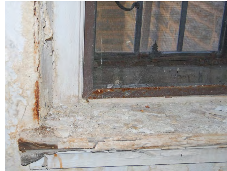
Figure 7 Interior screen set into wood jamb, possible location for interior casement storm window
