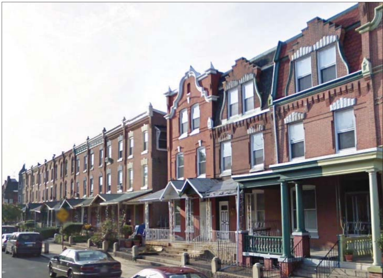
2.8 Rowhouses on 4000 block of Spring Garden Street
