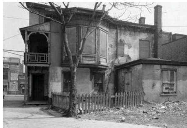
3.17 Dilapidated Victorian houses, ca. 1930
