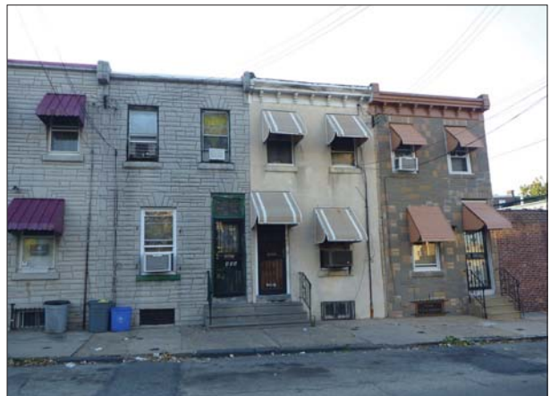
5.13 These rowhouses on N. Sloan Street are covered by stucco and permastone, but original historic fabric remains underneath
