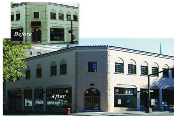
5.33 The Photo Art building in Portland, OR, before and after it was rehabilitated with new paint, windows, and doors
