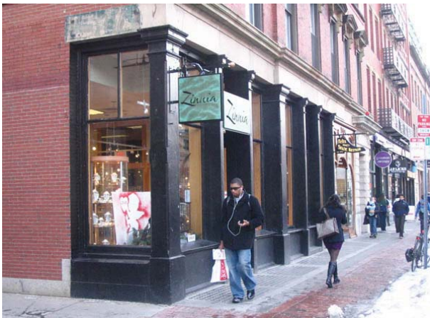
5.32 A renovated storefront in Cambridge, MA
