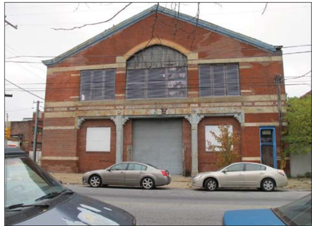
5.2 Terminal for the West Philadelphia Passenger Railroad at 4100 Haverford Avenue
