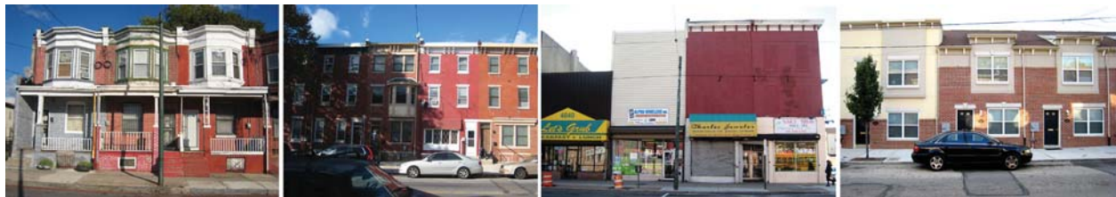
4.24 Building integrity (L-R): intact buildings, buildings with some alterations, buildings with many alterations, and infill
