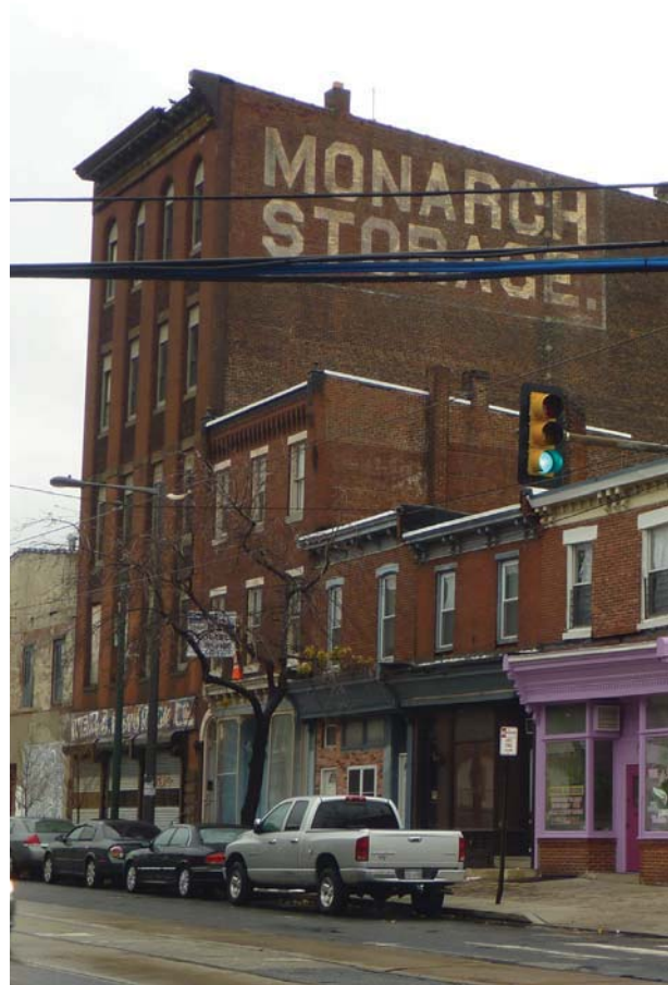
1 Monarch Storage Building, 3970-72 Lancaster Ave.
