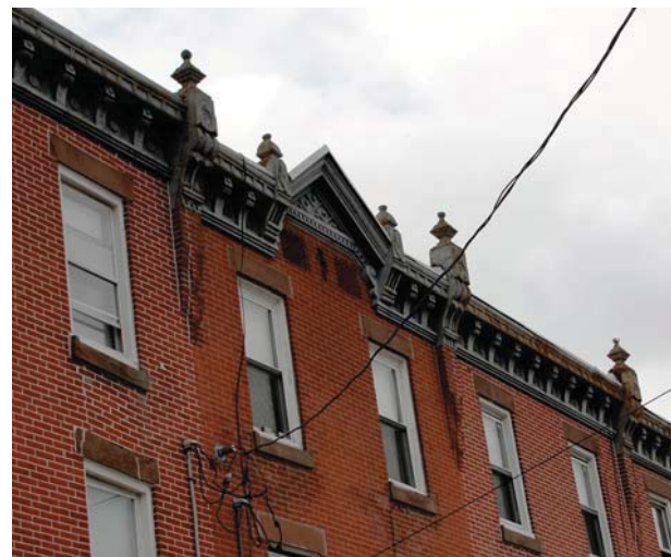
18 Brick façade with accent colors on cornice and decorative pediment. (A. Gonçalves)
