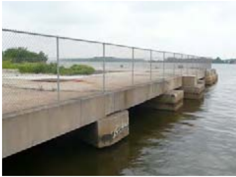
Pier on pilings
