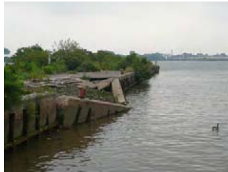
Pier with concrete bulkhead and rubble fill
