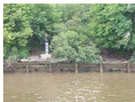
Pier with wooden bulkhead and soil fill
