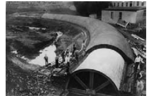
Mill Creek Sewer under construction, 1883 PWD Historical Collection
