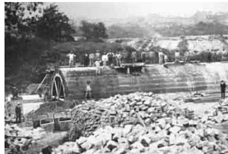
Wingohocking Creek Sewer under construction, 1909 City Archives of Philadelphia
