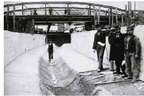
Aramingo Canal during its conversion into a sewer, April 1, 1901 PWD Historical Collection
