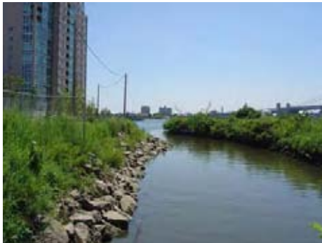
Rip-rap with backfill
