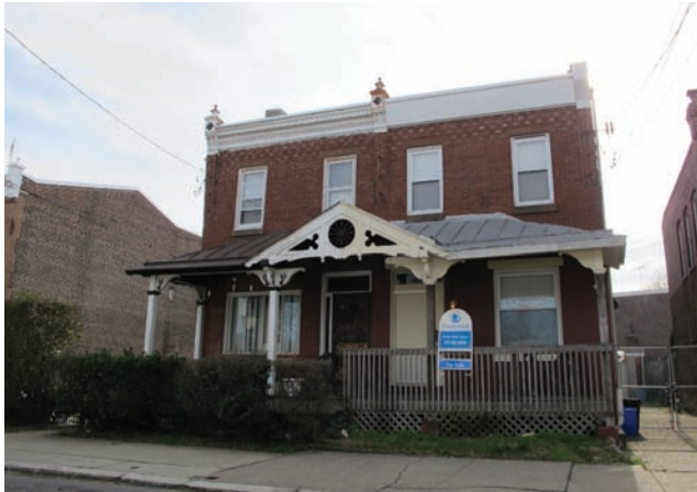
4.3 Part of high-integrity grouping with intact setting, design, and materials
