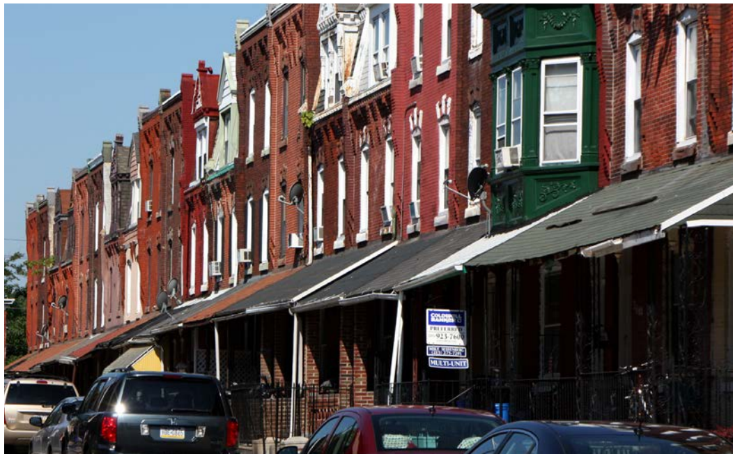
The corridor consists of many diverse districts -- residential, commercial, and institutional -- and also contains a wide variety of building types and scales. The Hub at 40 th and Chestnut (above) and residences at 40 th and Green (below) illustrate the architectural variety along the corridor.
