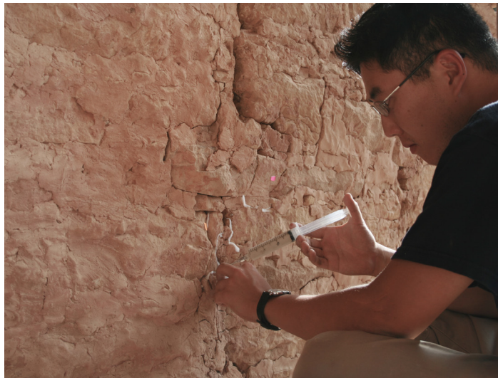
Above: Gelatin treatment of masonry wall (ACL)
