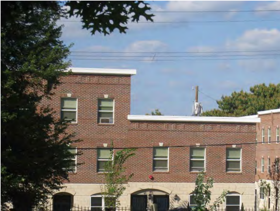
Figure 63: WCRP Housing. Fairhill Studio. 2009.
