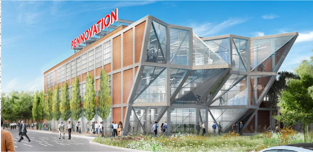
Rendering of the Pennovation Center under construction.
