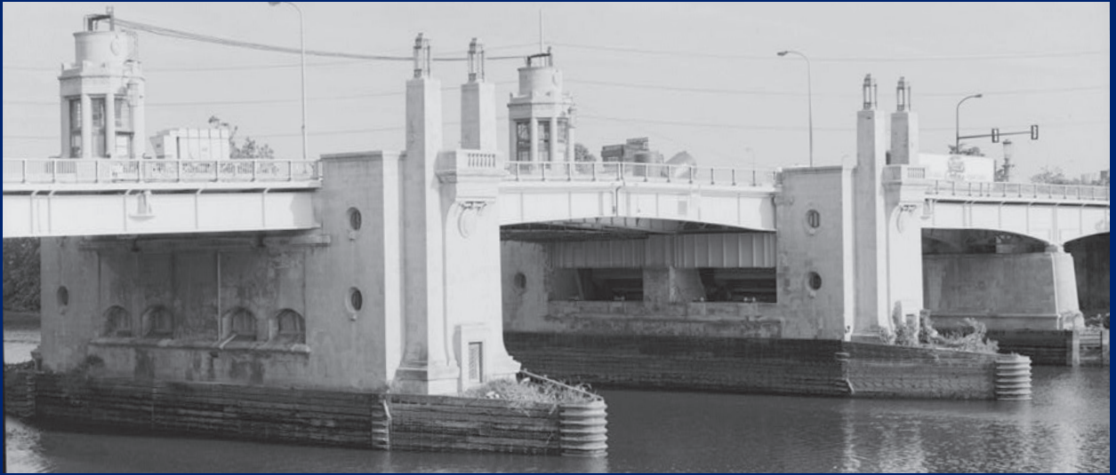
View of the 34th Street Bridge, looking southeast, 1998.
