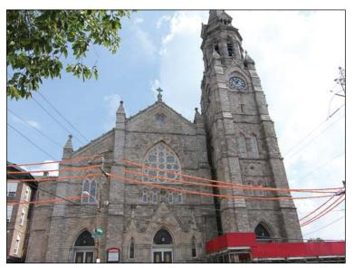
The stone exterior is in fair condition, with some areas showing much more damage than others. The tower at the northwest corner of the building is surrounded by scaffolding under which is a protected walking path, and repairs to secure the tower are ongoing. Some vegtation is growing on the tower.
