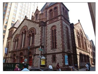
The building was under extensive renovations at time of survey. The masonry has some mortar loss and staining, but is in generally good condition. Windows (in worse condition than the doors) are in fair condition; frames and glass need some repairs. The asphalt shingle roof is in very good condition with no visible issues. Renovation plans do not include significant exterior alterations.
