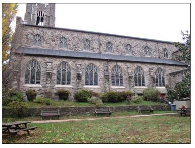
The masonry exhibits spalling, significant mortar loss, and staining throughout. The tower has clearly had structural issues that were repaired recently with incompatible patching. Some cracking still exists at the northeast elevation and at various buttresses (where mortar loss is also concentrated). A wood porch on the side elevation is in fair condition. Windows are in poor condition. The asphalt shingle roof is in fair condition, with some sagging sections.
