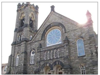
The church's schist walls and tower are extensively stained. The masonry also exhibits spalling, and vines are growing on the north elevation. Windows are in fair-poor condition, with frames that need repairs. Eight windows are broken or missing. The asphalt shingle roof is stained, and shingles look worn. Damage/patching are evident at the north end, near the tower.
