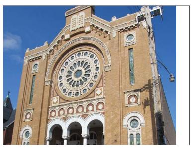
The primary elevation features yellow-brick walls in fair-good condition, while the secondary exterior walls are red brick and in fair condition. The masonry exhibits efflorescence and staining, particularly on the secondary elevations. Doors and windows are in fair-good condition, depending on the elevation; some frames on west elevation were being repaired at time of survey. Drainage is intact. The roof is not visible from the street and could not be assessed.
