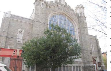
The masonry is in good condition overall, although various areas need repointing. The doors and windows are in fair condition; several windows have bowing or sagging glass. The asphalt shingle roof is in fair condition, with some missing shingles, sagging, and patches concentrated on the west end.
