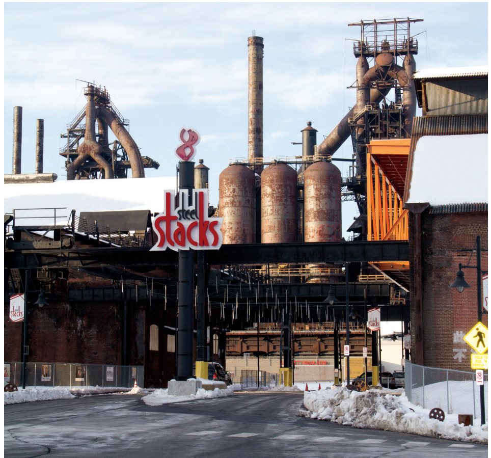
The Steel Stacks brownfield redevelopment in Bethlehem, PA, was built in conjunction with a Sands Casino. It is one of three redevelopment efforts being examined by the studio. Credit: Ryan Debold.
