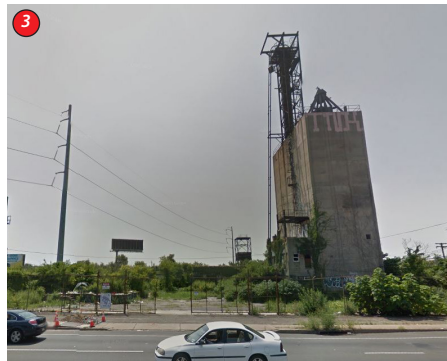
Coal Silo • Owned by PIDC • Working to obtain rights for remediation
