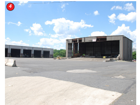
Waste Management • Owned by Waste Management with long term contract • They hold a non-transferable permit
