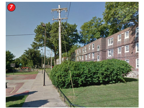
Bartram Village • Pennrose and Philadelphia Housing Authority will be redeveloping this site
