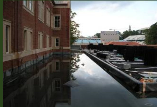
Testing the roof garden during construction
