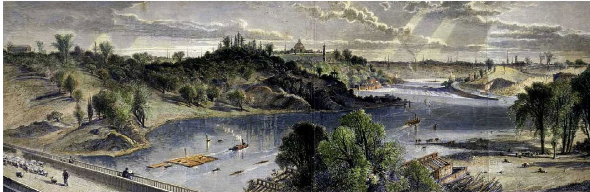
Fairmount Water Works from Columbia Bridge
