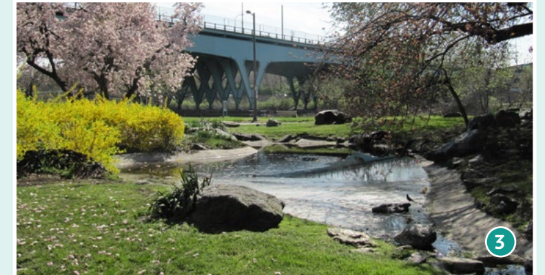
Glendinning Creek's path before it is culverted under Kelly Drive.
