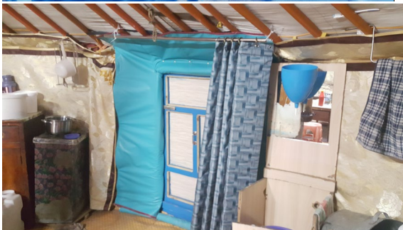
Figure 6. Toono cover (top) on ger D and door insulation (bottom) on occupied ger 4
