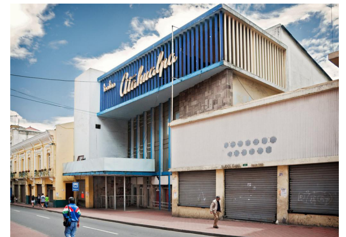
FIGURE 2.07 - Teatro Atahualpa, exterior view
