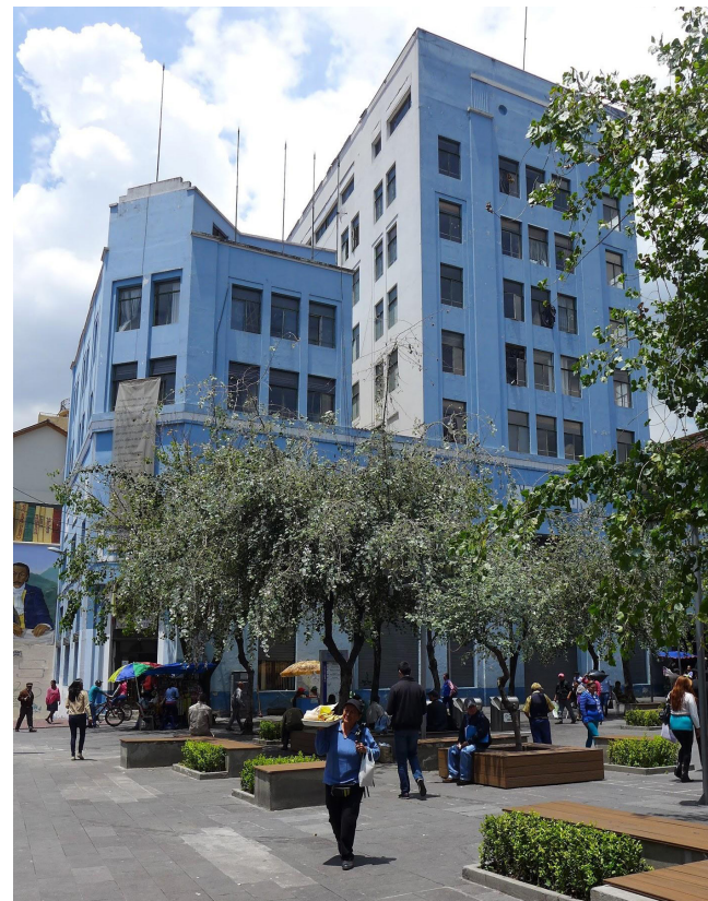
FIGURE 2.11 - Ex Hotel Humboldt | Edificio la Previsora with the front public plaza
