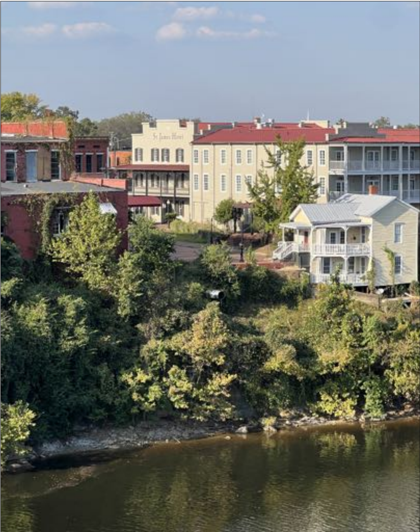
Figure 5.1 : Looking Northeast from the Edmund Pettus Bridge to the St. James Hotel and Alabama Riverfront.
