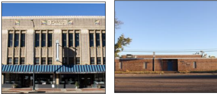
Figure 2.40 : Downtown Buildings (Left) Kress Building, (Right) Masonic Temple
