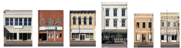
Figure 3.19: Main street Commercial Building.
