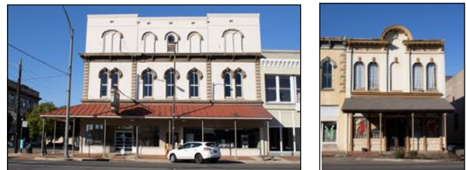
Figure 2.30 : West Side of Broad Street
