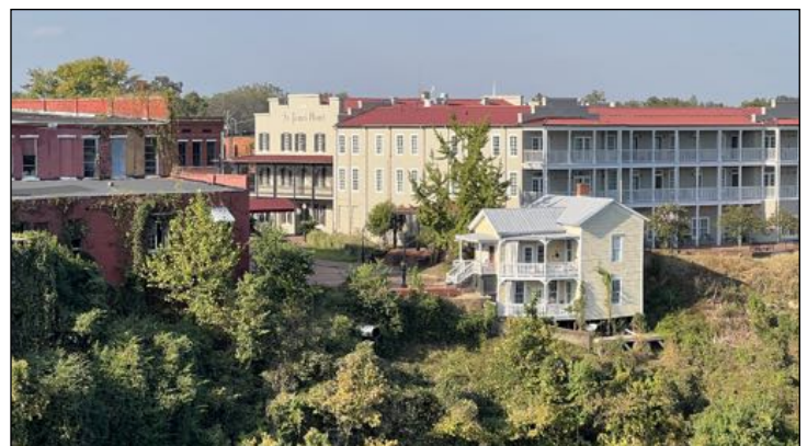
Figure 3.16 : Waterfront Open Space Condition
