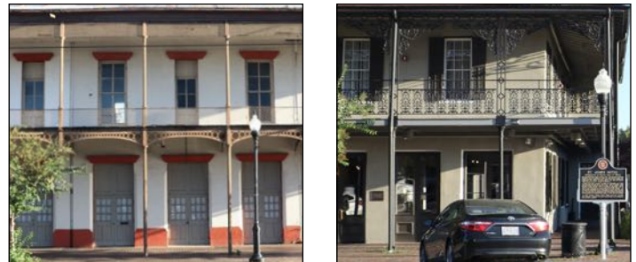
Figure 3.20: Porches of Downtown Building
