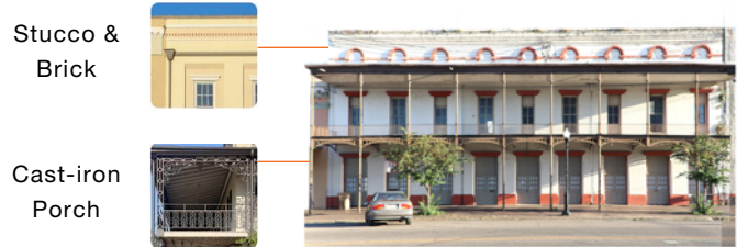
Figure 2.43 : Water Avenue Italianate Features
