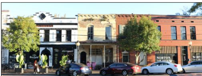
Figure 2.28 : South Side of Water Avenue
