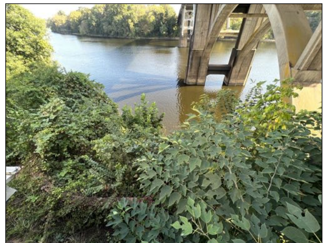
Figure 4.25 : Existing conditions of riverfront beneath bridge in Songs of Selma Park
