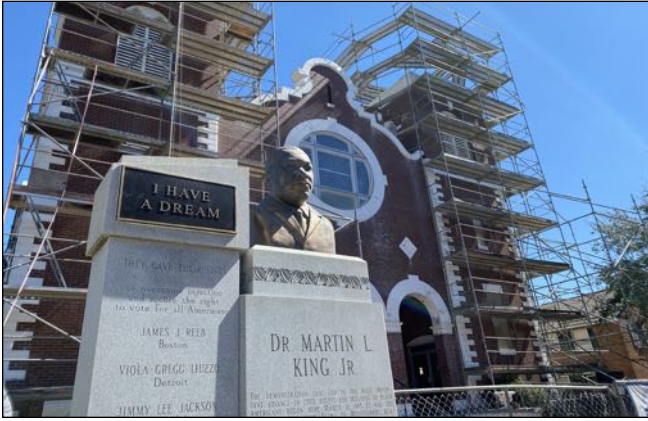
Figure 2.59 : Ongoing renovations at Brown Chapel AME Church.
