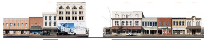
Figure 2.42 : Broad Street Existing Buildings, Comparing 1887 with 2022
