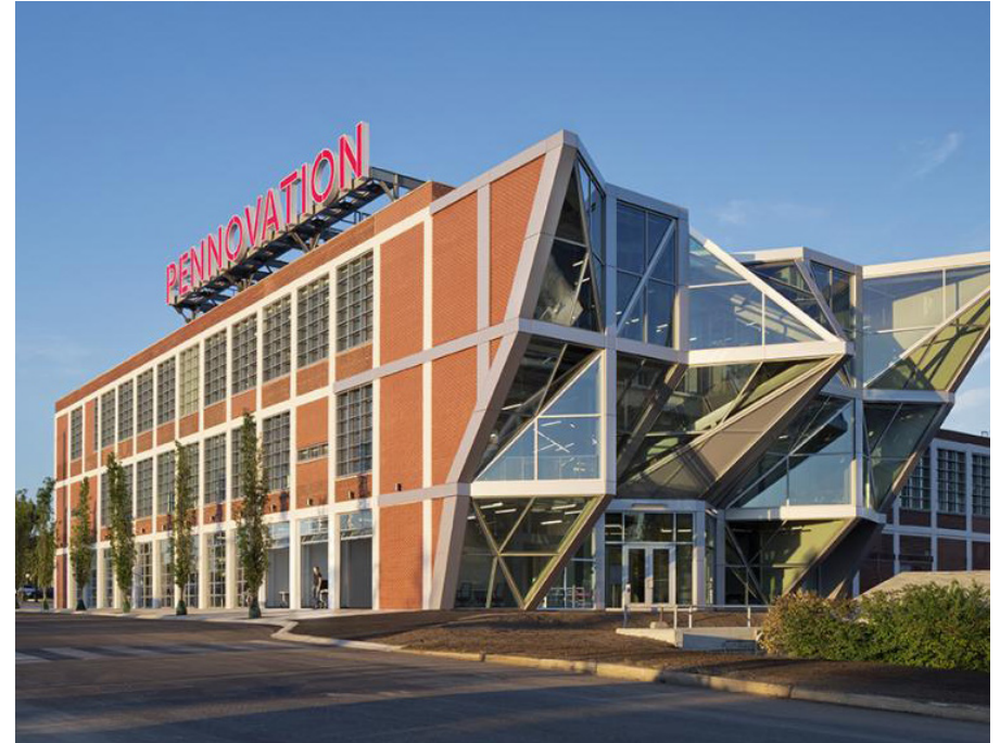
Image: Pennovation Center, University of Pennsylvania)
