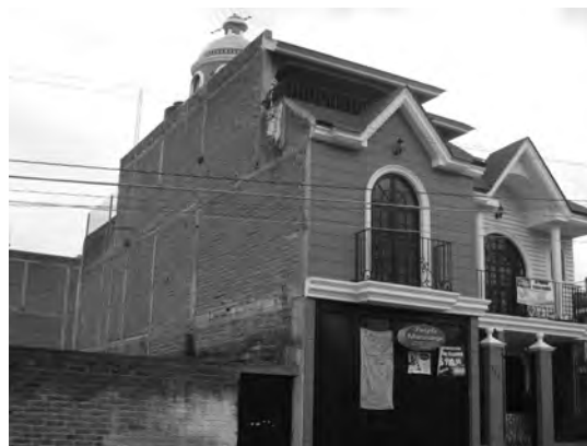
Figure 9. The façade of this house, built in Jalisco by a family living in Texas, mimics wooden siding using stucco and concrete. Note the side of this house is unadorned even though there are no plans to build an adjacent house. Photograph by author.
