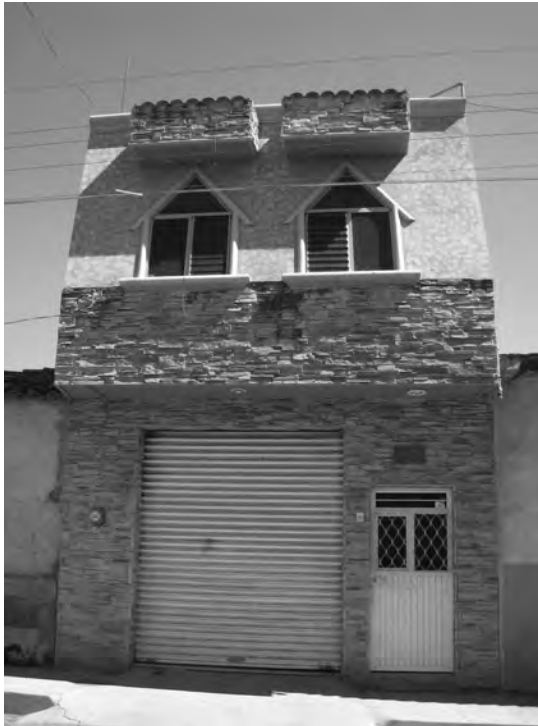
Figure 10. Note the representation of pitched-roof dormers in the ornate window frames and the innovative, cantilevered shed-roof features above the windows. Photograph by author.
