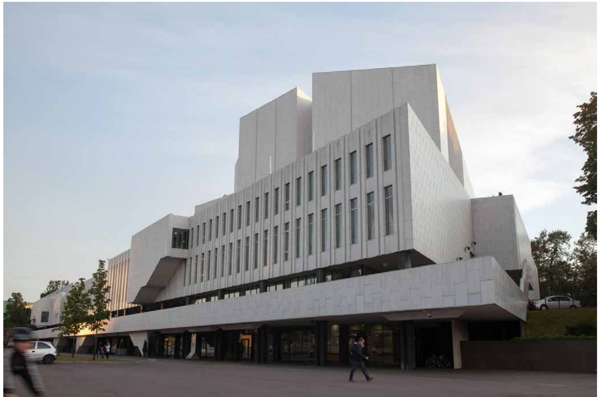
Figure 1. Finlandia Hall. by Mari on 28th September 2019. (Source: Photo Credit: Athenaeum of Philadelphia, Lawrence Williams Inc. Collection, Local ID#:77133-A).
