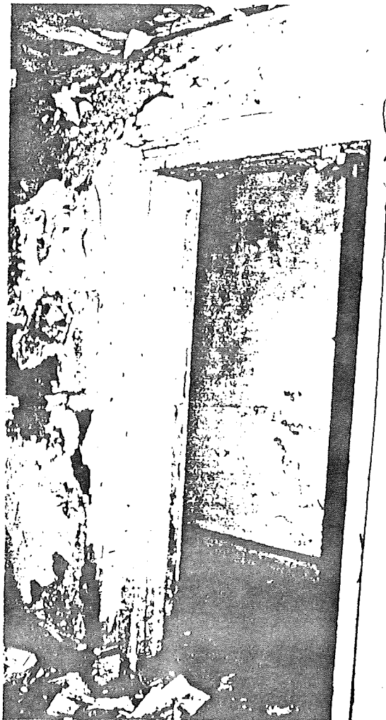
16. Treating House, first floor, office, southeast addition, southeast corner. There is extensive water damage in the southeast corner caused by a leaking roof and damaged gutters on this one-story addition. Neg. 3-12.
