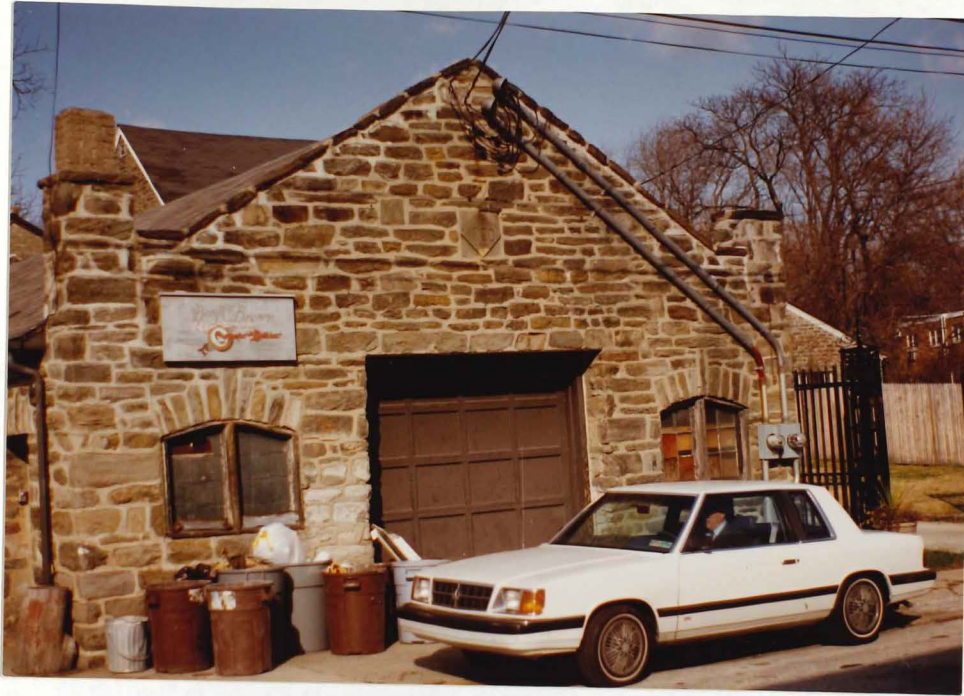
"Benj. C. Blaw, Carpenter" (former garage) - 15 E. Maryland Ave., Chestnut Hill
