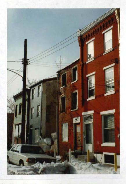
Figure 6.1.a. The red building on the right side of the photo is rated Condition One: Very few to no signs of deterioration. The small red building to its left is rated Condition Three: Severely deteriorated.
