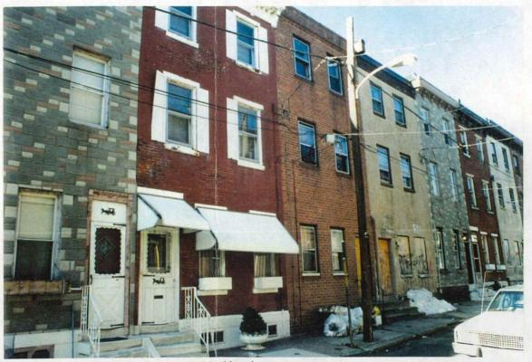
Photo 4. A: Awnings added, shutters in original location.C: Peeling paint, basement windows boarded up, cornice missing.
