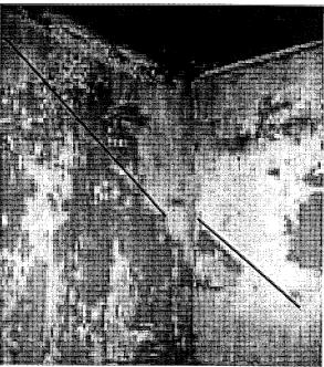
Figure 4.2. Diagonal lines on the planter walks of room 20th indicate evidence of a previously existing stair
