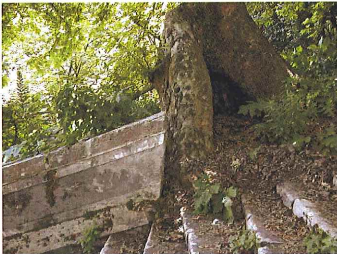
View to the south indicating the location where the railing wall was intentionally cut to allow for the growth of the historic plane trees. (UPenn 2002)
