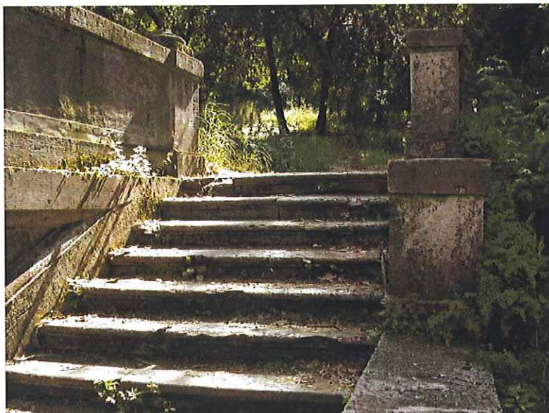
Cracks in the stone, as well as invasive vegetation are clearly evident on the South Fountain Stair. (UPenn 2002)
