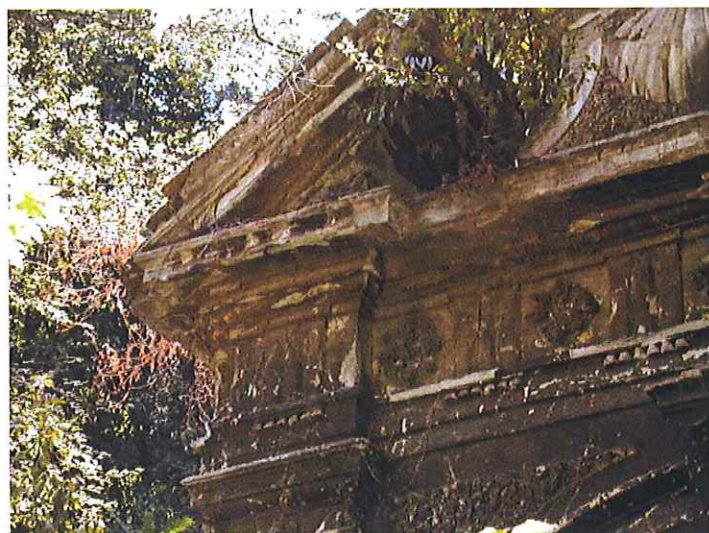
Conditions found on the Nicchione include loss of surface finish as well as carbon deposits associated with fires created inside the apse. (UPenn 2002)
