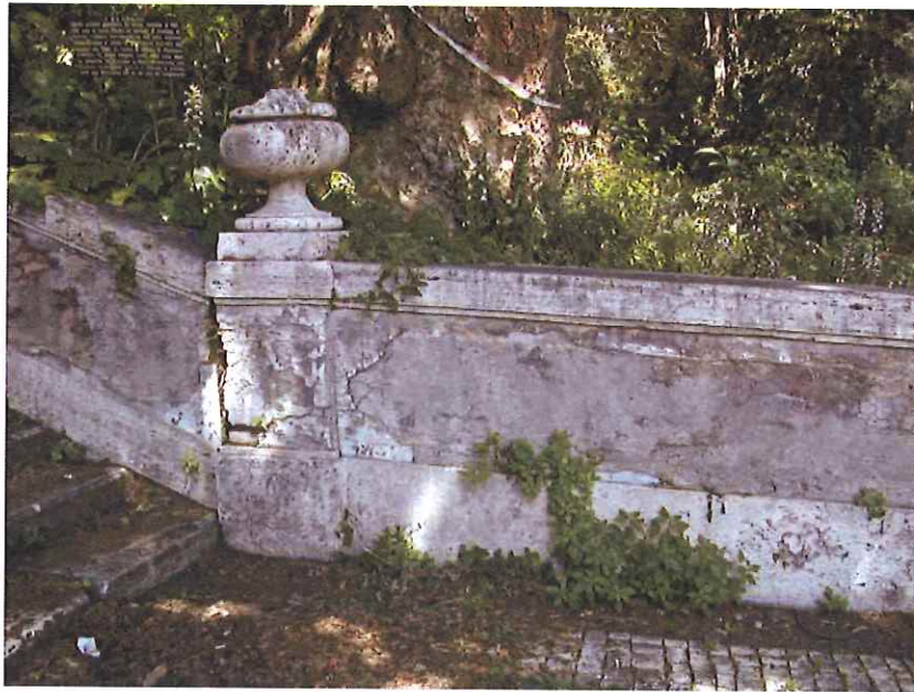
Looking north at the railing wall of the second landing. Note the invasive vegetation. (UPenn 2002)
