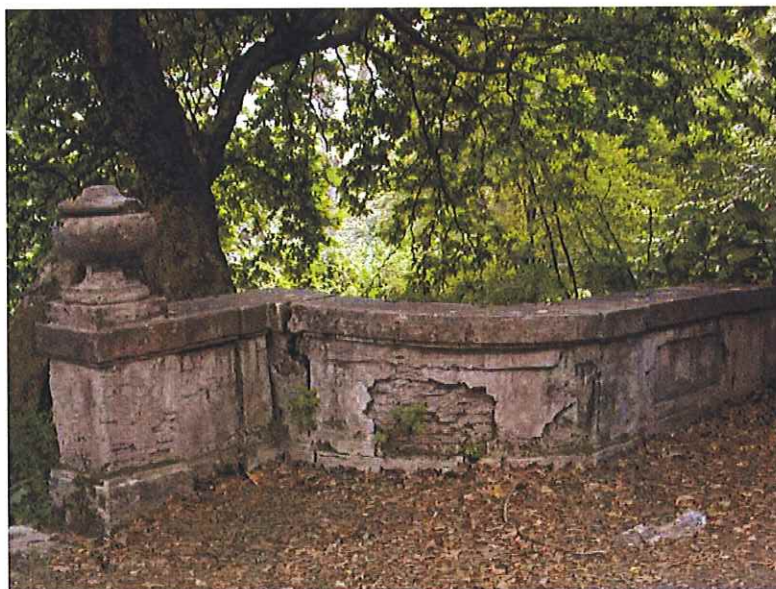
The railing wall of the north landing-2 showing extensive damage to the surface finish. (UPenn 2002)
