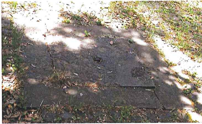
A manhole cover located in the second landing which provides access to the sub-grade vault. (UPenn 2002)
