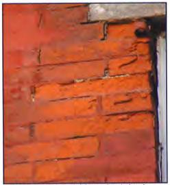
brick damage: these bricks are located under a leaky gutter, the increased moisture has caused the brick faces to crack off (UPenn 2003)
