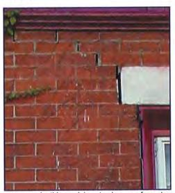
stress crack: this crack is not only a way for water to get into the building, it can also be a sign of more serious structural damage (UPenn 2003)
