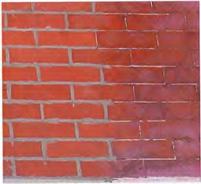
improper re-pointing: the new mortar on the left is a different size, color and composition than the original mortar on the right (UPenn 2003)
