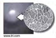
Crazing is the formation of fine cracks throughout a painted surface which is not yet peeling. This occurs when there are many paint layers on a surface which are not able to expand and contract during varying temperatures and humidity. Sanding by hand or with an electric sander will expose a sound layer of paint, which can then be repainted.
