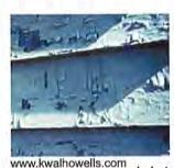
Peeling is usually due to moisture which collects behind the paint in the wood or masonry causing the paint to pop off. It is imperative to locate and repair the source of water infiltration. This will help prevent future disintegration of paint layers and also protect the material underneath the paint from deterioration. The sources may be clogged gutters, decayed flashing, cracks in the siding, open
