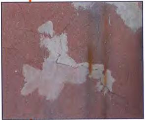
An example of an inappropriate stucco repair: the replacement material is dissimilar to the existing stucco (UPenn 2003)
