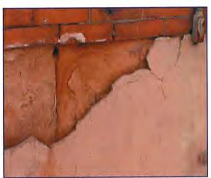
An example of damage caused by moisture: this stucco and the stone behind it has been damaged by water trapped behind the stucco (UPenn 2003)
