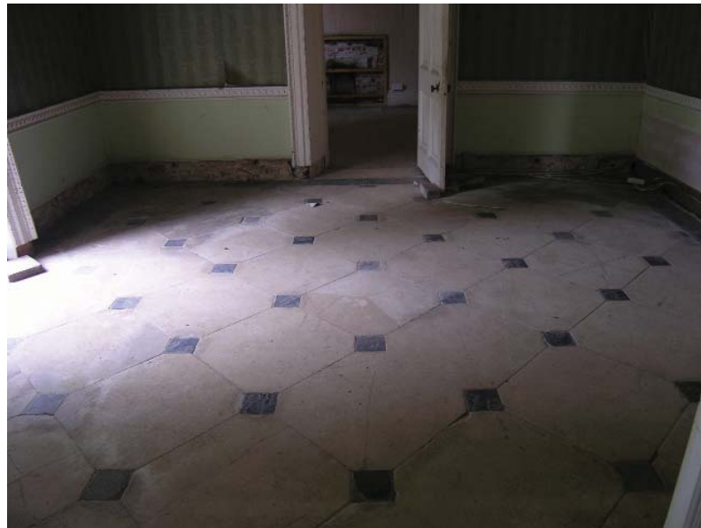
Figure 26: Outer Hall: View looking down at floor, which consists of large square Portland stone tiles, laid on the diagonal, with small square black slate tiles set at the corners. Source: University of Pennsylvania.
