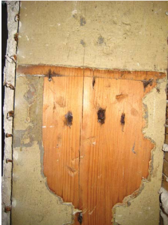
Figure II.10: View from the west of the painted profile at the top of the balustrade on the east jamb board of the balustraded opening. The paint evidence indicates that the carved chair rail, installed at the time the south wall was plastered, was also applied to the Inner Hall side of the balustrade hand rail since it overlays earlier paint. The fact that a similar chair rail profile exists on the Outer Hall side of the hand rail with no evidence of earlier paint may indicate that the chair rail was also used in conjunction with the original Outer Hall paneled walls. Source: University of Pennsylvania.
