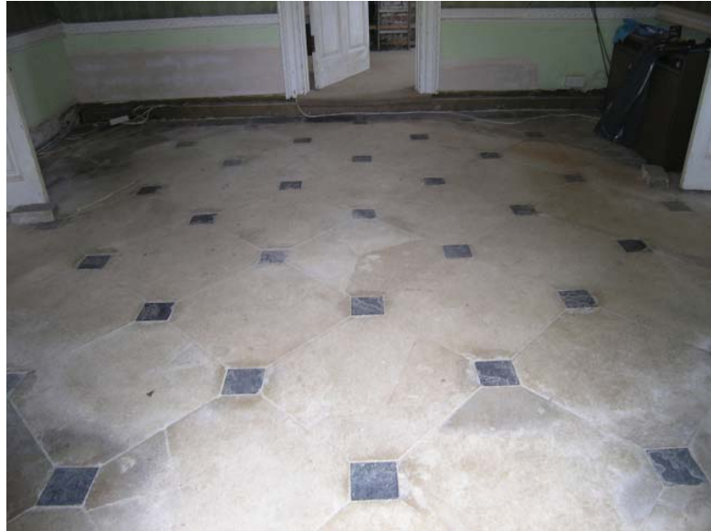
Figure I.24: View from the south of the original masonry floor in the Outer Hall. Source: University of Pennsylvania.
