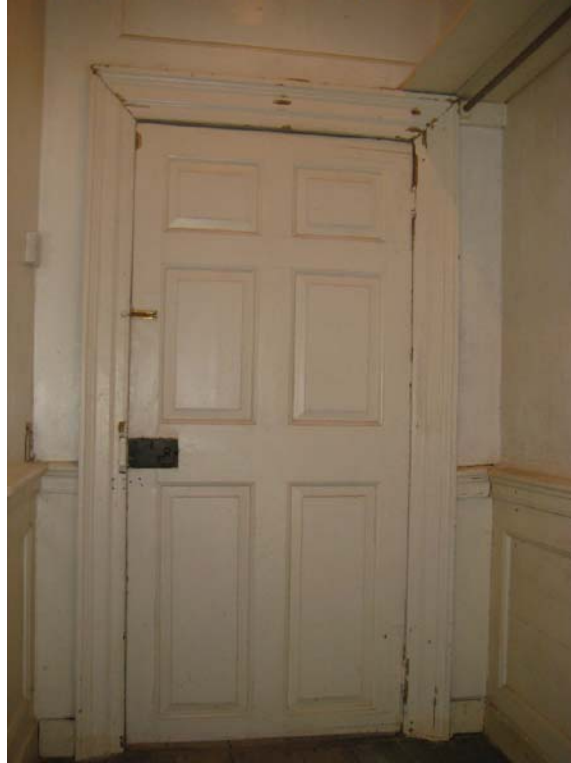
Figure 40: Corridor: View looking south at door and simple woodwork in the form of a cornice, chair rail and wainscoting. Source: University of Pennsylvania.
