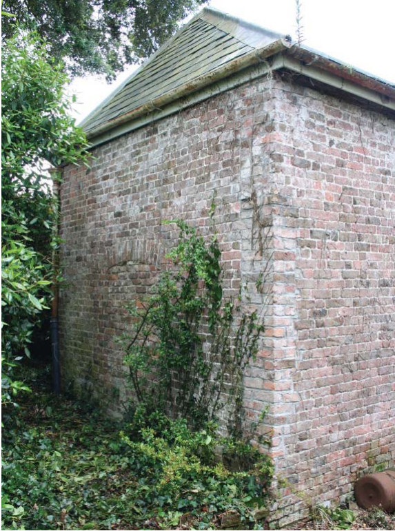
Figure I.1: East wall of French Garden house. The butt joint between the east and rear wall is clearly visible - an indication that the side was added onto the rear wall. Source: University of Pennsylvania.
