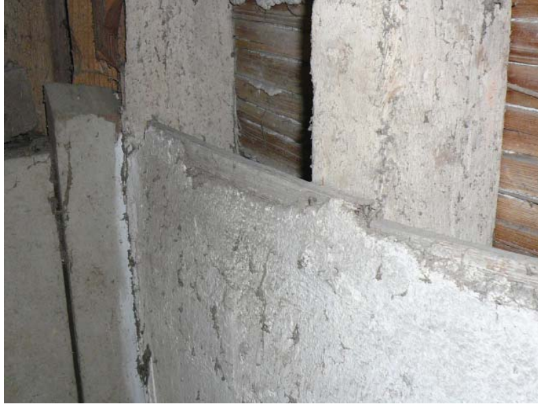
Figure III.15: The top of the plaster around the rear of the apse appears finished, as the edge is smoothed over the edge of the apse. Likewise, there are no lath nail holes above the plaster, and the studs are painted. Source: University of Pennsylvania.
