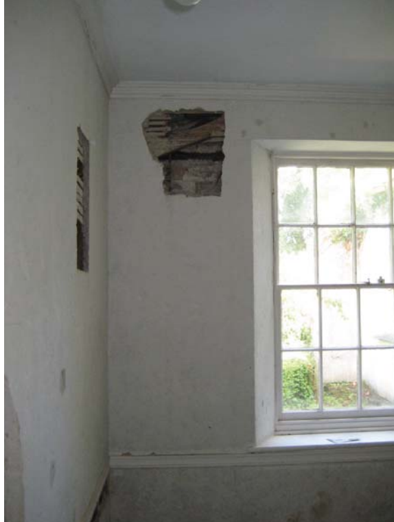
Figure II.17: View from the west wall of the bathing room showing space for a wood nailer in the masonry at chair rail level. Source: University of Pennsylvania.
