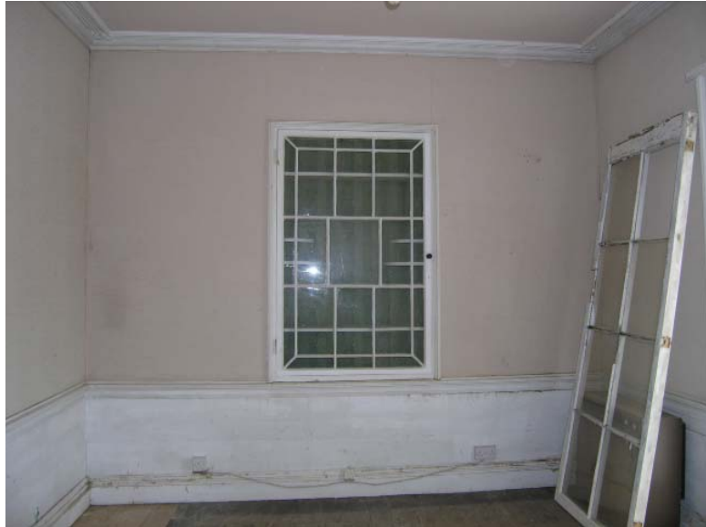
Figure 29: East Room: View looking east at built-in cabinet set above the wood wainscot. Source: University of Pennsylvania.
