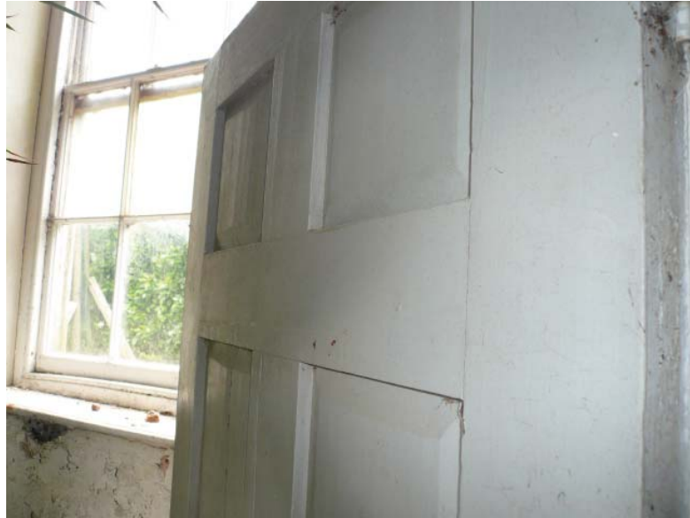
Figure III.7: The doors to the back room all appear to be hand-planed. Note the uneven surface, evidence of the hand crafting. Source: University of Pennsylvania.
