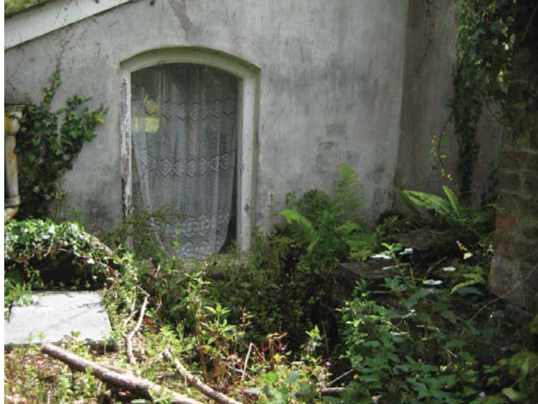
Figure V.1: View from the west of the exterior west wall of the Rear Room. The previous door in this location was converted to a window. Source: University of Pennsylvania.
