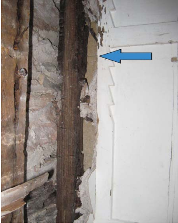
Figure I.4: View from the south of the butt joint between the north wall of the Bathing Room (at the left) and the west façade of the original building (at the right). A portion of the original scored stucco exterior finish on the west façade has survived in this joint. Source: University of Pennsylvania.
