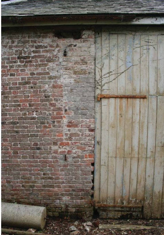
Figure III.1: The brick infill in the openings of the original window are visible to the left of the rear door. The insertion of the rear doors re-quired the removal of the window. Source: University of Pennsylvania.
