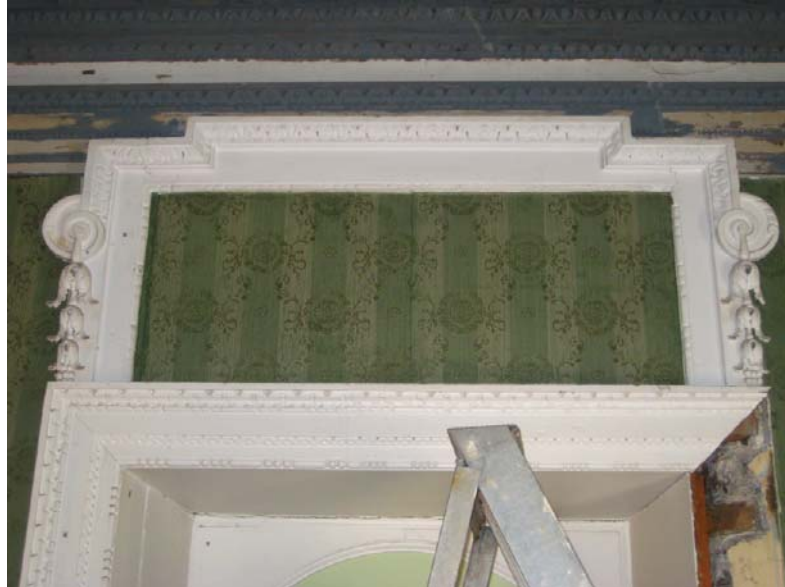
Figure I.18: View from the west of the top portion of the interior frame for the original east window. Source: University of Pennsylvania.
