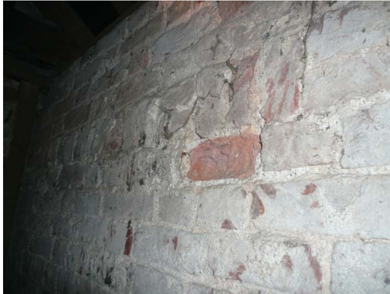
Figure II.2: These courses of brick, the bottom row containing the broken faced brick and the course above it containing the bricks laid on edge, indicate the section of the wall that was infilled. Source: University of Pennsylvania.
