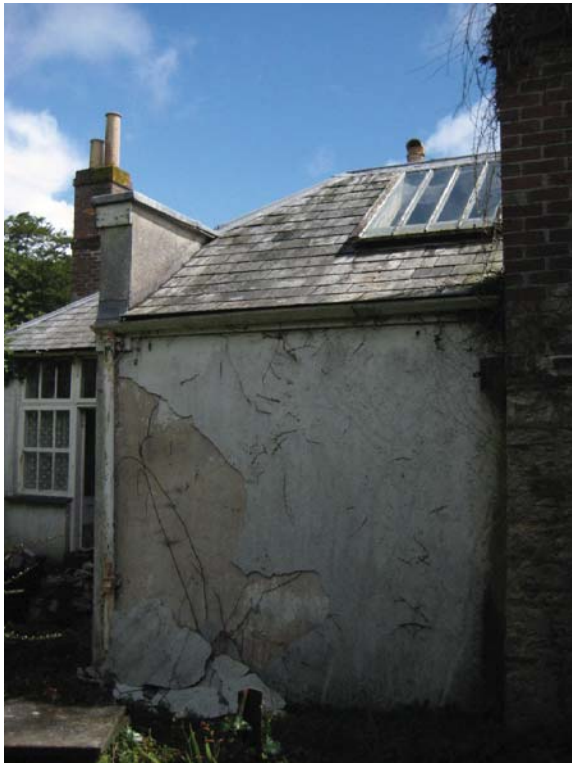
Figure II.16: View from the west showing the later-hipped roof over the bathing room and the north parapet wall which was original to the bathing room. Source: University of Pennsylvania.
