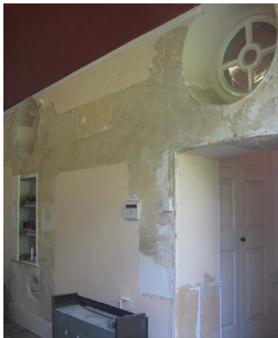
Figure I.1: View of the original north façade from the northwest (in current Kitchen). Original clerestory windows appear at the top; original scored stucco exterior finish revealed under modern wall paper. Source: University of Pennsylvania.
