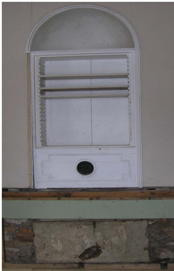
Figure III.12: View from the east of the wainscot in the northeast corner of the East Room, indicating the advanced deterioration that exists. The black tar paper was installed in the recent past to combat the effect of migrating moisture on the wood elements of the room. The exterior grade is approximately 16 inches above the floor level, exacerbating the situation. Source: University of Pennsylvania.
