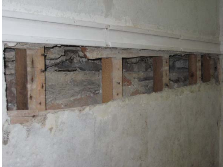
Figure II.17: View from the west wall of the bathing room showing space for a wood nailer in the masonry at chair rail level. Source: University of Pennsylvania.
