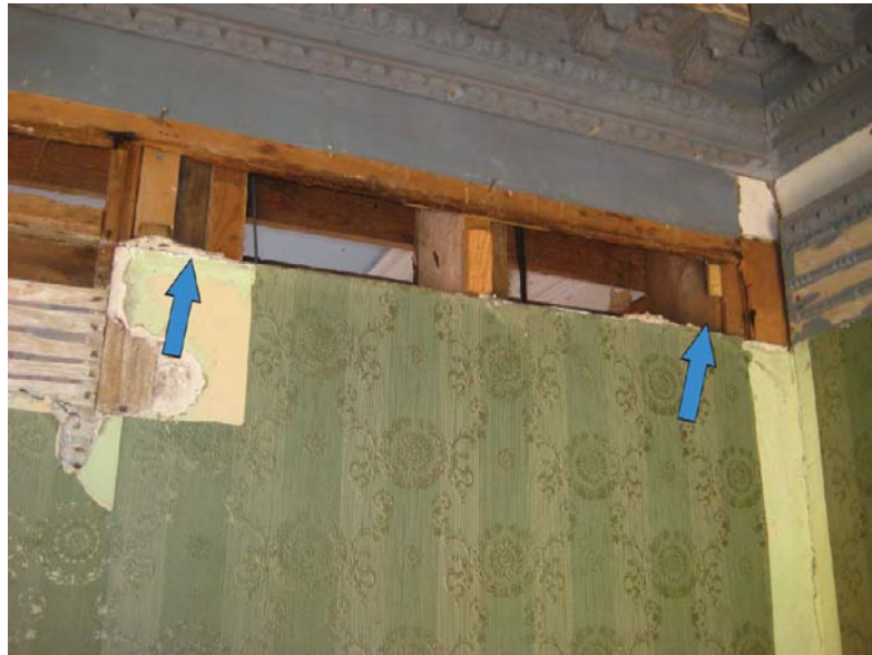
Figure I.12: View from the south in the location of the eastern jamb of the original balustraded opening. The original stud has no evidence of lath and plaster. Source: University of Pennsylvania.
