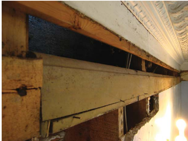
Figure I.33: View from the east of the surviving rail of original paneling that existed on the south wall of the Inner Hall above and around the balustraded opening. Source: University of Pennsylvania.
