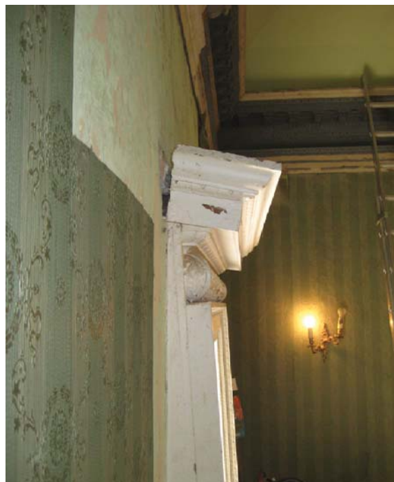
Figure I.21: View from the east of the cornice for the south interior door surround. The cornice was pulled away from the wall after the paneling was removed to facilitate plastering of the south wall. Source: University of Pennsylvania.
