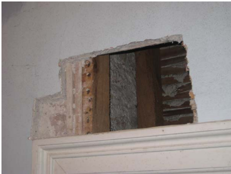
Figure II.12: View from the east looking into the void above the doorway in the west wall to the Bathing Room. This section of wall was replastered, perhaps in Phase III. Source: University of Pennsylvania.
