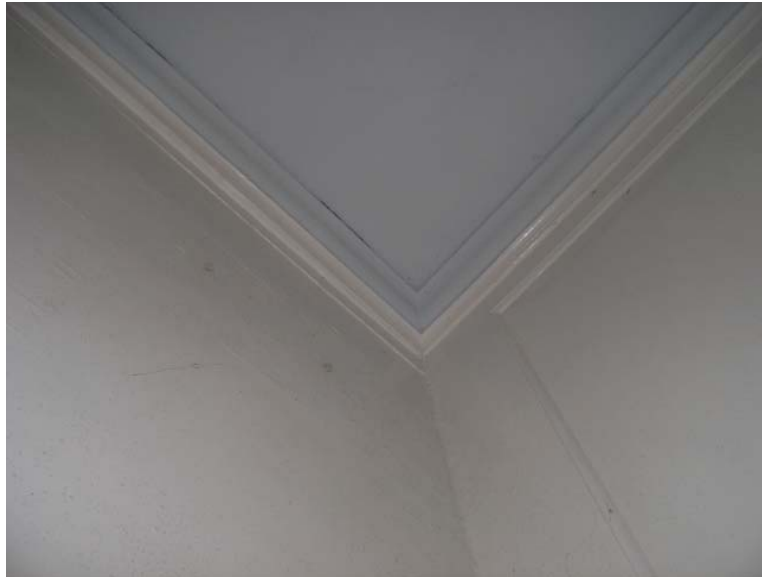
Figure I.37: View looking up at the original cornice molding in the Privy which is similar in dimension to the evidence found on the north paneled wall of the Inner Hall. Source: University of Pennsylvania.
