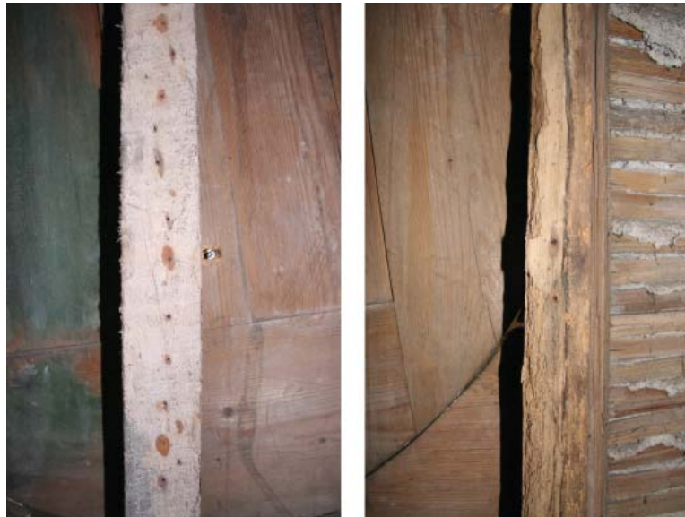
Figure III.14: The plaster on the rear of the apse never continued around the entire arc. Visible here on the left are lath nail holes in a stud about halfway around the arc. The adjacent stud, on the right, is clean. Source: University of Pennsylvania.
