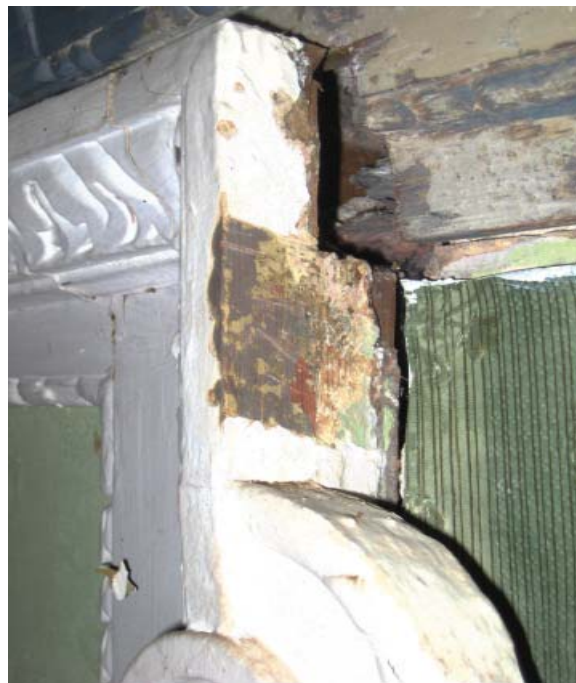
Figure I.19: View from the south west of the corner of the original east window frame that was designed to be partially recessed in the original wood paneling. The portion of the frame to the right of the red primer/grey paint line was recessed. Source: University of Pennsylvania.
