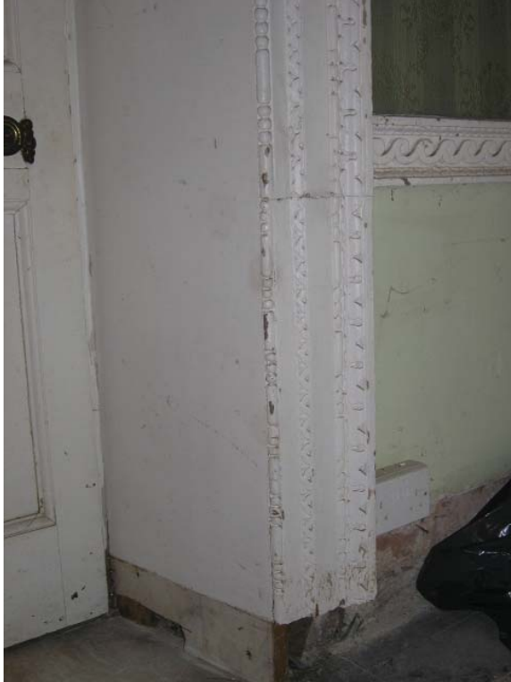
Figure III.1: View from the west of the lower portion of the door frame leading to the east Room. New pieces were added to the bottoms of the east and west door frames to reconfigure them as doorways. Source: University of Pennsylvania.
