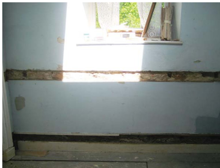
Figure II.20: View from the west at the east wall of the Inner Hall. Removal of the existing chair rail exposed the stone masonry which contained no seams or other evidence of a doorway connecting with a wing to the east. Source: University of Pennsylvania.
