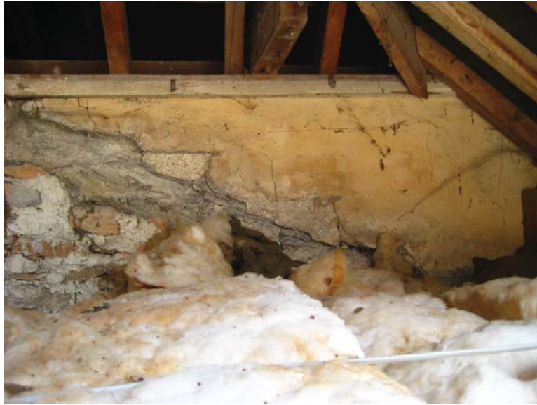
Figure II.15: View from the north in the attic space above the ceiling of the Bathing Room. The evidence of the original sloping roof is a mirror image of photo II.14. The parapet wall above the sloping roof is also covered in stucco. Source: University of Pennsylvania.
