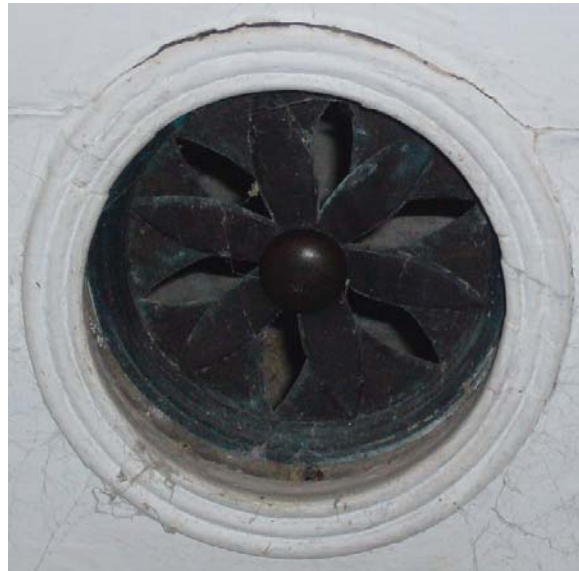
Figure III.14: View of the ventilation device centered in the base of the north cabinet. This device, and the stone slabs below, may be related to the fireplace feature on the northern side of this stone wall that was retro-fitted from its original use in the earlier wing to the north. Source: University of Pennsylvania.
