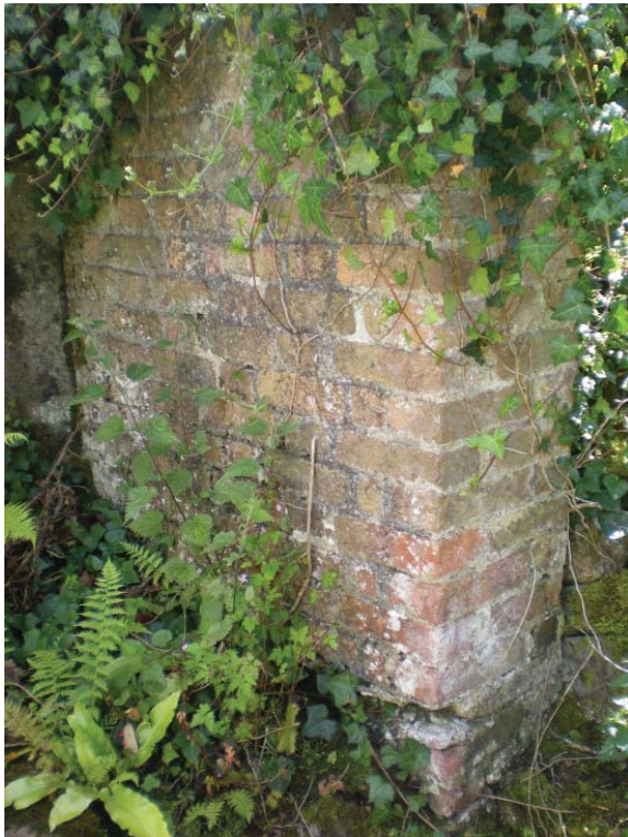
Figure IV.2: View of a portion of Flemish bond brick wall incorporated in the rear building. The bricks in this wall are identical to those found in the north wall of the French Garden House. Source: University of Pennsylvania.
