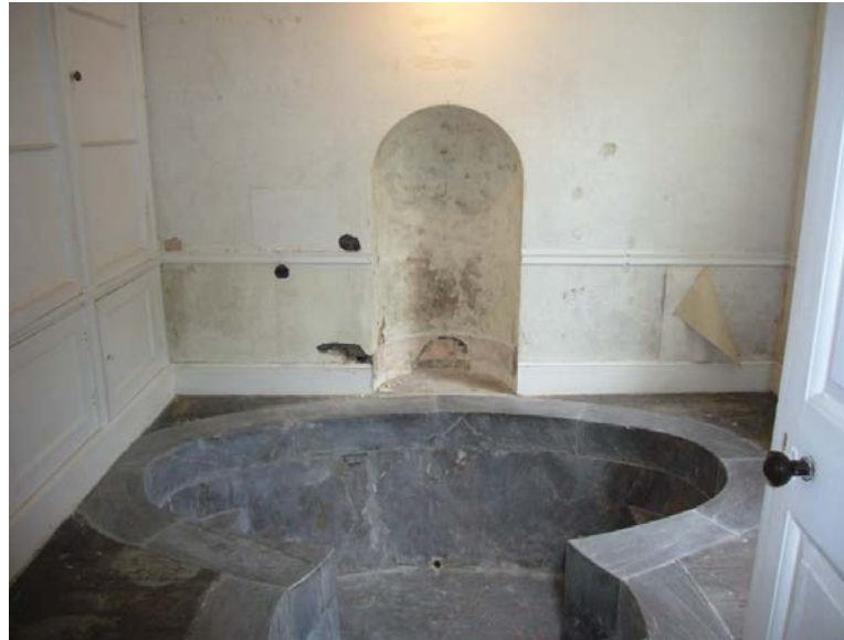
Figure III.6: View from the east of the west wall of the Bathing Room. The cabinets to the left (south) mask the alcove of the West Room which encroaches on the Bathing Room. The niche at the center of the west wall accommodated the bronze dolphin spouts that delivered hot and cold water to the tub. The date of installation of this niche is not known, although it is likely concurrent with the Phase III renovations. Source: University of Pennsylvania.
