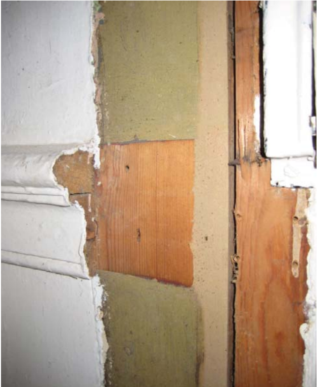
Figure I.39: Profile of the original chair rail existing in the Privy. Source: University of Pennsylvania.
