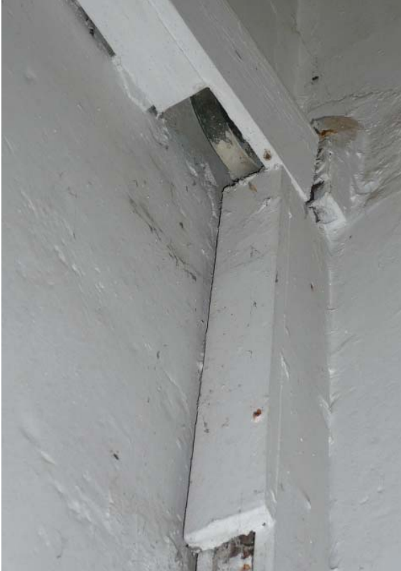
Figure III.3: The pulleys within the track system appear bronze and are thought to be original to the room. Source: University of Pennsylvania.
