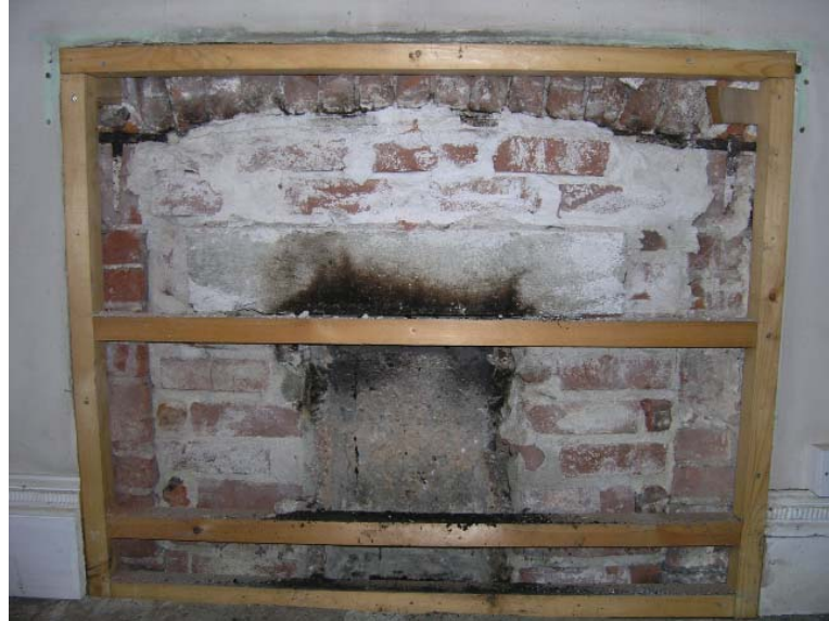
Figure III.16: View looking west at the fireplace centered in the west wall of the West Room. This feature has not been further investigated, but apparently incorporates a rather unique narrow flue imbedded in the west wall and rising diagonally to a chimney stack incorporated in the west wall of the Bathing Room. Source: University of Pennsylvania.
