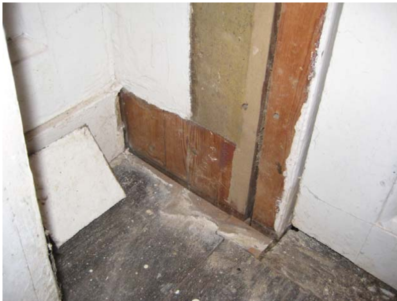
Figure 1.50: View from the northwest at the intersection of the east Privy wall with the wood partition to the west of the chimney mass. The original baseboard was removed to reveal original paint lines and evidence of modifications in the doorway width and surround. Source: University of Pennsylvania.
