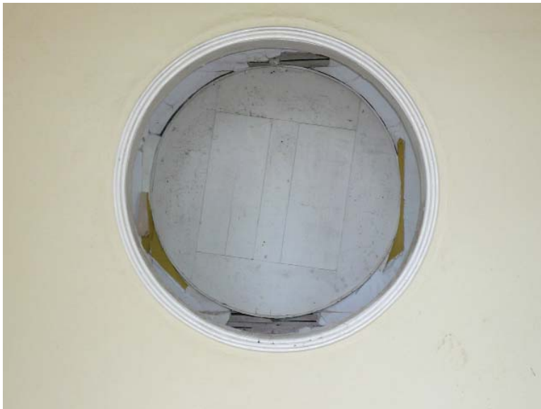
Figure III.2: The circular frame in the apse is constructed in the tradi-tional way one would build a large circle out of wood. A small lip around the edge of the front of the circle indicates that it was intended to hold something. Source: University of Pennsylvania.
