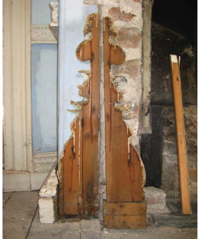
Figure I.42: View of the carved console applied to the west stile of the wood chimney breast. The console has been removed in this image and is laid back to the right. The paint evidence indicates that the console is original to this location. Source: University of Pennsylvania.
