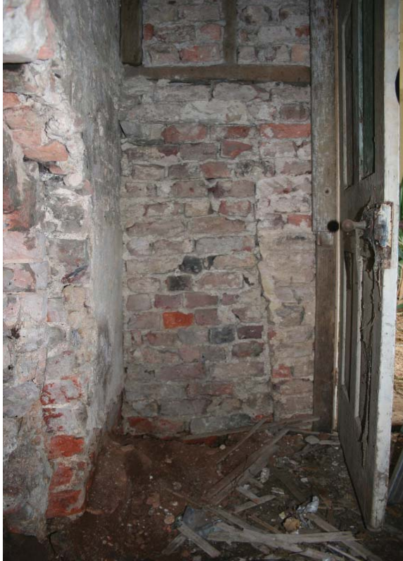
Figure III.13: Behind the east door in the back room is the visible infill of the flue. The partition wall was clearly built around the flue, and the wall was infilled at a later date. Source: University of Pennsylvania.
