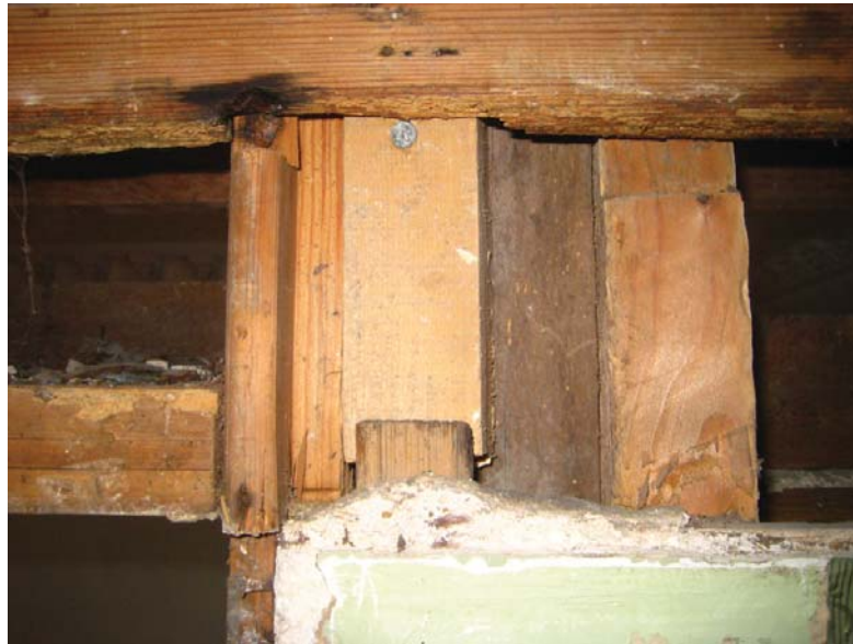
Figure I.14: View from the south of the original eastern jamb board showing the rebate to receive the wood paneling (now missing) and the \frac{3}{4} " edge bead. Source: University of Pennsylvania
