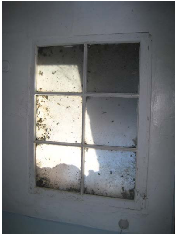
Figure V.7: View looking up at the glazed sash in the ceiling of the Modern Bathroom that borrows light from a skylight in the roof. Source: University of Pennsylvania.
