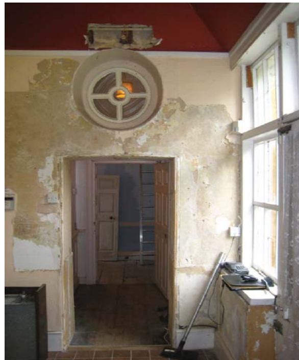
Figure 46: Kitchen: View looking southwest at the south wall and Corridor beyond. Source: University of Pennsylvania.
