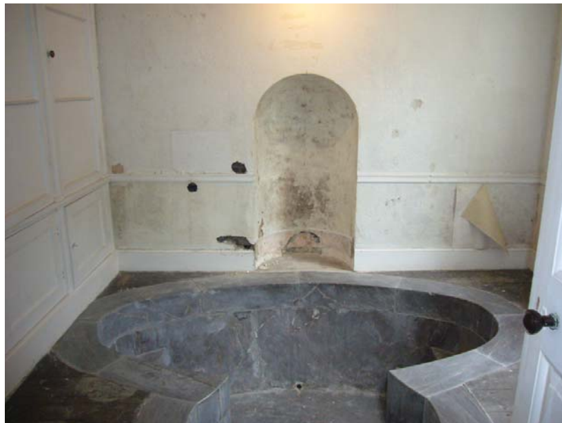
Figure 41: Bathing Room: View looking west at bathtub and west wall niche. Source: University of Pennsylvania.
