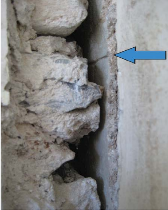
Figure I.6: View from the north in the Toilet of the butt joint between the south wall of the Toilet (at the left) and the east façade of the original building (at the right). A portion of the original scored stucco exterior finish on the east façade has survived in this joint. Source: University of Pennsylvania
