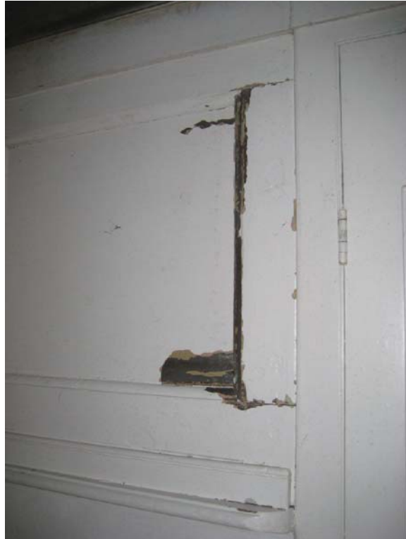
Figure I.47: View from the west of the wood paneled wainscot in the Privy. The stile to the left has been moved and refitted to accommodate the installation of a pair of closet doors on the east wall. Source: University of Pennsylvania.
