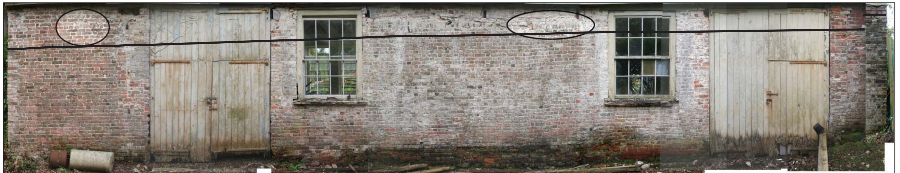
Photo mosaic of entire rear wall of French Garden house. The black line highlights the original height of the wall, and the ovals highlight areas where the coursing was increased to level the wall. Source: University of Pennsylvania.
