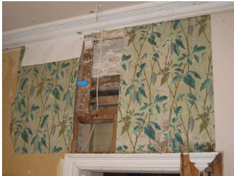
Figure I.17: View from the east in the East Room showing the original wood lintel above the east window in the original building. Source: University of Pennsylvania.
