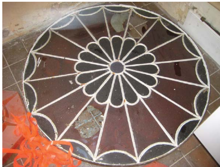
Figure V.9: View of removed round colored-glass skylight from Outer Hall covered ceiling. Source: University of Pennsylvania.
