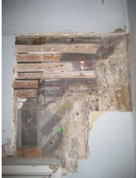
Figure II.8: View from the south of the wood paneled wall above the door in the north wall to the Storage/Dressing Area. Evidence of the previous position of a decorative overdoor is clearly discernable in the painted surface. Source: University of Pennsylvania.
