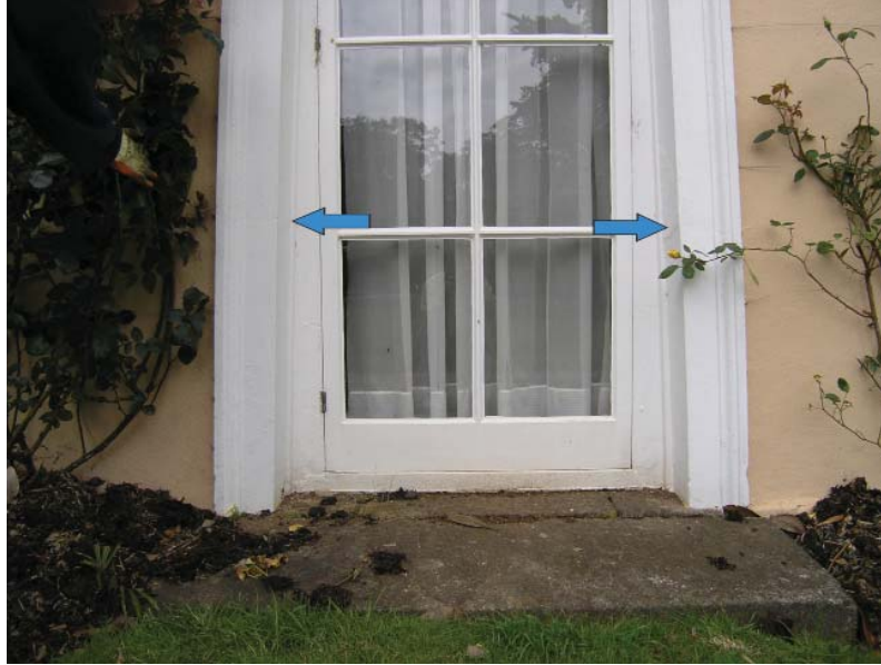
Figure III.15: View from the south of the south doorway in the East Room. The seams in the stone frames suggest that this feature was originally a window as depicted in the 1860-65 engraving. Source: University of Pennsylvania.
