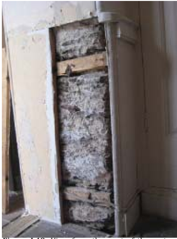
Figure 1.49: View from the west of the eastern jamb of the doorway from the Privy to the Kitchen. The stonework has been rebuilt to accommodate the wider opening. Source: University of Pennsylvania.
