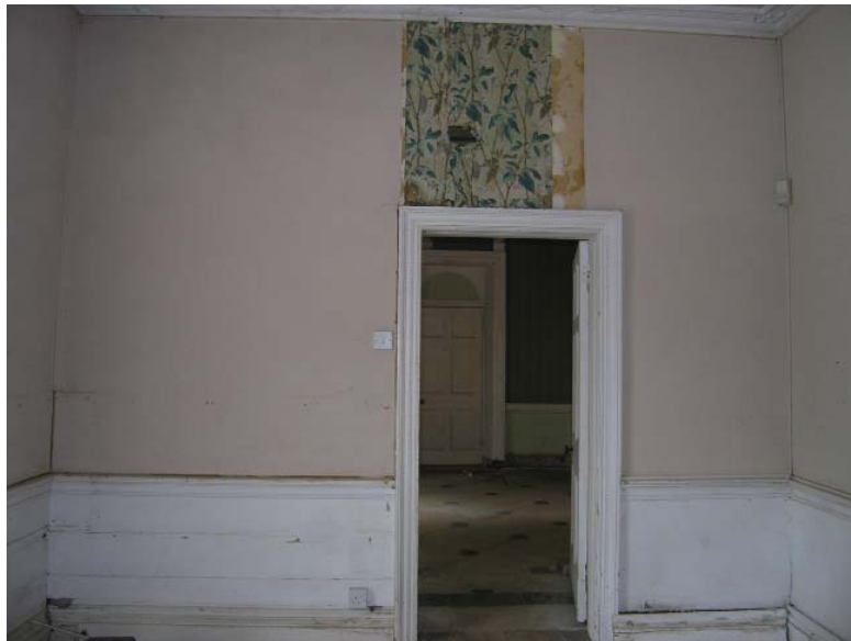
Figure 30: East Room: View looking west at the wood chair rail with wainscot below. The Outer Hall is beyond the door. Source: University of Pennsylvania.
