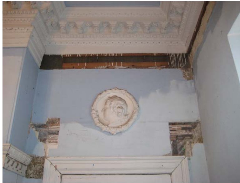
Figure II.7: View from the south of the upper portion of the north wall to the east of the chimney mass. Sections of the architrave of the cornice were removed for investigation, and the paint evidence and installation methodology supports the Phase II chronology. Source: University of Pennsylvania.
