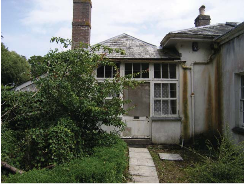
Figure 20: West Elevation: View showing series of intersecting slate hipped roofs from the west elevation. Source: University of Pennsylvania.
