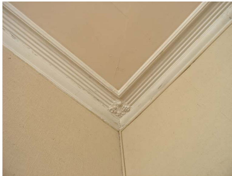
Figure III.11: View of the original plaster cornice in the northeast corner of the East Room. Source: University of Pennsylvania.
