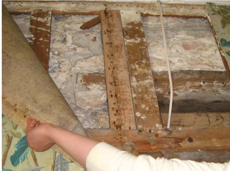
Figure III.8: View from the east of the west wall above the doorway leading to the Outer Hall. Fragments of original stucco exterior finish remain on the east face of the stone wall. The system of furring strips to which the wallpaper was applied is visible. The hand-hewn wood lintel behind the furring strips relates to the original east window in the original building. Source: University of Pennsylvania.
