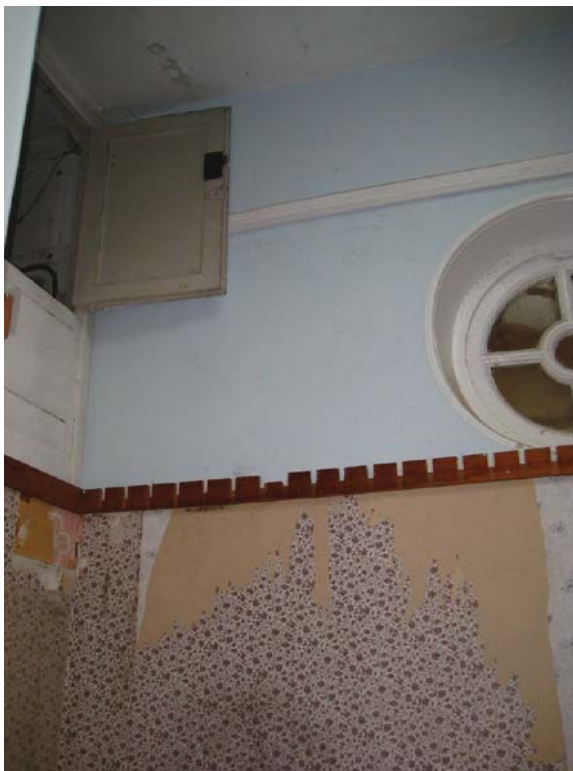
Figure 38: Modern Bathroom: View looking northwest at the upper portion of the west wall with cabinet access to mechanical closet. Also looking at the north wall's high circular window above the bathtub. Source: University of Pennsylvania.
