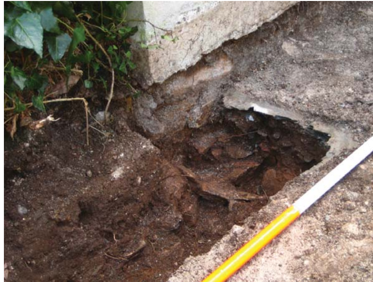
Figure II.19: View from the northeast showing the northeast corner of the existing East Room. Archeological excavations, concurrent with the compilation of this report, revealed the existence of a stone foundation wall integral with the north stone wall of the East Room and extending to the north. This evidence supports the hypothesis that an eastern wing, symmetrical with the Bathing Room wing, existed prior to the construction of the East Room. Source: University of Pennsylvania.
