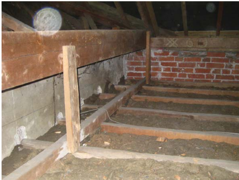
Figure I.3: View of the original west façade from the northwest (in the attic space above the West Room ceiling). The original scored stucco exterior finish is largely intact. Source: University of Pennsylvania.
