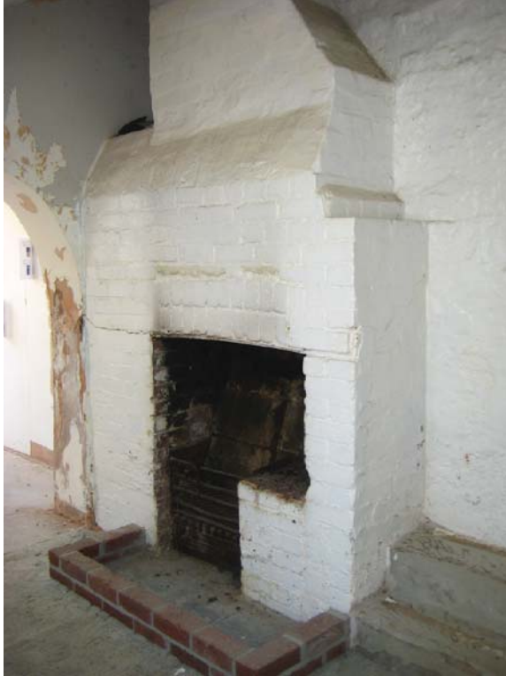
Figure IV.3: View from the northwest of the fireplace on the south wall of the Rear Room. Its purpose and function relative to the English Garden House are not known. Source: University of Pennsylvania.
