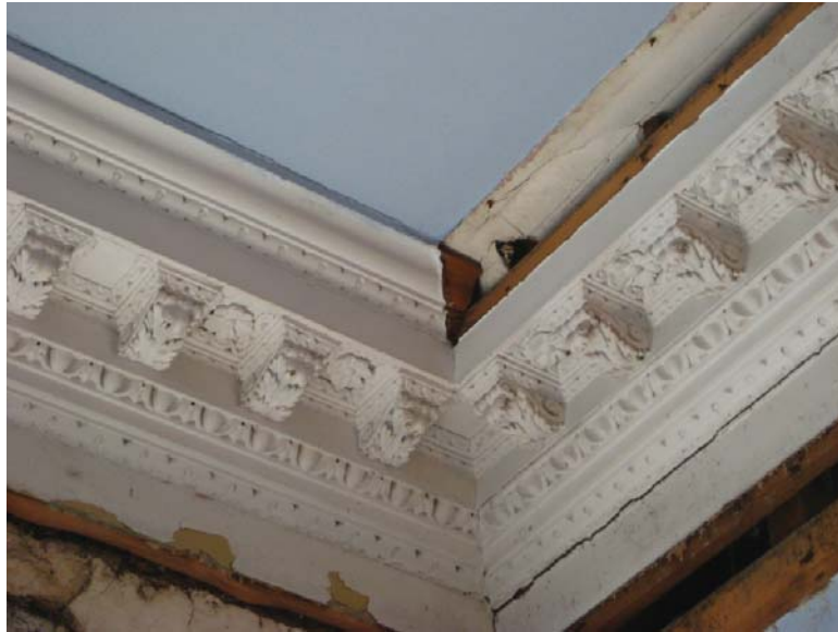
Figure II.6: View from the northwest of the southeast corner of the cornice in the Inner Hall. The design, detailing and installation of the cornice indicate that it was intended specifically for this room and not recycled from another location. The coped crown moulding is supportive of this point. Source: University of Pennsylvania.
