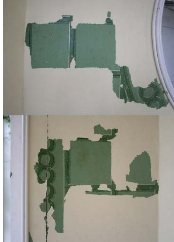
Figure III.4: The circular pattern found on the walls outlines the elements with trim in the room. The rest of the walls are decorated with a repeating square pattern, the texture visible through the top layer of paint. Source: University of Pennsylvania.
