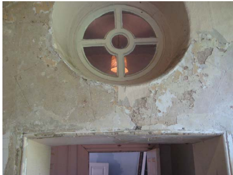
Figure I.9: View from the north of the original scored stucco below the circular window in the Privy. Source: University of Pennsylvania.
