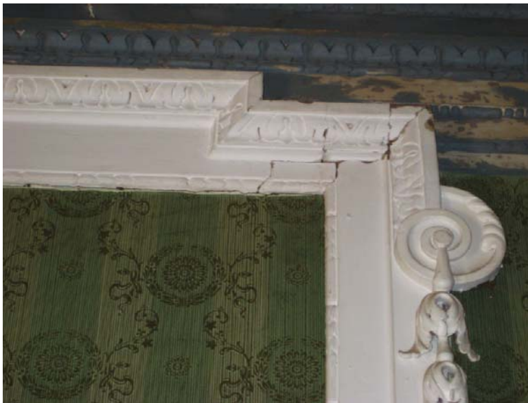
Figure III.2: View from the west of the overdoor at the doorway to the East Room. As previously mentioned, this overdoor is the top portion of the original frame for the east window in the Outer Hall. It was salvaged and used as a decorative element in Phase II when the paneling was removed, the walls were plastered and the window openings fitted with new carved frames. When the doorways were added to access the new East and West Rooms, the Phase I and Phase II frames were widened to fit the wider door openings. The 3 inch insertion at the top edge of this frame is evident. A symmetrical 3 inch piece was also added at the other side of the frame. Source: University of Pennsylvania.
