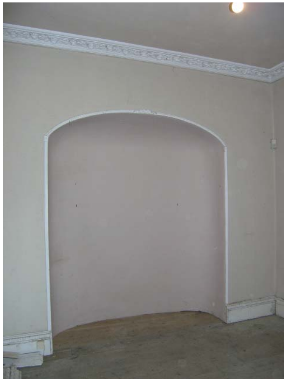
Figure III.17: View from the south west of the alcove in the north wall of the West Room. This feature is original to the construction of the room. Source: University of Pennsylvania.
