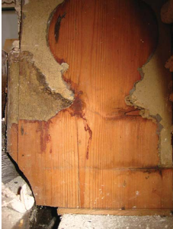
Figure II.11: View from the west of the painted profile at the bottom of the ballustrade on the east jamb board of the ballustraded opening. The paint evidence indicates that the baseboard present in the inner hall once turned the corner into the ballustraded opening. The outline overlays earlier paint indicating that this baseboard was installed in Phase II. Source: University of Pennsylvania.
