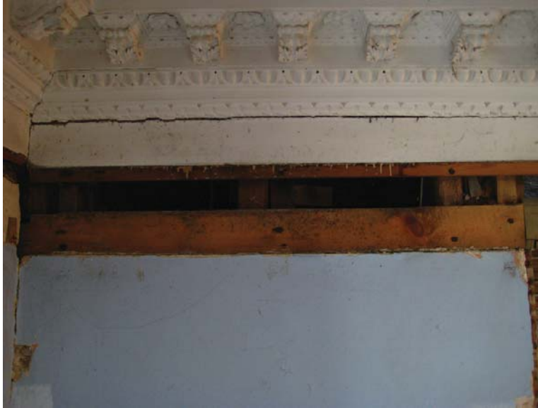
Figure II.9: View from the north of the cornice at the east end of the south partition wall, east of the original balustraded opening. The white plaster at the far left of this image ends in a straight line where it abutted the original wood paneling on the south wall. After the paneling was removed, the new elaborate cornice was installed, and the plaster was applied abutting the bottom edge of the architrave and the \frac{3}{4} " bead (now missing) at the far right of this image. The plaster also abutted the new chair rail and baseboard that were attached to the wall framing. Source: University of Pennsylvania.
