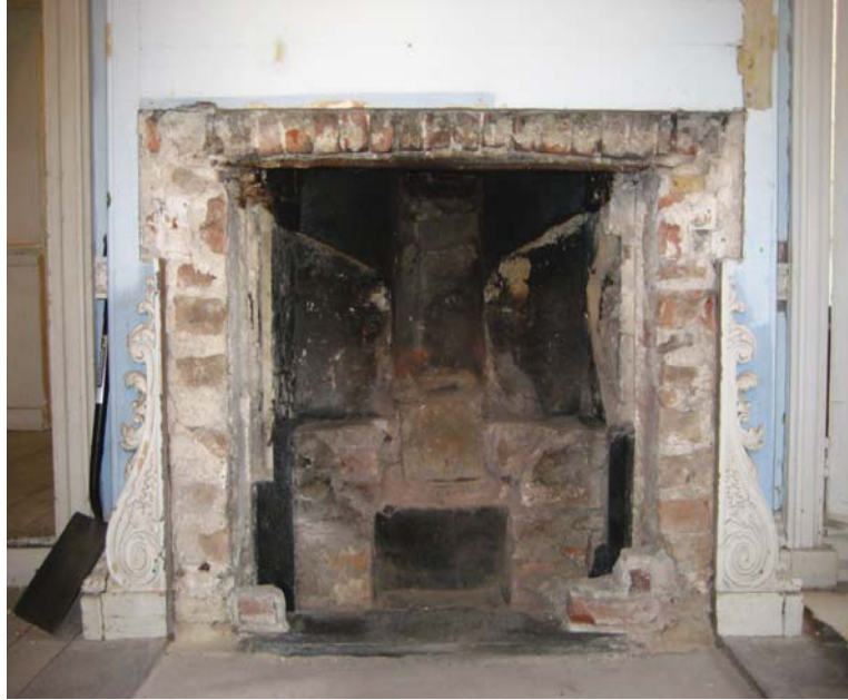
Figure I.43: View from the south of the fireplace following removal of a portion of the later infill, revealing the evidence of a previous (not original) fireplace insert. Source: University of Pennsylvania.
