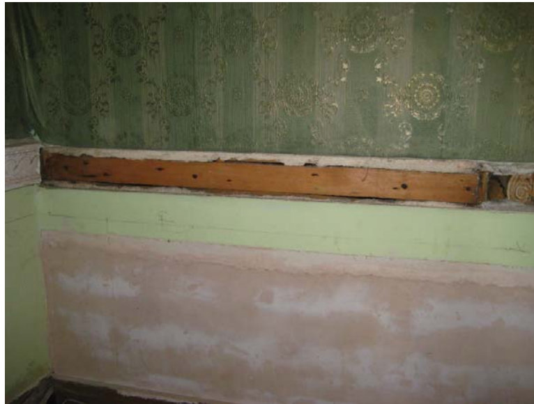
Figure II.3: View from the south of the west end of the north wall at its intersection with the west wall. Removal of the chair rail revealed that it was attached with hand-wrought nails to a furring strip that was in turn nailed to the studs with hand-wrought nails. The furring strip and chair rail were secured to the original wall framing before the plaster was installed. The furring strip terminates on the right at the western jamb of the balustraded opening. New chair rail was installed to the right when the balustraded opening was filled in in Phase III. Source: University of Pennsylvania.
