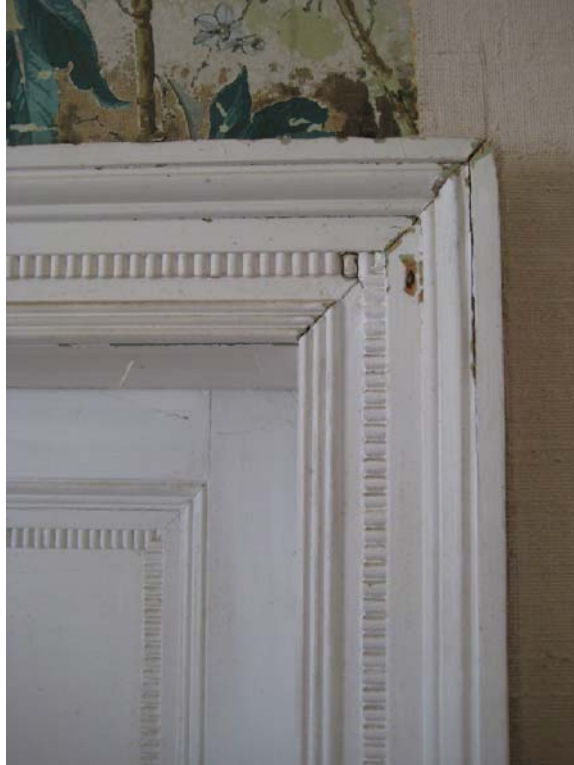
Figure III.10: View from the east of the top right corner of the door frame leading to the Outer Hall. The frame is attached to the furring strips behind it with hand-wrought nails, and is in its original Phase III position. Source: University of Pennsylvania.
