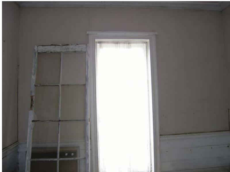
Figure 27: East Room: View looking south at the exterior door (secondary to the Outer Hall's main entrance). Source: University of Pennsylvania.
