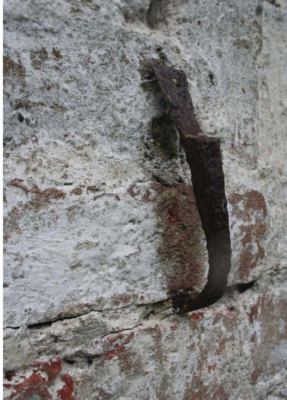
Figure II.9: Hand-wrought wall anchor. The ledger holding the rafters for the rear lean to sat on the flat portion at the top of the anchor and a nail was driven through the hole in the anchor into the wood. Source: University of Pennsylvania.
