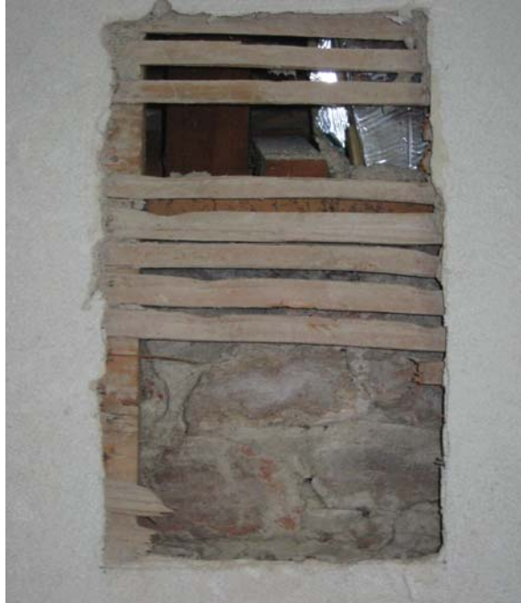
Figure II.13: View from the east showing the west wall of the Bathing Room. A section of lath and plaster was removed revealing that the original west wall terminated at a point approximately 6 ½ feet above the floor. The framing above the stone wall appears to date from the twentieth century, probably when the current hipped roof was installed over the Bathing Room. Source: University of Pennsylvania.
