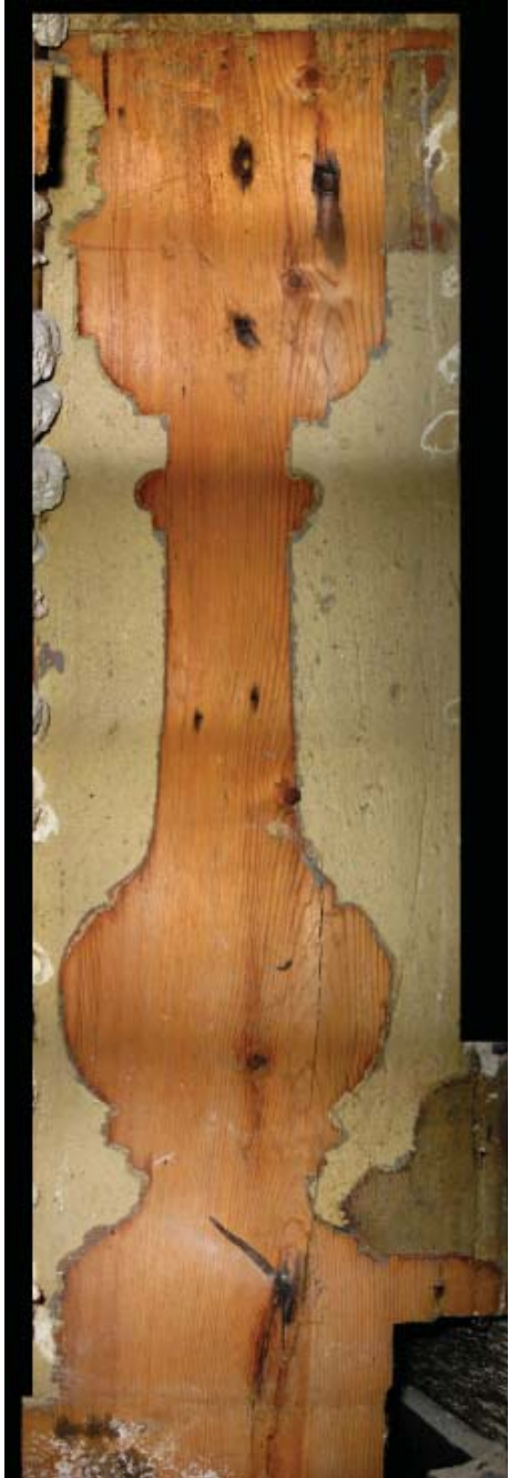
Figure I.27: View from the east of the baluster profile on the west jamb of the original balustraded opening. Source: University of Pennsylvania.
