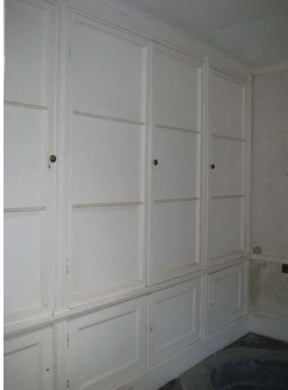
Figure V.6: View from the east of the cabinetry on the south wall of the Bathing Room. Source: University of Pennsylvania.
