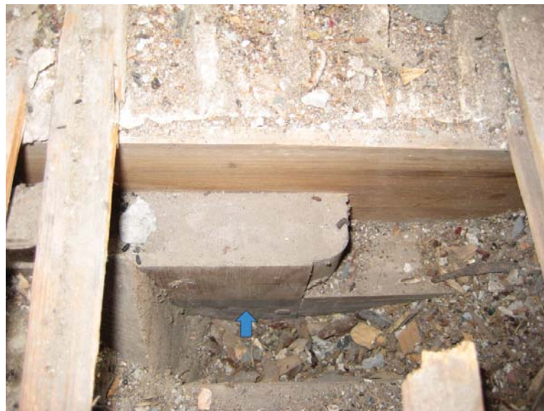
Figure I.36: View looking down from the attic space above the Inner Hall at the top of the paneled wall to the east of the fireplace mass. The paint line indicates the point of intersection of the original cornice moulding (now missing) and the paneling. Source: University of Pennsylvania.
