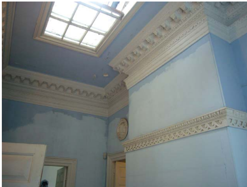
Figure 34: Inner Hall: View looking up at ceiling. Notice the window sash borrowing light from a skylight in the roof. Source: University of Pennsylvania.
