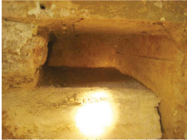
Figure I.10: View from the north of the original scored stucco extending into the reveal of the blind opening below the circular window to the Storage/Dressing Area. Source: University of Pennsylvania.
