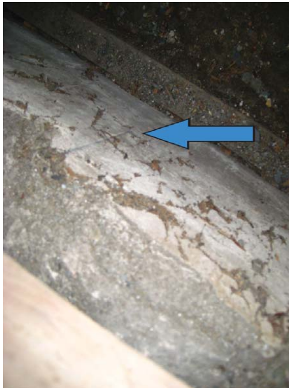
Figure II.1: View looking down at the top of the south (parapet) wall from the north side of the attic space above the West Room. The surviving scored stucco exterior finish is visible. Source: University of Pennsylvania.
