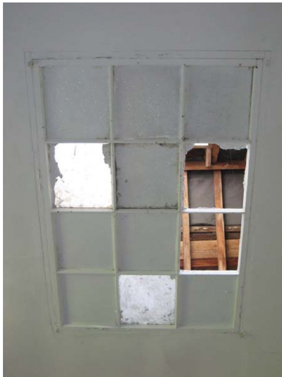
Figure V.3: View looking up at the glazed sash in the ceiling of the Bathing Room that borrows light from a skylight in the roof. The roof framing is visible through the missing window pane. Source: University of Pennsylvania.
