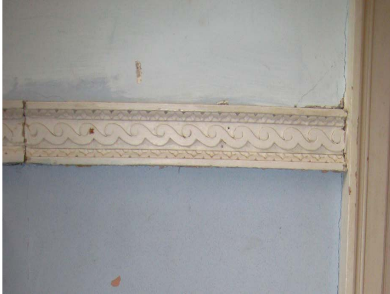
Figure III.5: View from the north of the south wall of the Inner Hall to the left (east) of the central doorway inserted in the in-filled balustraded opening. The chair rail and baseboard were pieced out to span the eastern in-filled section of the wall. Source: University of Pennsylvania.
