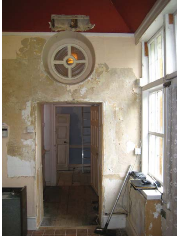
Figure V.2: View from the north (in the existing Kitchen) of the doorway leading to the current Corridor and former Privy. This doorway was widened, probably when the Kitchen was constructed. Source: University of Pennsylvania.
