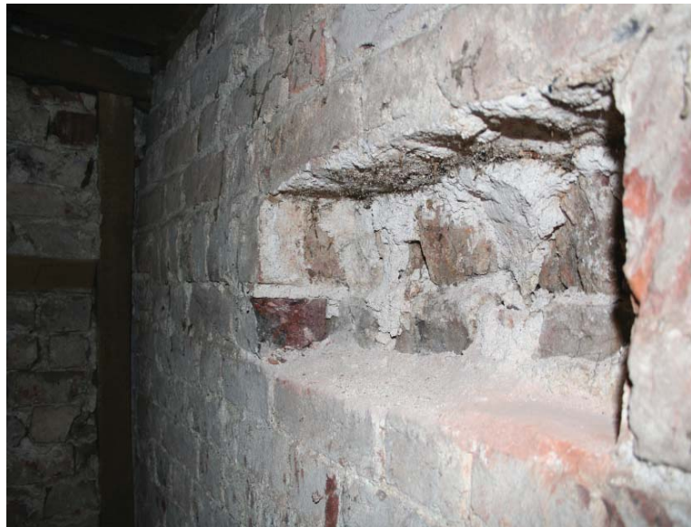
Figure II.3: Wall with portion of infill bricks removed. There are no obvious places where the removed bricks would have keyed into the wall, indicating that they were later infilled. Source: University of Pennsylvania.
