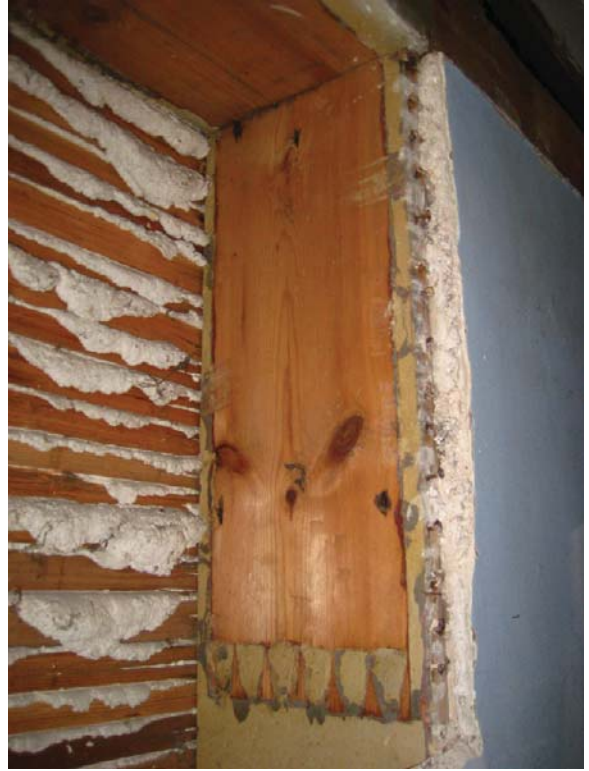
Figure I.28: View from the east of the paint evidence for the bracket at the top of the original balustraded opening. Source: University of Pennsylvania.
