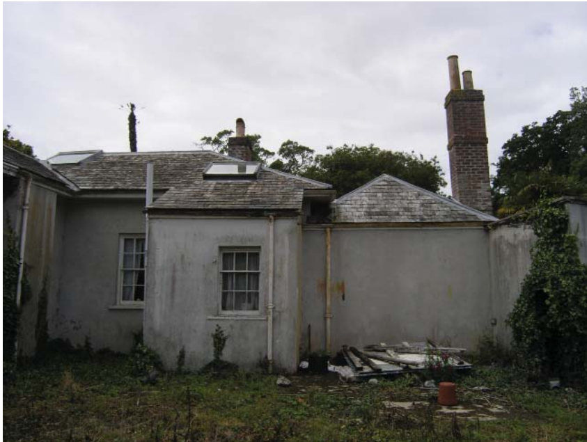
Figure 21: East Elevation: View showing series of intersecting slate hipped roofs from the east elevation. Source: University of Pennsylvania.
