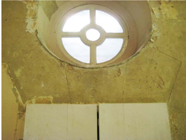
Figure I.8: View from the north of the original scored stucco below the circular window in the Storage/Dressing Room. Source: University of Pennsylvania.
