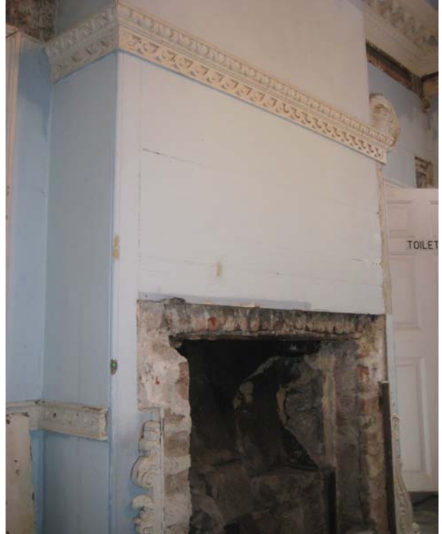
Figure I.40: View from the southwest of the original chimney breast sheathed with flush boards and trimmed with a carved egg and dart moulding. Source: University of Pennsylvania.
