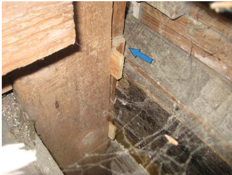
Figure I.15: View from the attic space above the center partition showing a fragment of original paneling in place (facing the Outer Hall) at the eastern end of the partition. Source: University of Pennsylvania.
