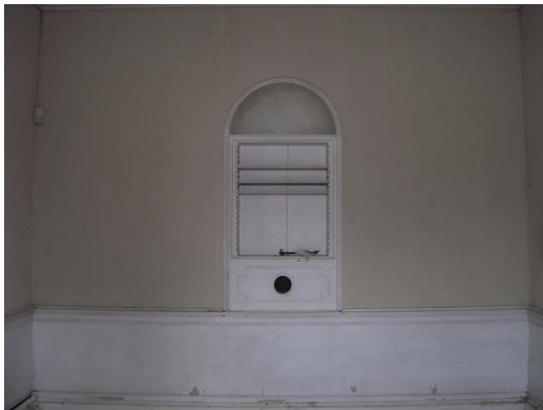
Figure 28: East Room: View looking north at built-in cabinet set above the wood wainscot. A circular brass ventilation device is built into the base of this cabinet. Source: University of Pennsylvania.
