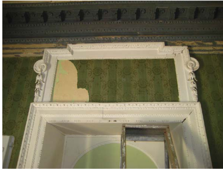
Figure III.3: View from the west at the top of the door frame leading to the East Room. The top piece of the carved frame was pieced to accommodate the wider doorway. The top piece of the overdoor was also pieced as shown in the previous image. Source: University of Pennsylvania.
