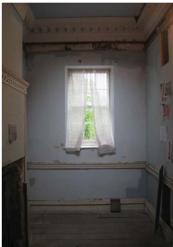
Fig. B16 Inner Hall - East Elevation: View looking East 2008 Summer Conservation Team
