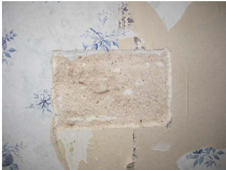
Figure I.11: View from the south of the original plaster on the north wall of the Storage/Dressing Area inside of the blind opening which did not extend through the wall. Source: University of Pennsylvania.
