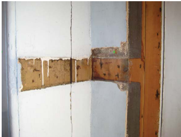
Figure I.38: View from the south east at the intersection of the east face of the chimney mass with the eastern paneled wall showing evidence of the earlier chair rail. Source: University of Pennsylvania.
