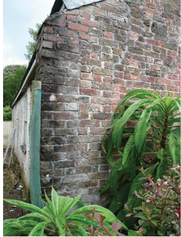
Figure I.2: West wall of French Garden House. Two butt joints are visible. The joint on the left shows where a buttress was added later in construction, and the joint on the right shows the intersection between the original wall and the west wall. Source: University of Pennsylvania.
