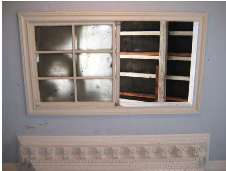
Figure V.8: View looking up at the glazed sash in the ceiling of the Inner Hall that borrows light from a skylight in the roof. Source: University of Pennsylvania.
