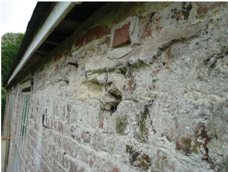
Figure II.8: Remains of mortar flashing and slate roof tiles in rear wall, visible just underneath the modern brick. Mortar was commonly used as flashing before lead became readily available. Source: University of Pennsylvania.
