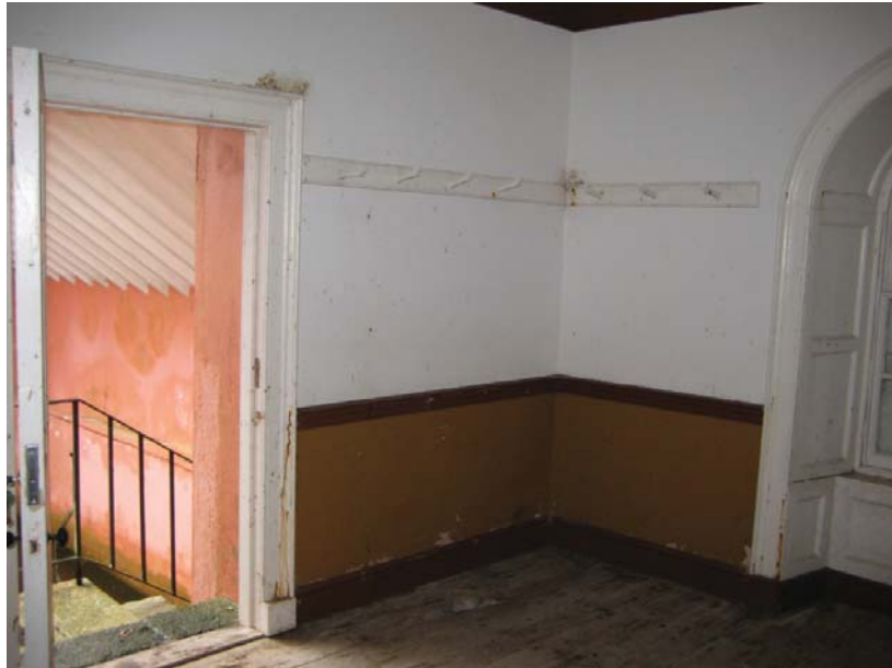
Figure 15: The Bath at Antony: View looking northeast at corner of warming room, adjacent to bathing room. Source: University of Pennsylvania.
