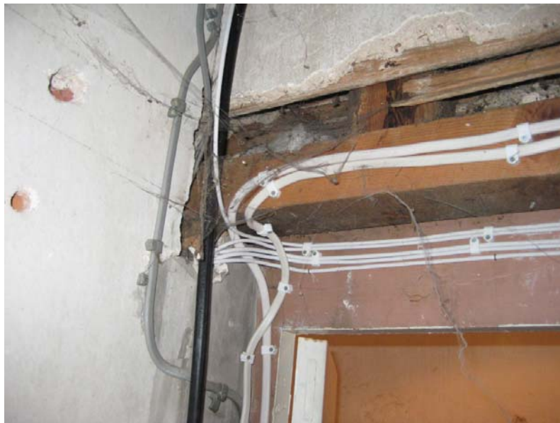
Figure I.48: View from the east (inside of the closet) of the surviving upper portion of the original east wall of the Privy. Source: University of Pennsylvania.
