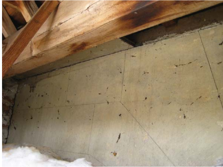
Figure I.2: View of the original west façade from the west (in the attic space above the Bathing Room ceiling). The original scored stucco exterior finish is largely intact; the radiating scoring lines at the left relate to the circular clerestory window, the top of which is still in place. Source: University of Pennsylvania.
