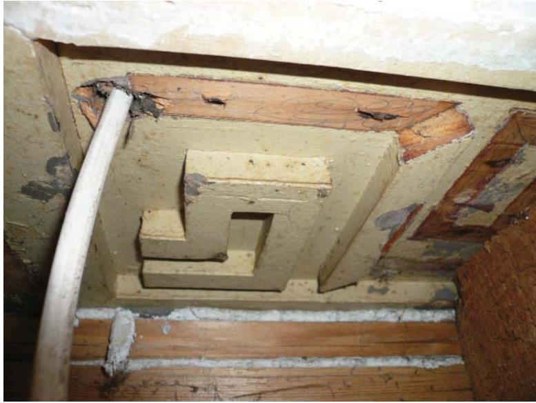
Figure 1.29: View looking up at the Greek key that has survived on the soffit of the original balustraded opening. Source: University of Pennsylvania.
