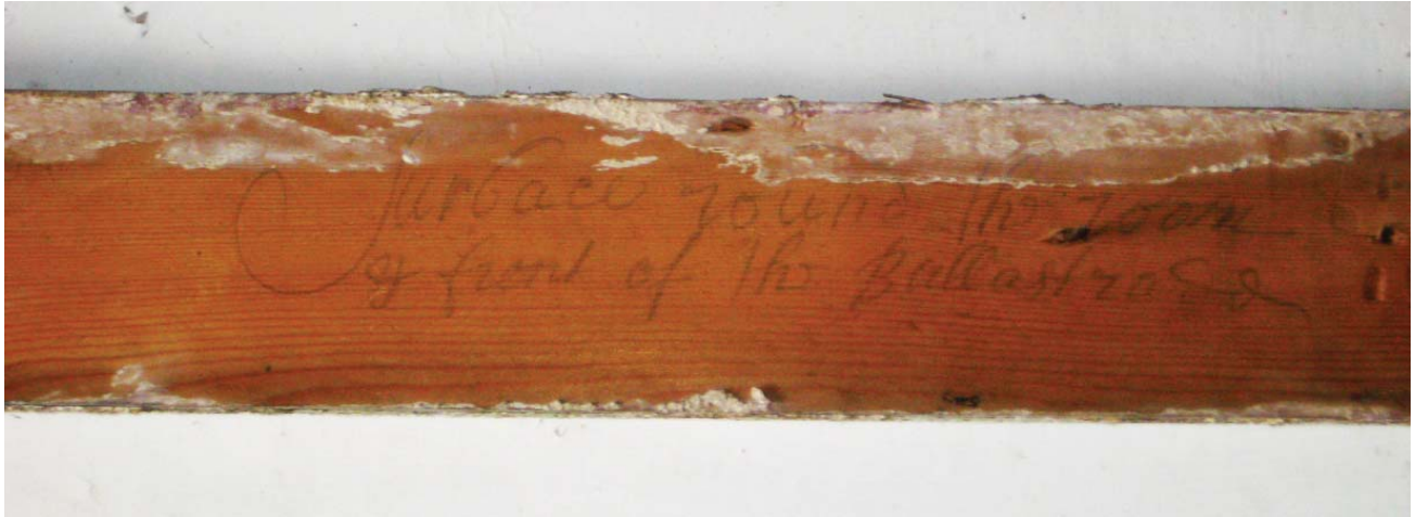
Figure II.4: The chair rail in the corresponding location on the eastern end of the north wall, to the east of the balustraded opening, was removed for investigation. This inscription in pencil was found on the back side of the chair rail, indicating that the balustrade was in place when the chair rail was installed. The nails and nail holes relating to this installation indicated that it is in its original position. Source: University of Pennsylvania.
