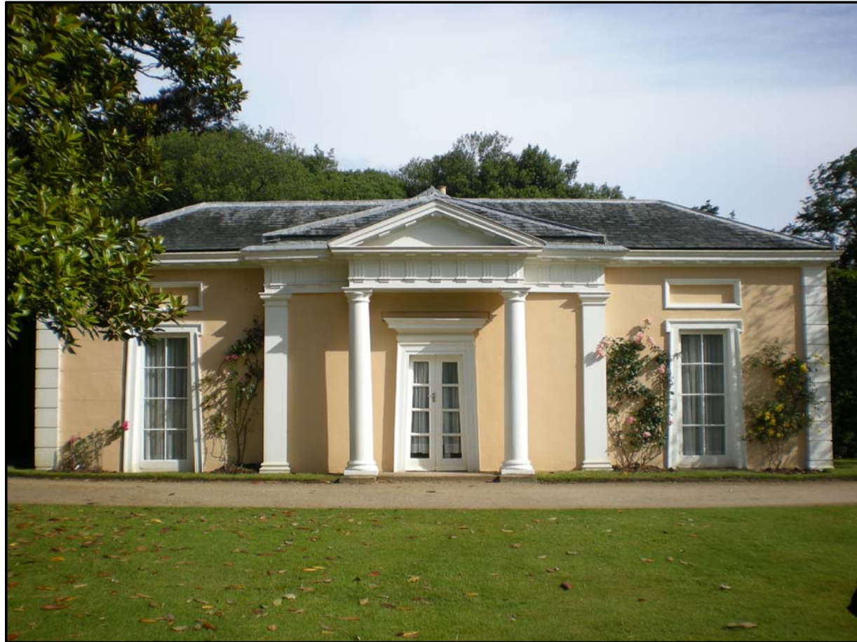
South Elevation (front) of the English Garden House at Mount Edgcumbe Summer 2008
