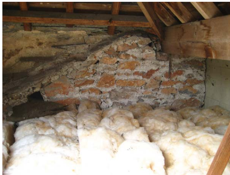
Figure II.14: View from the south in the attic space above the ceiling of the Bathing Room. The evidence of the original sloping roof over the Bathing Room is apparent. The parapet wall above the sloping roof is covered in stucco, and fragments of what appears to be slate cap flashing project from the wall. No evidence of interior finish exists on the north parapet wall below the roof slope. Source: University of Pennsylvania.
