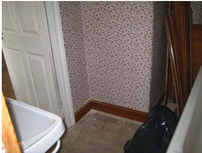
Figure 37: Modern Bathroom: View looking southwest at wall jogging inwards due to the Inner Hall's fireplace. The sink is in the lower left corner and the bathtub is in the lower right corner. Source: University of Pennsylvania.
