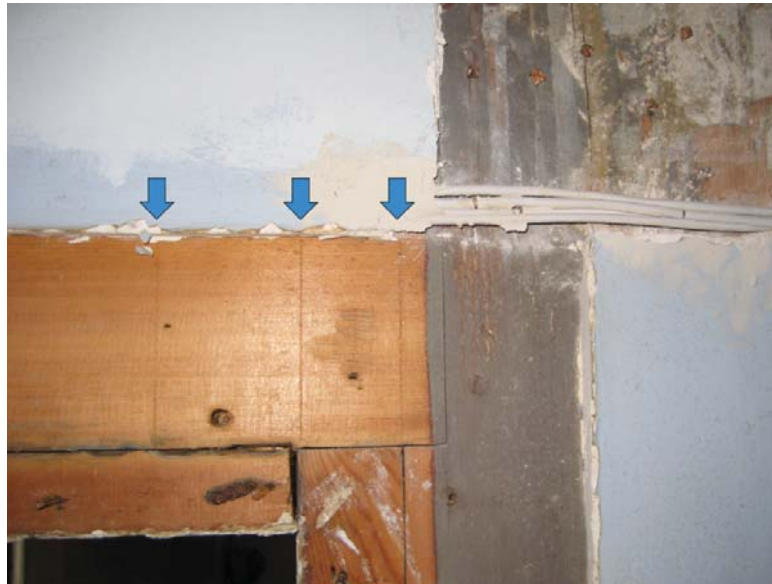
Figure I.35: View from the south of a portion of the western doorway into the Privy (following removal of the current door surround) showing evidence of the Phase I door opening and frame. Source: University of Pennsylvania.
