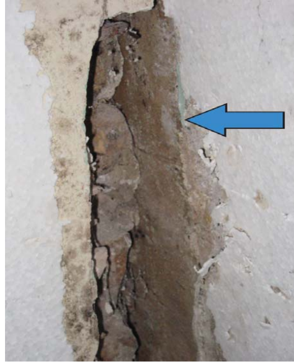
Figure I.5: View from the northwest (inside of the bottom cabinet on the south wall) of the butt joint between the south wall of the Bathing room (at the right) and the west façade of the original building (at the left). A portion of the original scored stucco exterior finish on the west façade has survived in this joint. Source: University of Pennsylvania.
