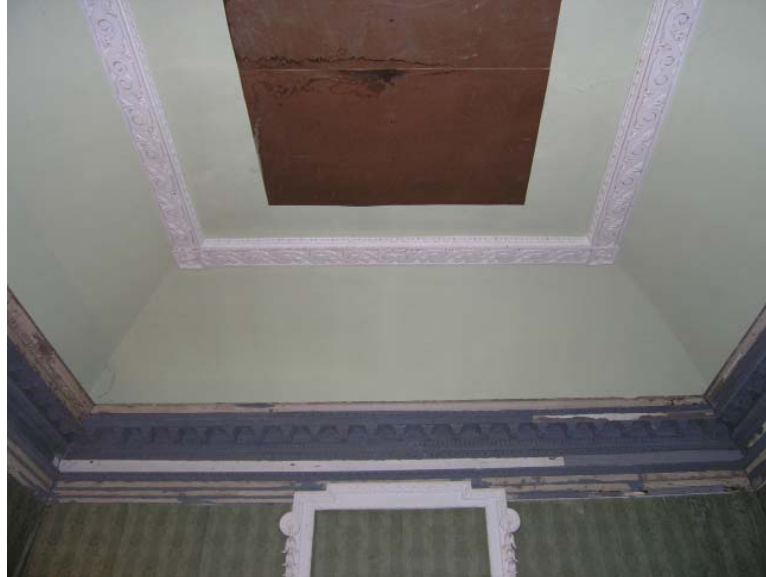
Figure II.5: View from the west looking east and up at the cornice, plaster cove ceiling and carved ceiling frame. The brown fiberboard panel at the center of the carved frame was installed following removal of a circular glass glazed sash that borrowed light from a skylight in the roof. This feature was not original, although its position in the building's chronology has not yet been determined. The carved frame is addressed in the Phase I discussions, and may have been relocated from an earlier flat ceiling the Outer Hall. Source: University of Pennsylvania.
