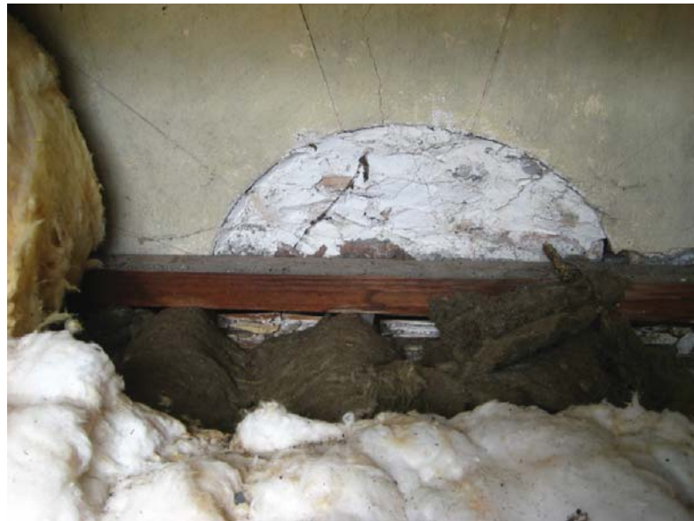
Figure I.26: View from the west of the top portion of the original circular clerestory window in the west façade. Source: University of Pennsylvania.
