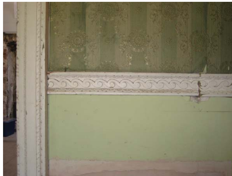
Figure III.4: View from the south at the chair rail to the east of the central doorway leading to the inner hall. The seam in the chair rail coincides with the eastern jamb of the original balustraded opening that was filled in as part of the Phase III renovations. The piece of chair rail to the left (west) of the seam was installed to span the eastern in-filled section of wall. Source: University of Pennsylvania.
