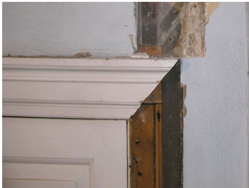
Figure I.34: View from the south of a portion of the eastern doorway into the Storage/Dressing Area (following removal of the current door surround) showing evidence of the Phase I door opening and frame. Source: University of Pennsylvania.
