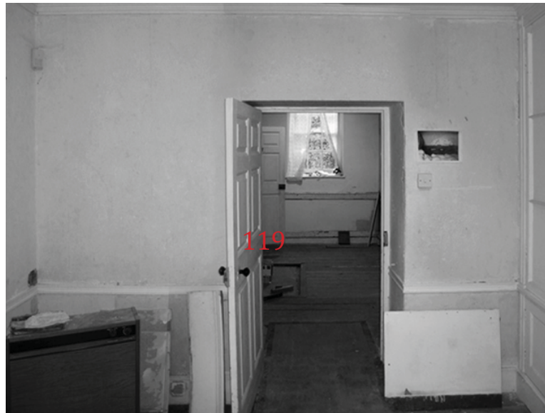
Bathing Room - East Wall
