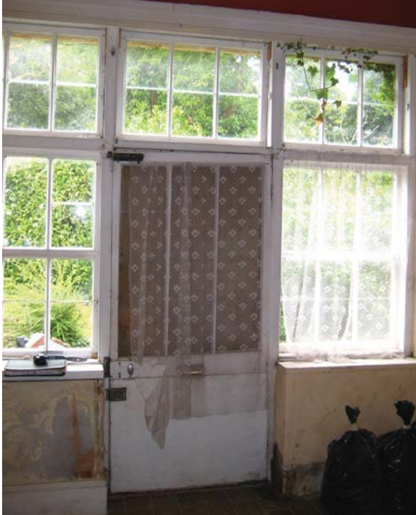
Figure 47: Kitchen: View looking at the west wall and the windows surrounding the door. Source: University of Pennsylvania.
