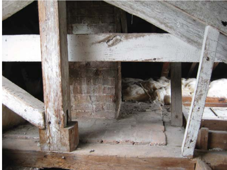
Figure I.25: View from the south in the attic above the Inner Hall. The framing is original and was fabricated and installed to accommodate the brick chimney mass. Source: University of Pennsylvania.
