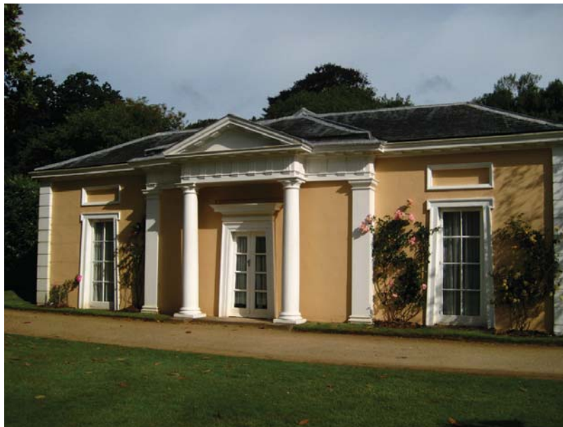
Figure 19: South Elevation: View depicting one-story building with exterior masonry walls, rendered in stucco. Source: University of Pennsylvania.
