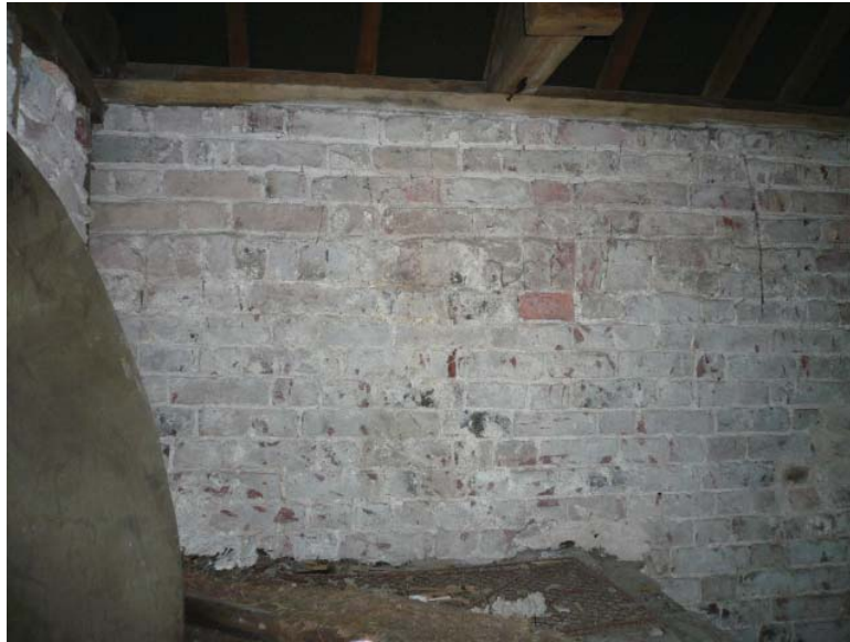
Figure II.4: The clean Flemish brick work is clearly visible above the infill layer. The bottom course of the infill contains the broken faced brick. To the right of this brick, the infill portion contains three courses and to the left only two. Source: University of Pennsylvania.
