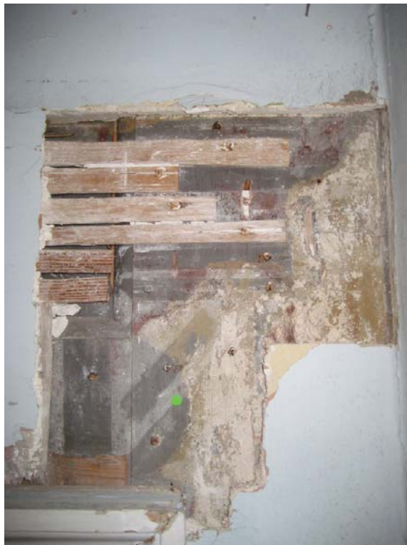
Figure I.32: View from the south of the original paneling that had been concealed by later decorative applications. Source: University of Pennsylvania.
