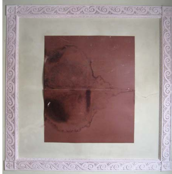
Figure I.22: View looking up at the square frame in the coved ceiling. The carving in this frame is quite similar to the other Phase I carving on the original east and west window frames in the Outer Hall and the fireplace consoles in the Inner Hall. Source: University of Pennsylvania
