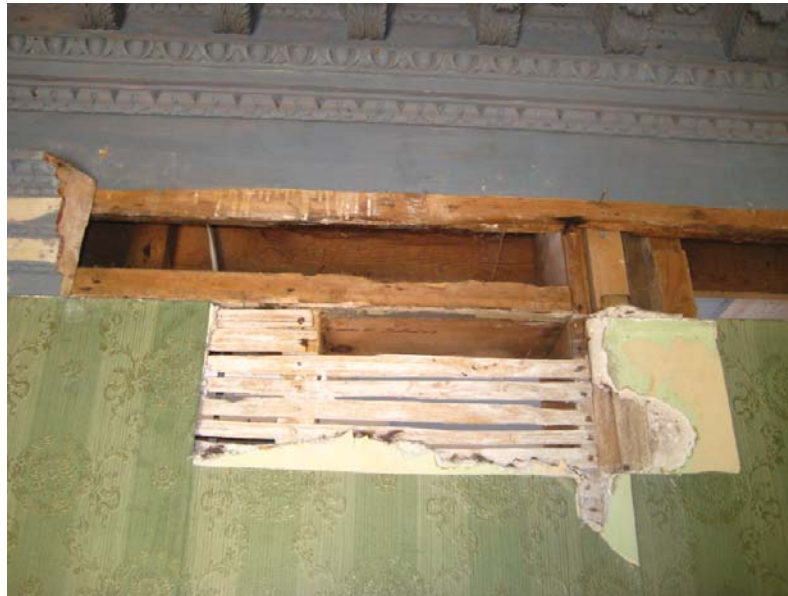
Figure I.16: View from the south of the unpainted south edge of the original soffit board spanning across the balustraded opening. The architrave of the cornice was originally nailed directly to the soffit board. Source: University of Pennsylvania.
